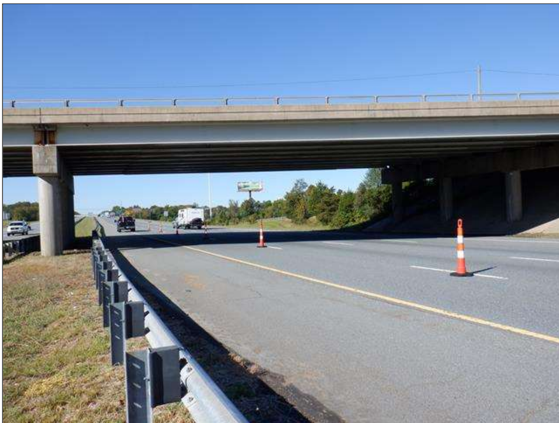
SPAN 2 VERTICAL CLEARANCE, LOOKING SOUTH
