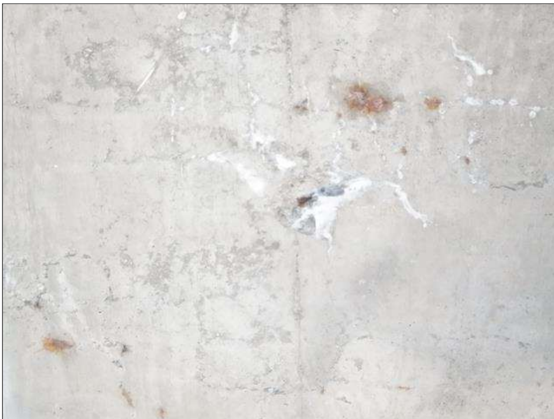
Span 3 Deck: PAR: 10 INCH DIAMETER X 1 INCH DEEP SPALL WITH EXPOSED REBAR, 5 PERCENT SECTION LOSS, IN UNDERSIDE BAY 3 AT 3 FEET PAST CENTER DIAPHRAGM, NO SECTION LOSS
