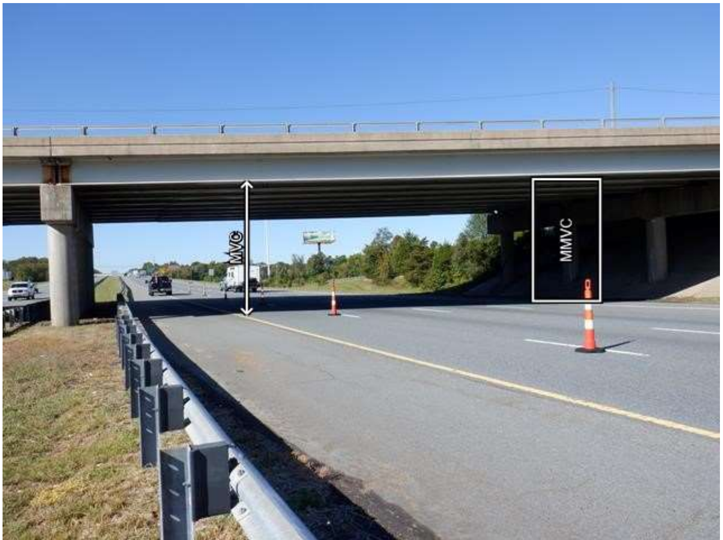
SPAN 2 VERTICAL CLEARANCE, LOOKING SOUTH - REQUEST LIDAR
