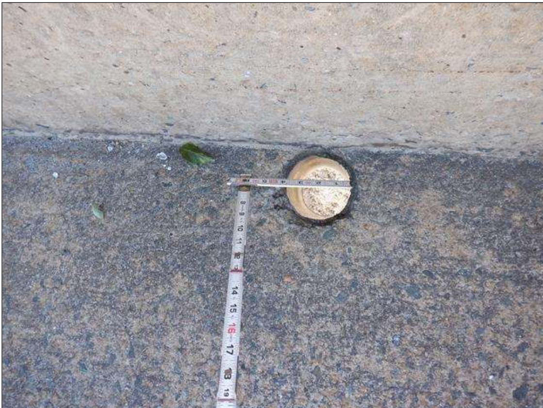
ALONG LEFT BRIDGE RAIL, 4 INCH DIAMETER SCUPPER
