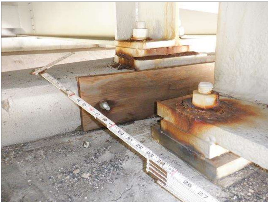
BENT 1 BEAM 5 BEARINGS
