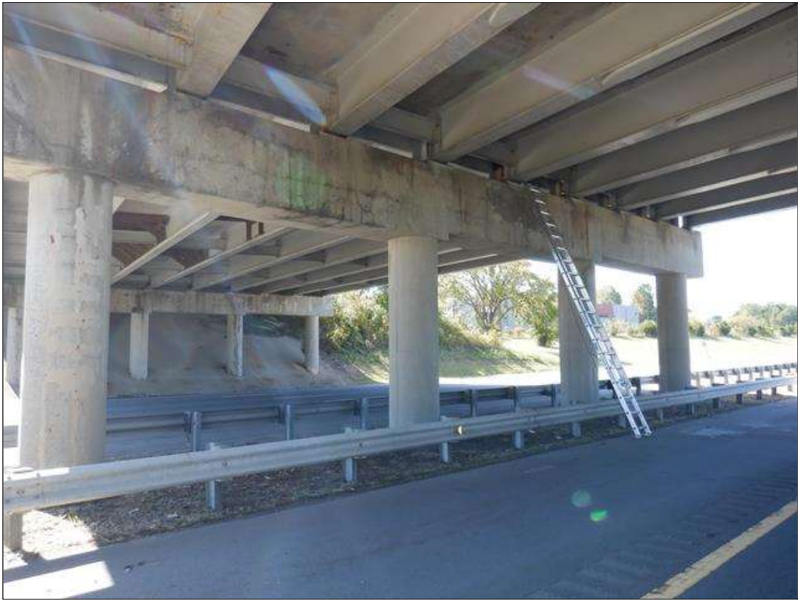
BENT 2 LOOKING EAST
