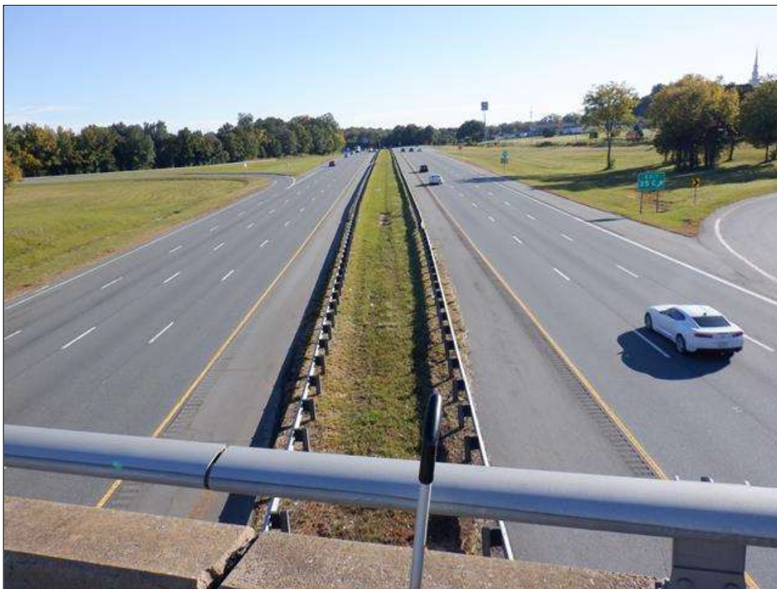
LOOKING NORTH FROM BRIDGE
