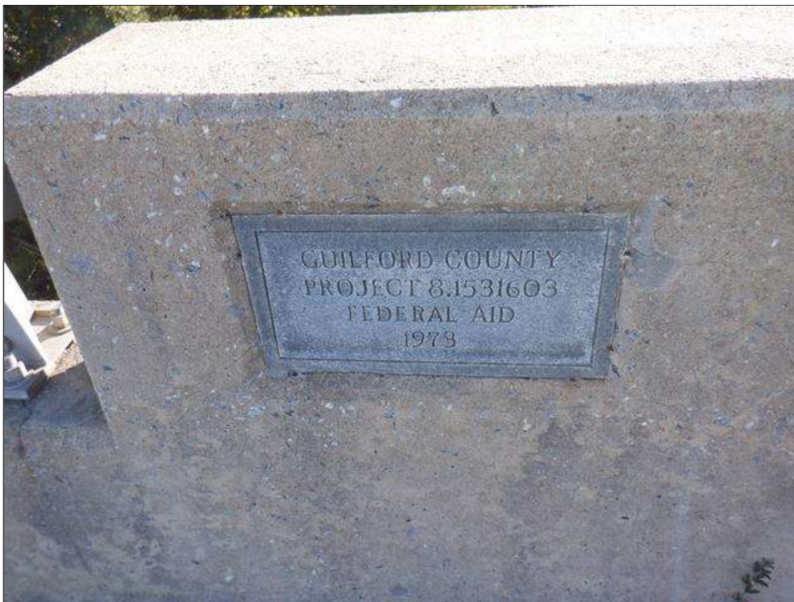
NORTHEAST BRIDGE PLAQUE
