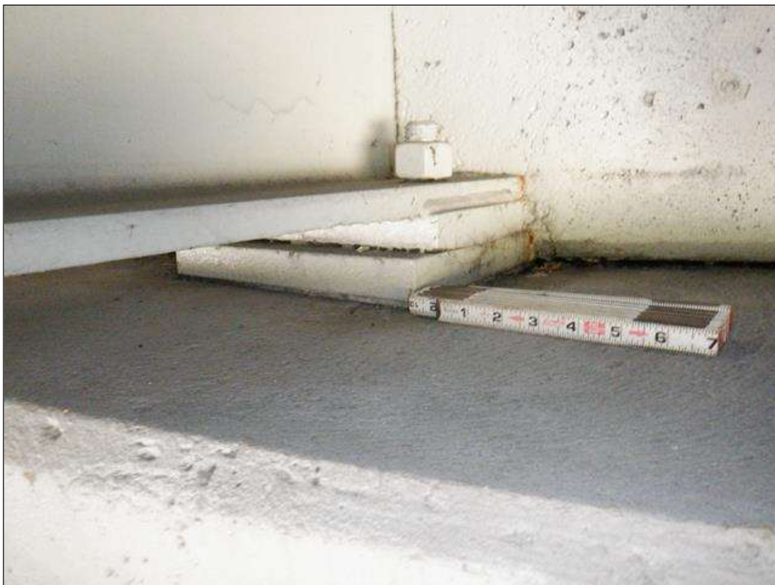
SPAN 4 BEAM 6 FAR BEARING
