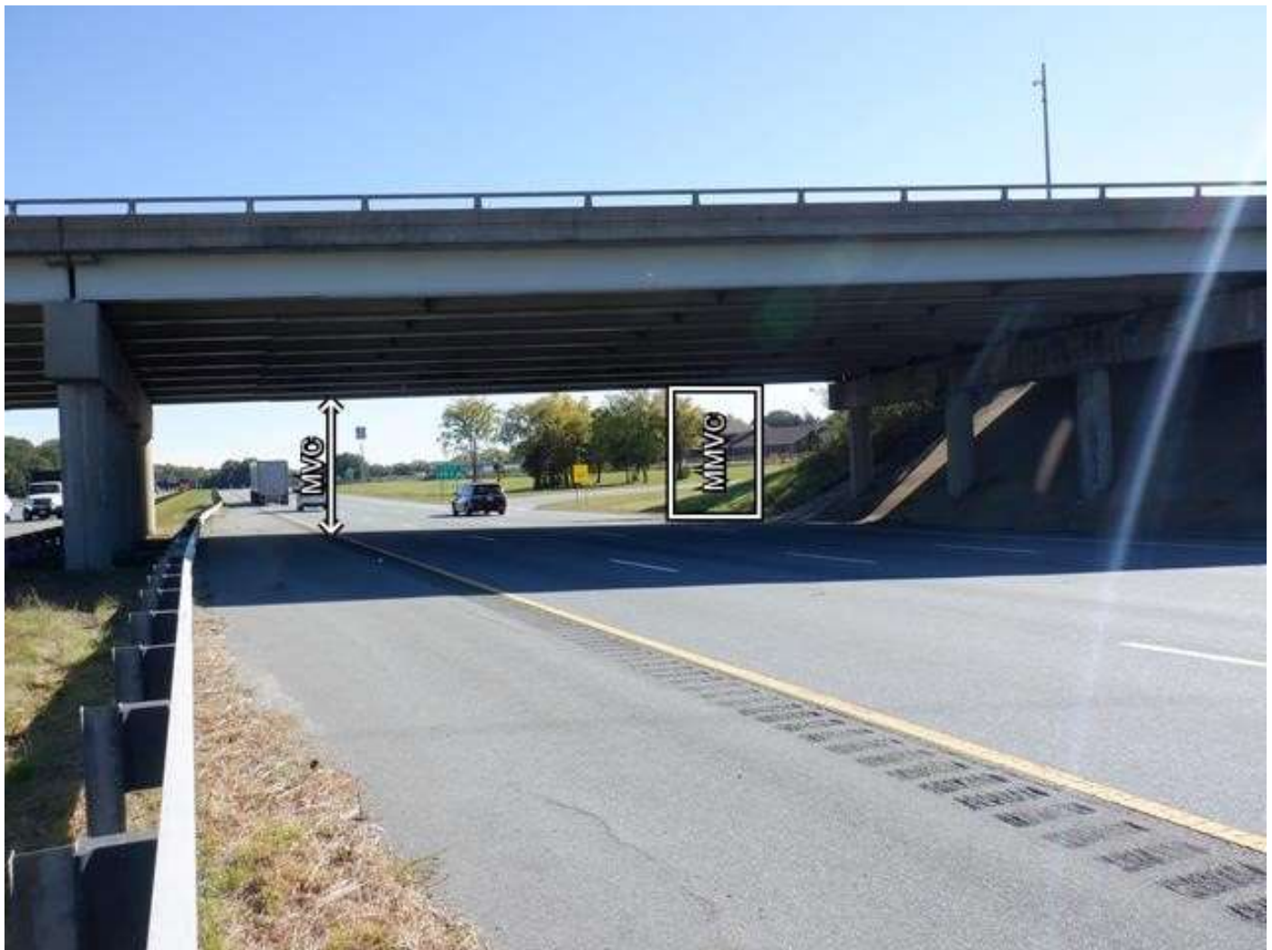
SPAN 3 VERTICAL CLEARANCE, LOOKING NORTH - REQUEST LIDAR
