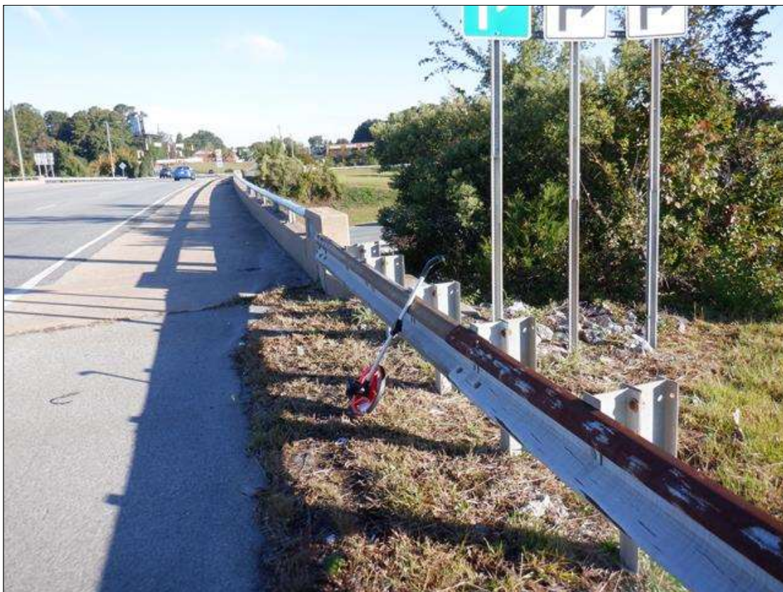
NORTHEAST GUARDRAIL TRANSITION
