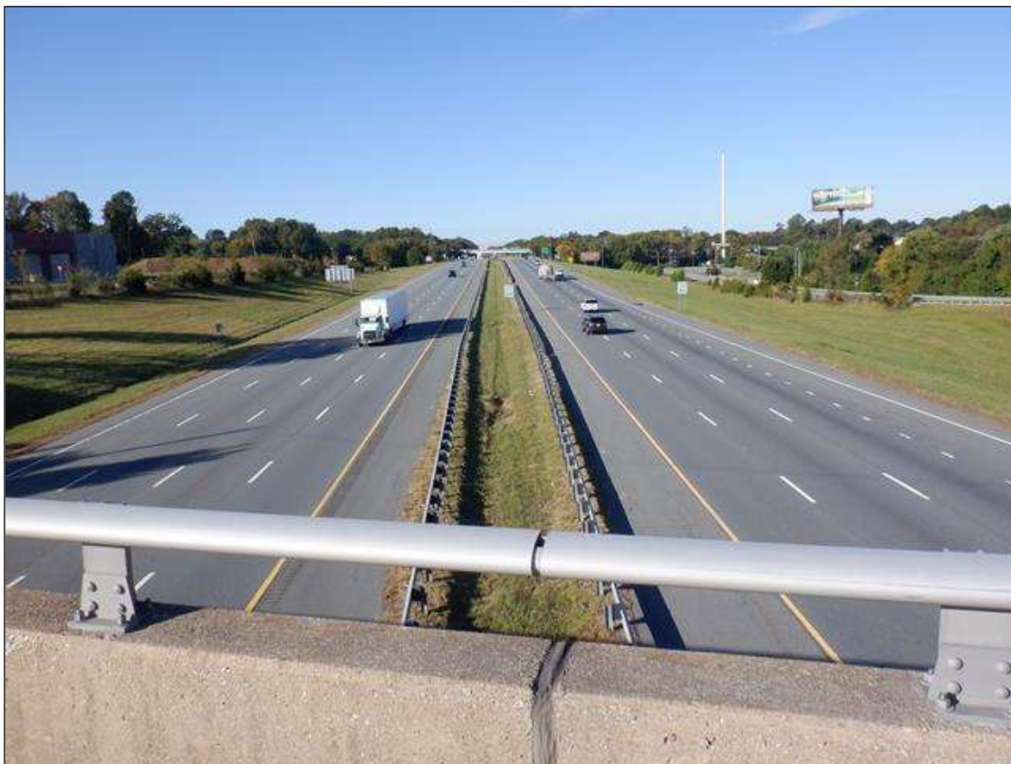
LOOKING SOUTH FROM BRIDGE
