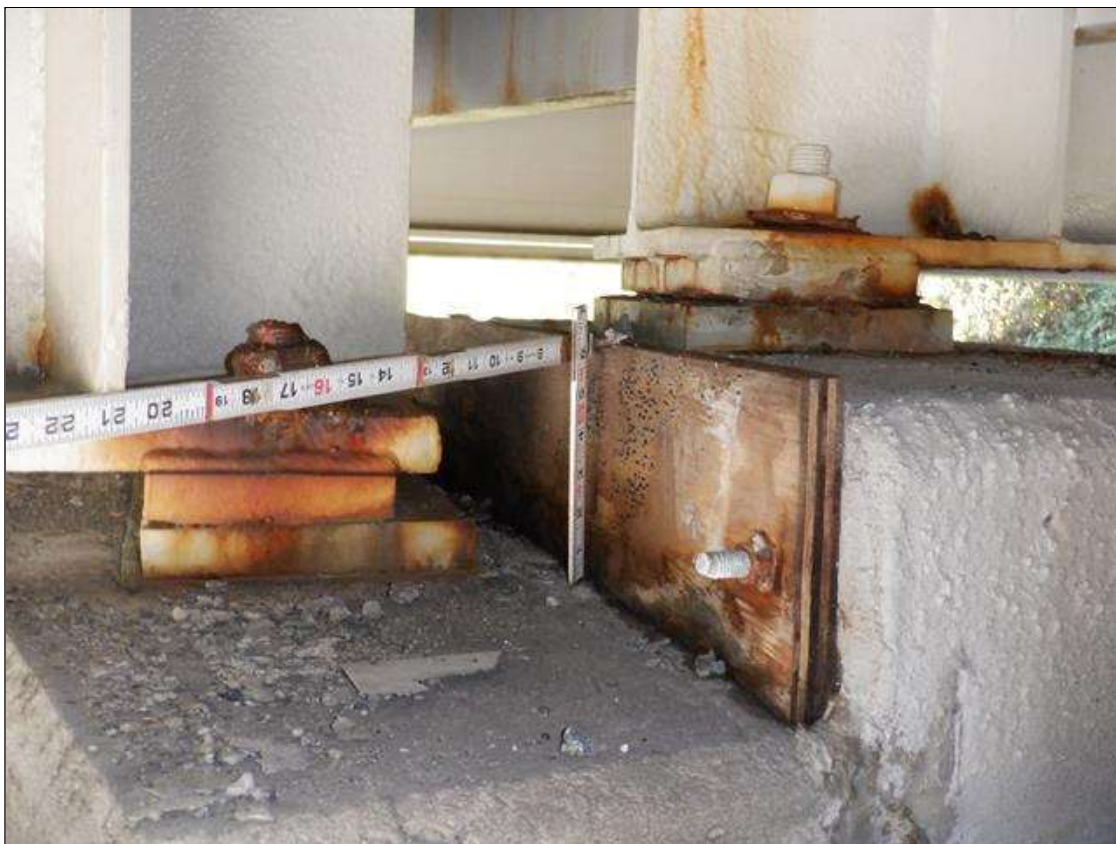
Bent 1 Cap 1: PATCHED PREVIOUS PRIORITY MAINTENANCE UNDER GIRDER 6 SPAN 1
