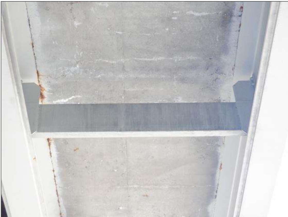
SPAN 3 BAY 1 INTERMEDIATE DIAPHRAGM
