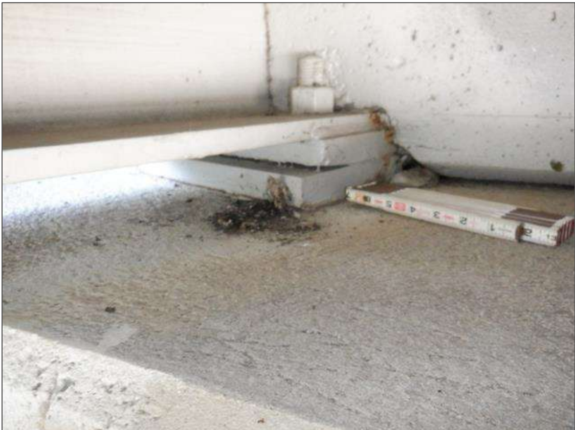
SPAN 1 BEAM 9 NEAR BEARING
