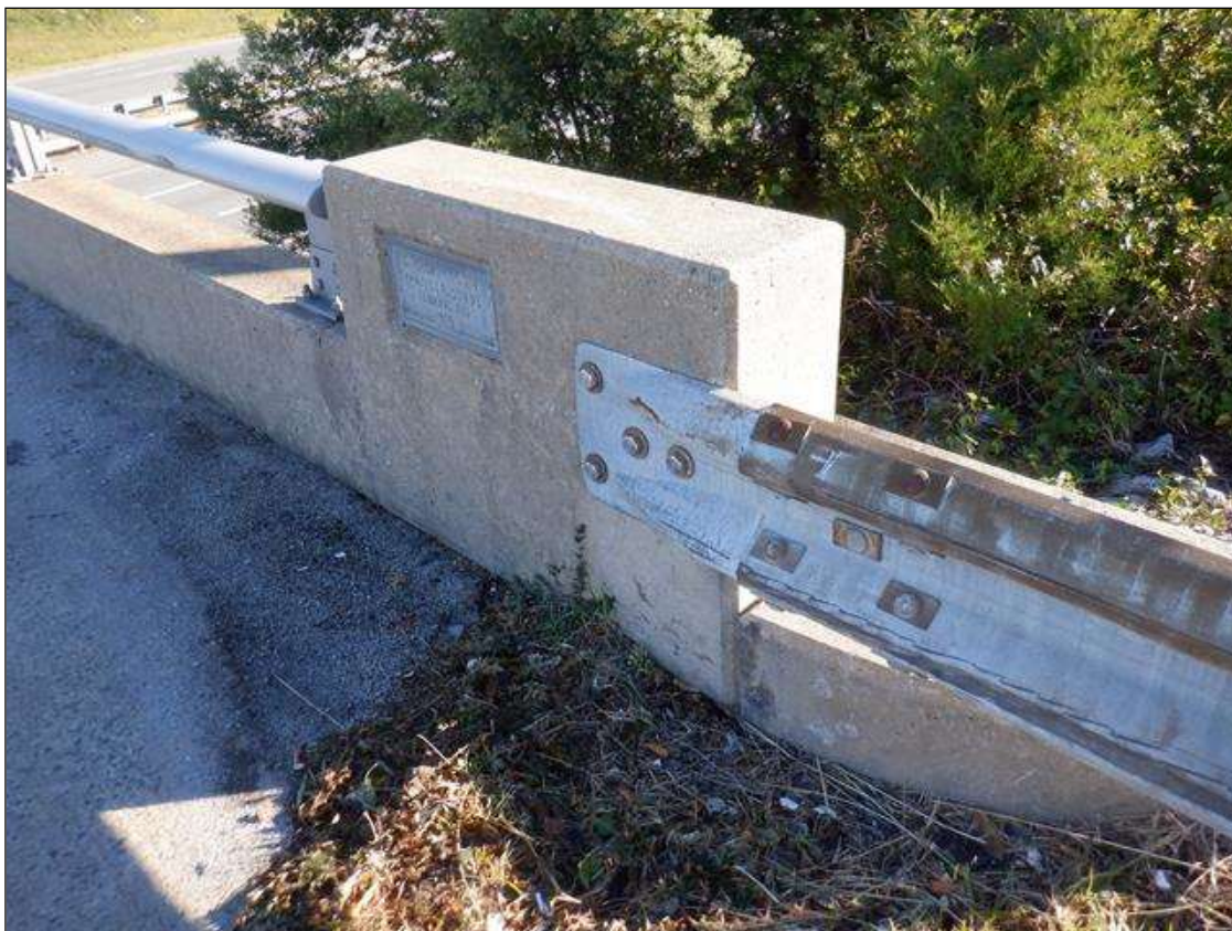
NORTHEAST GUARDRAIL ATTACHMENT
