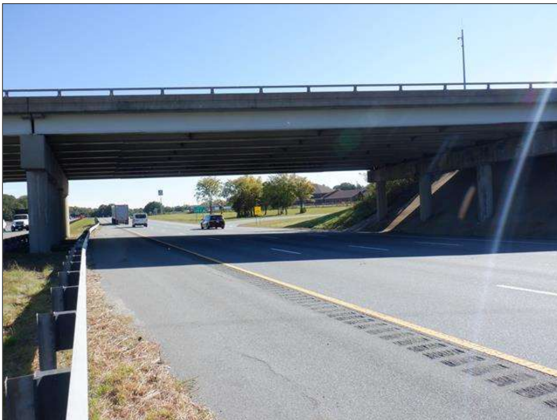
SPAN 3 VERTICAL CLEARANCE, LOOKING NORTH
