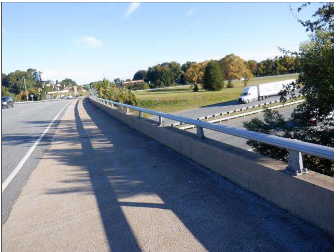
LEFT BRIDGE RAIL
