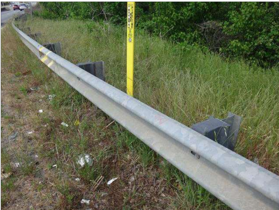
Southeast guardrail continuous
