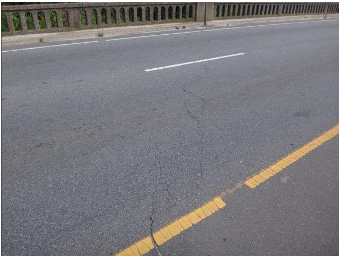
asphalt over bent 2
