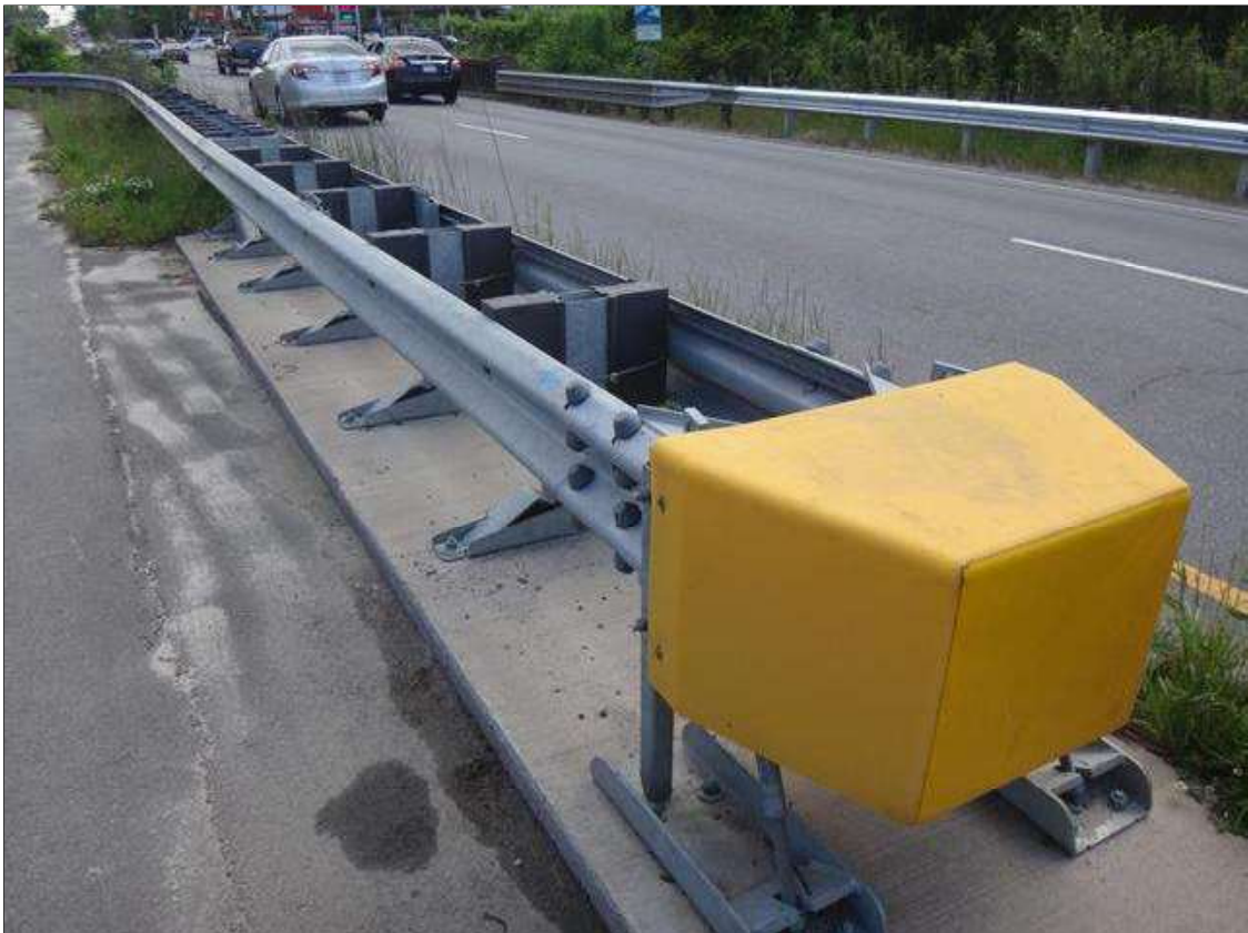
Northwest guardrail end treatment
