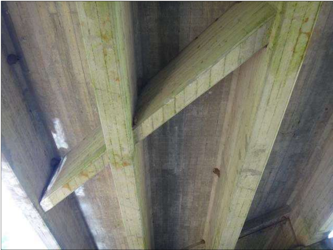
typical underside of deck
