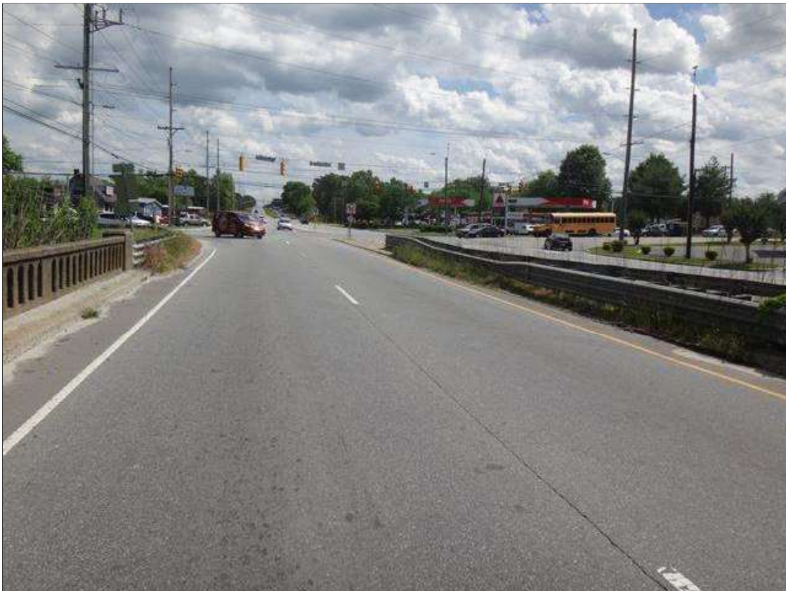
south approach roadway
