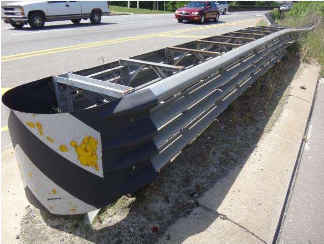
Southwest guardrail end treatment
