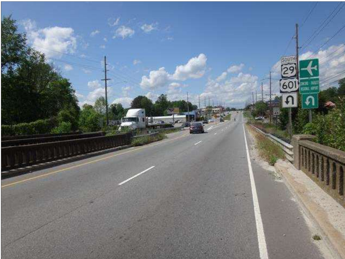
north approach roadway
