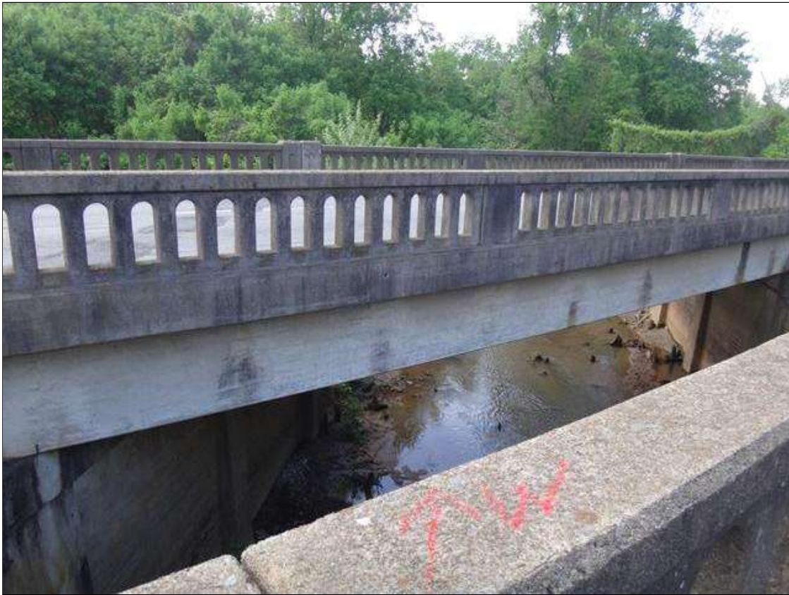
looking upstream west from bridge
