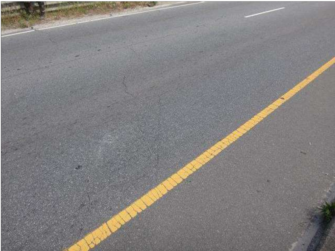
asphalt over end bent 2
