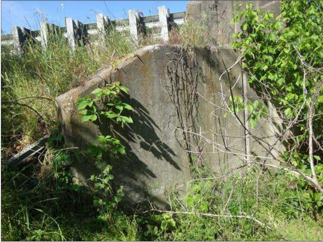
Southeast wingwall, typical all wingwall
