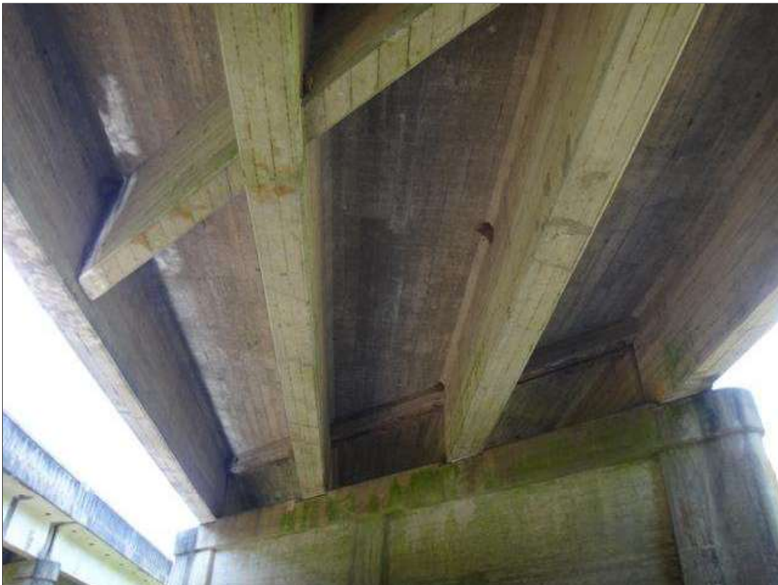
typical superstructure framing
