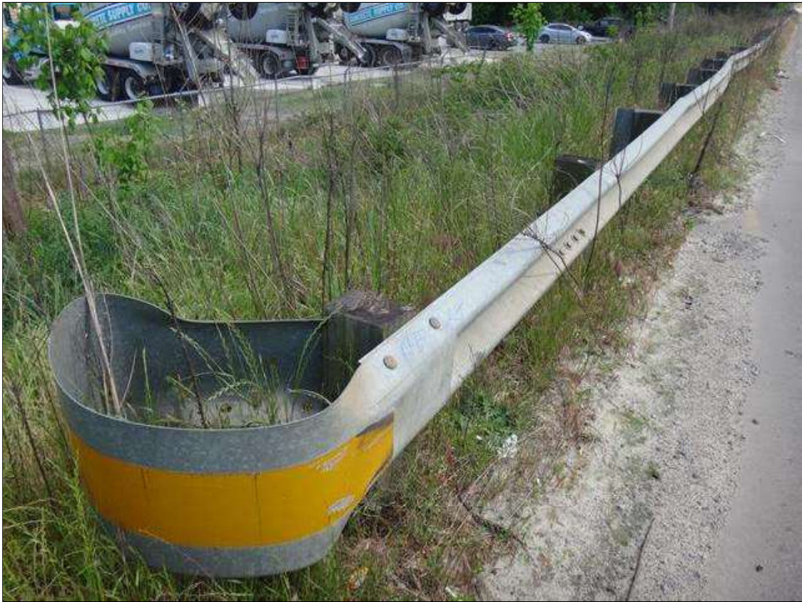
Northeast guardrail end treatment
