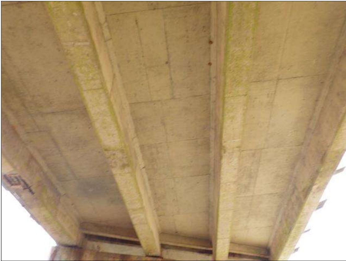
underside of deck (span 2)
