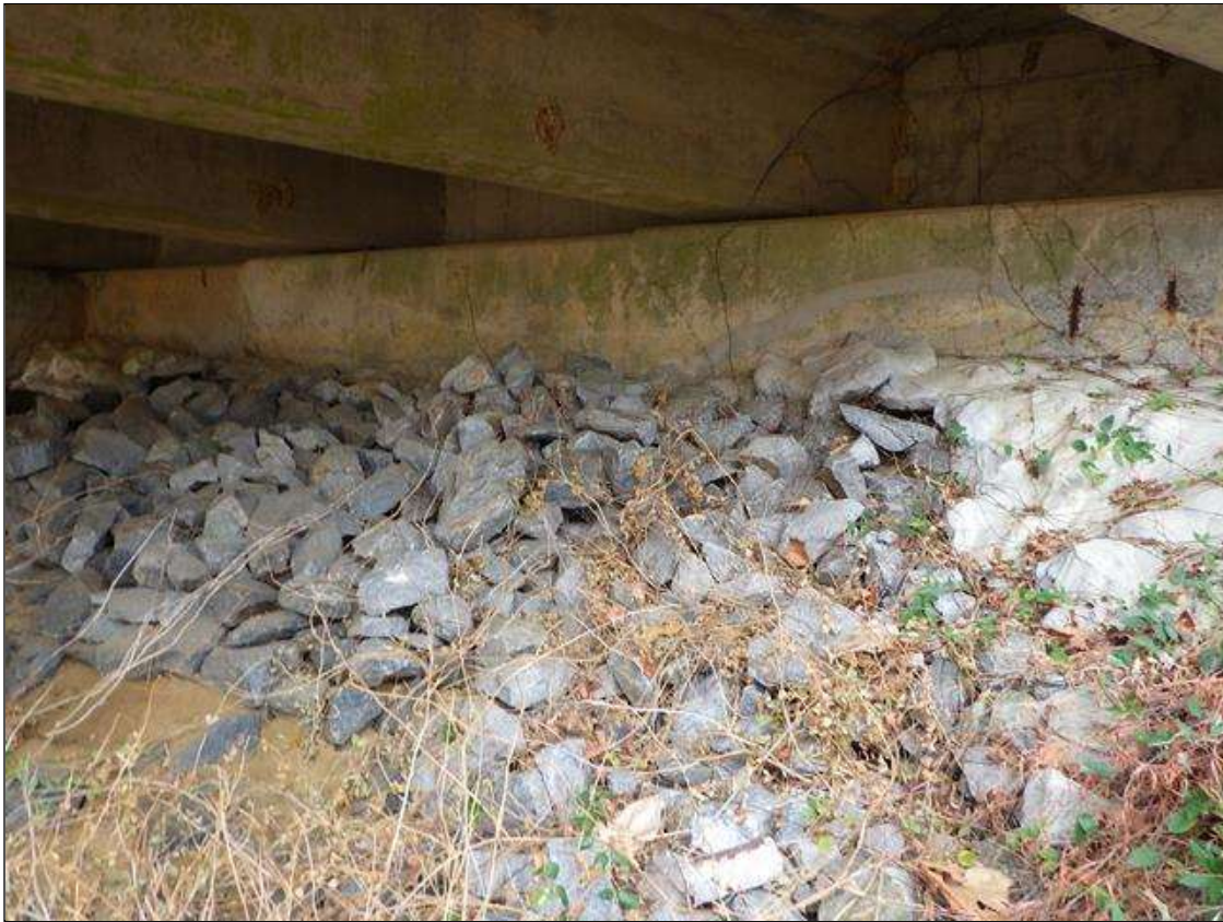
end bent 1 and slope protection
