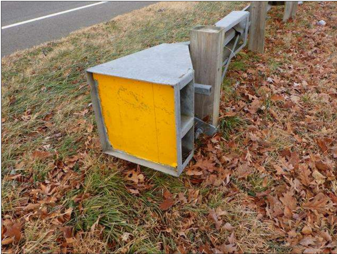
southeast guardrail termination
