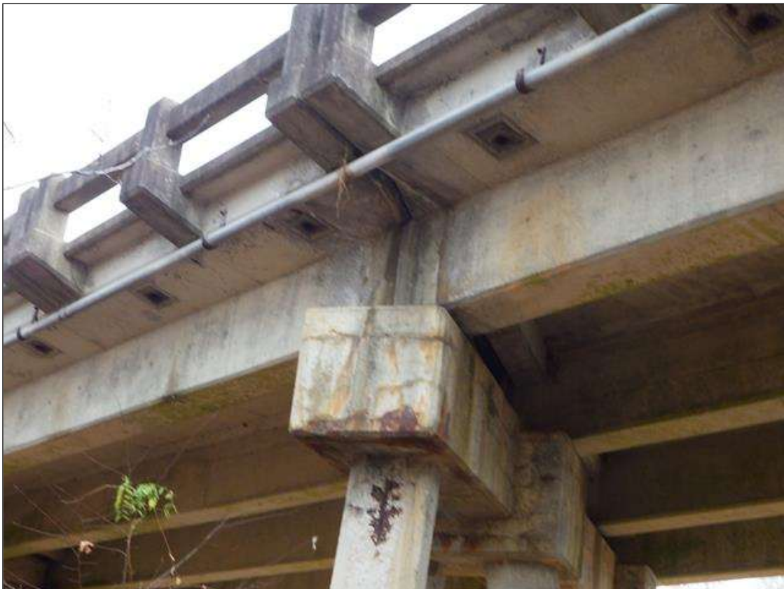
beams over bent 4
