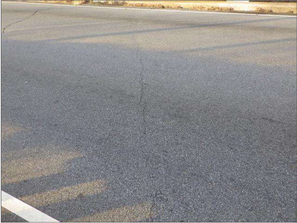
asphalt wearing surface over end bent 1
