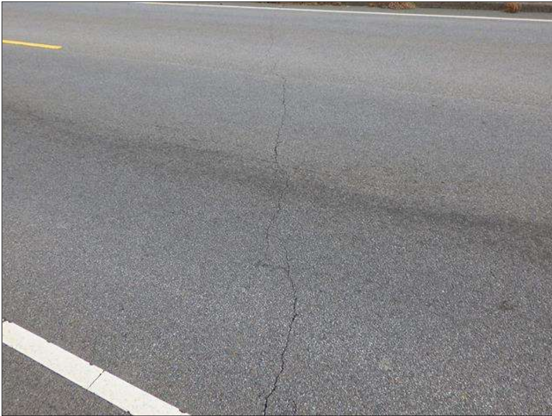
asphalt wearing surface over bent 2
