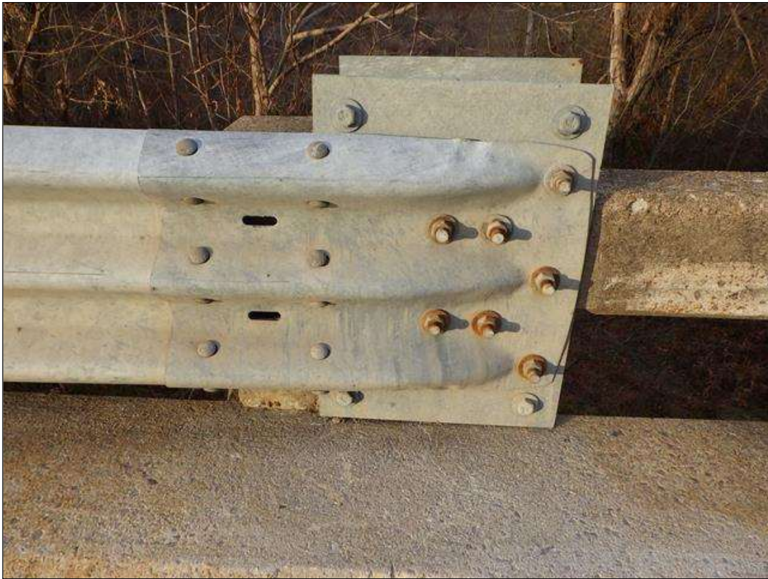
southwest guardrail attachment
