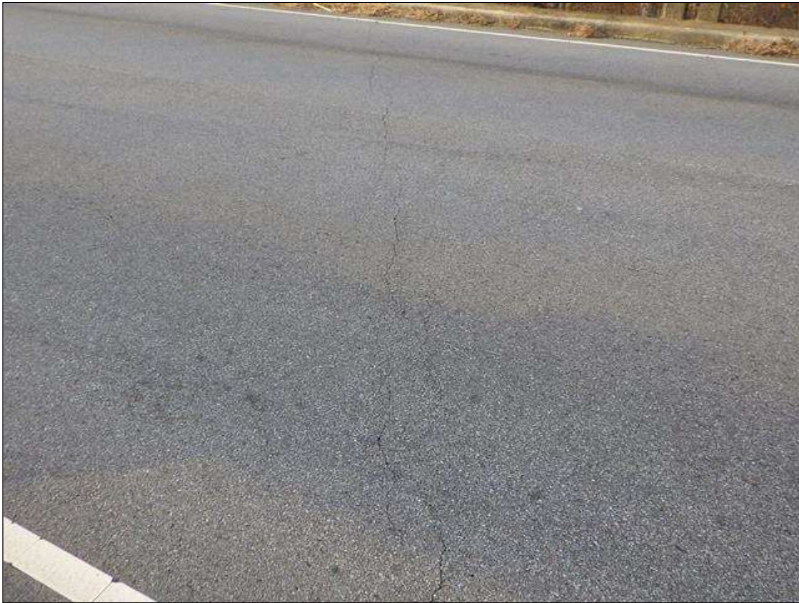
asphalt wearing surface over bent 4
