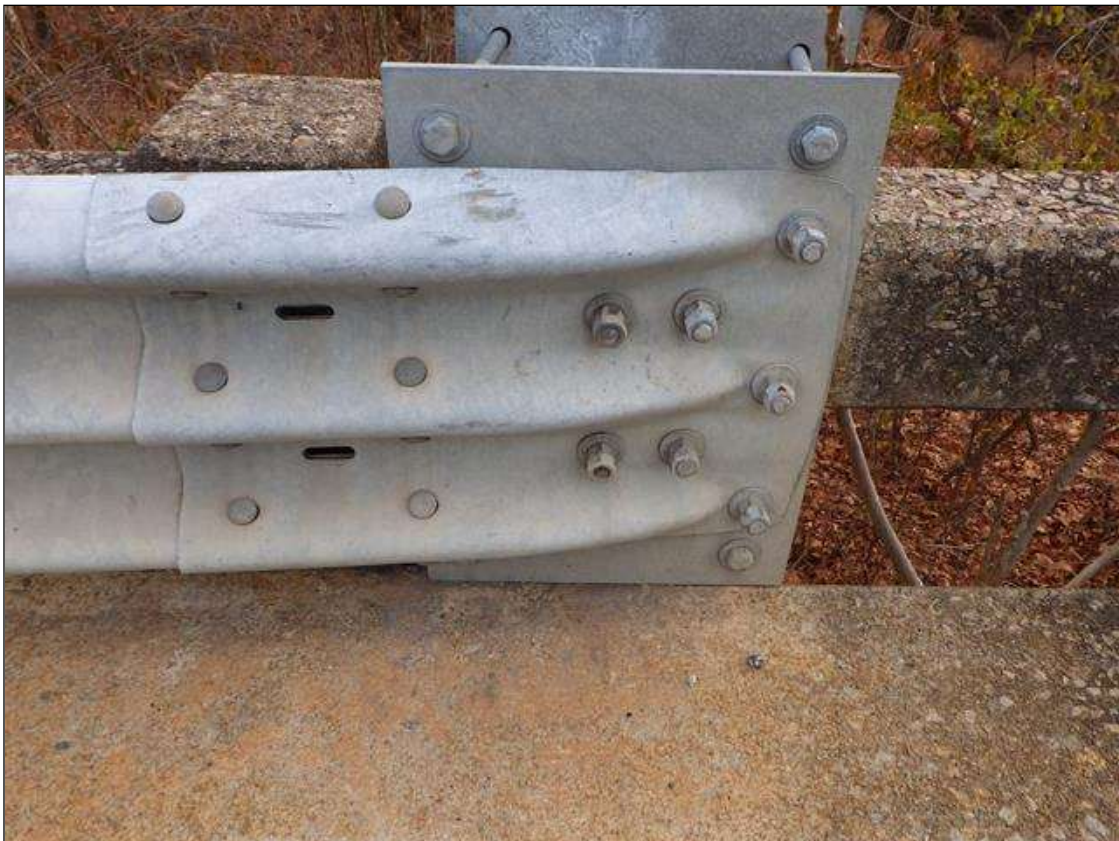
northeast guardrail attachment
