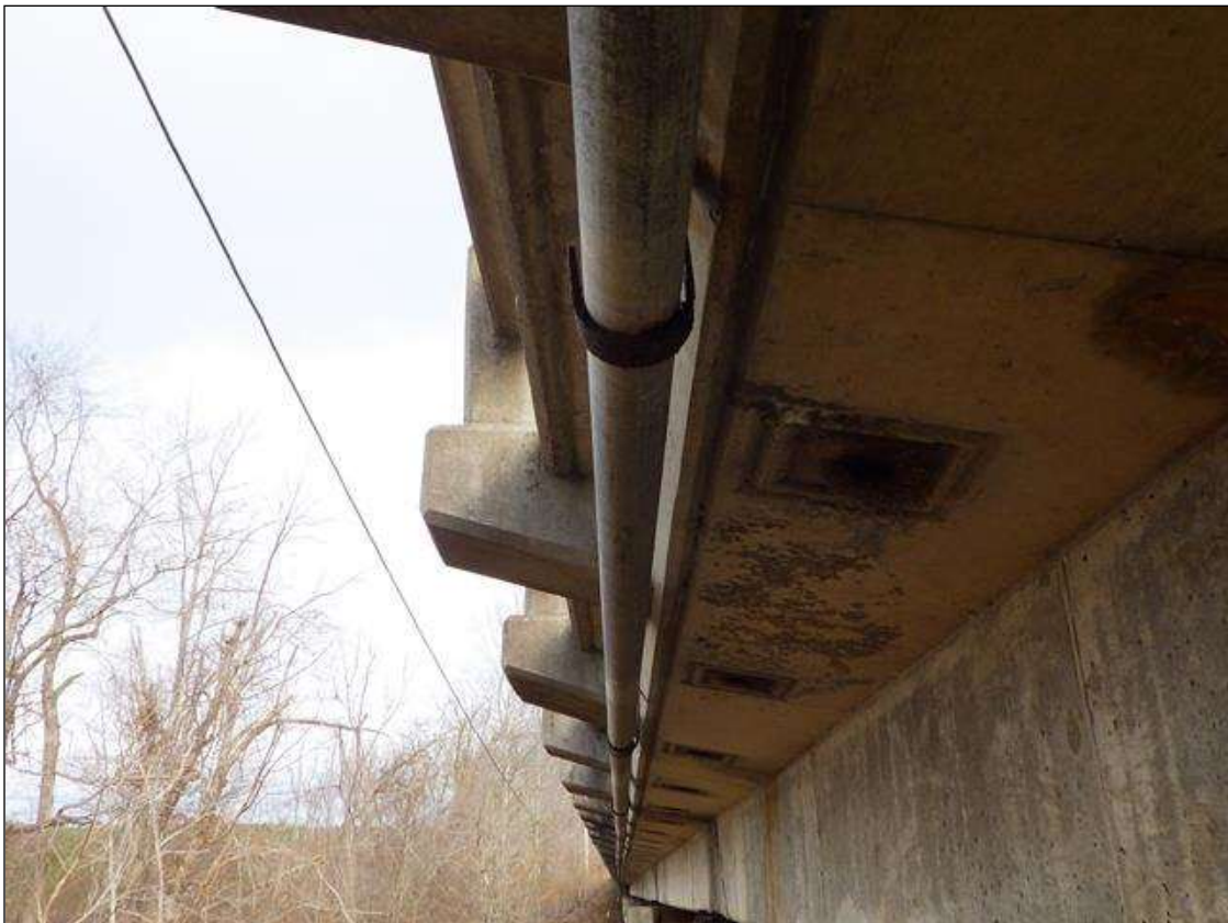
utility at west overhang, metal pipe (3-1/2" diameter)
