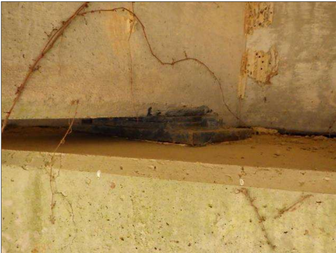
end bearing assembly
