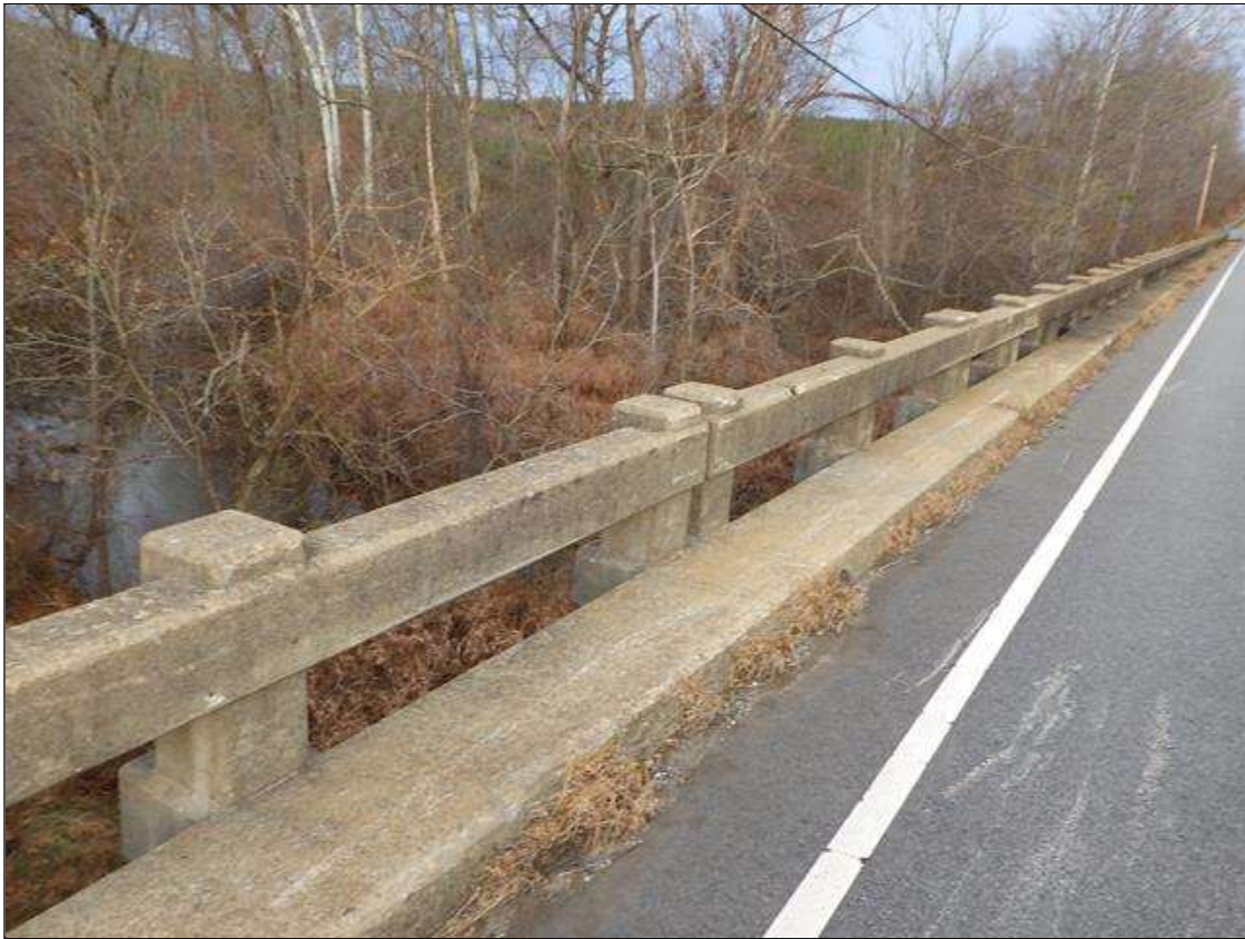
west bridge rail
