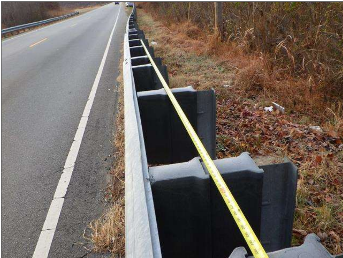
southwest guardrail and post spacing
