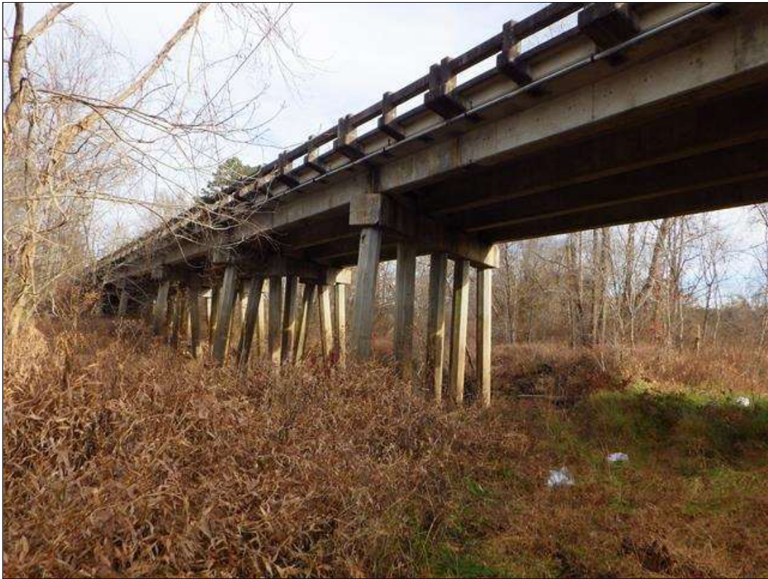
upstream profile, looking east
