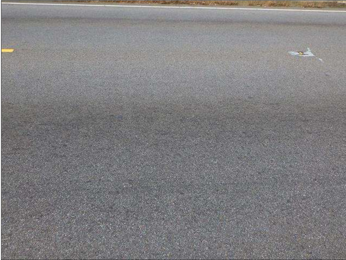
asphalt wearing surface
