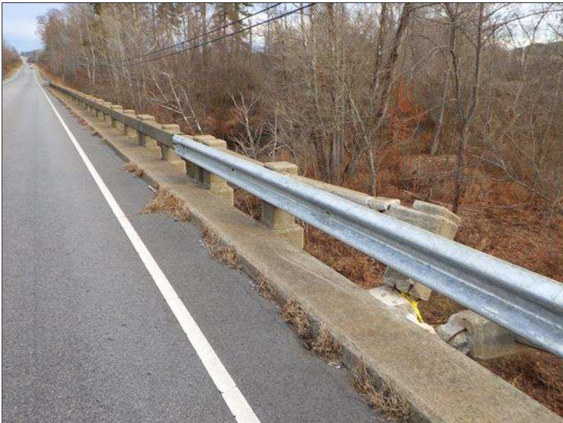
east bridge rail
