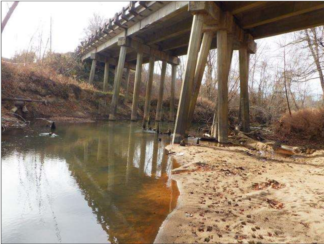
stream underview looking upstream, west (span 3)
