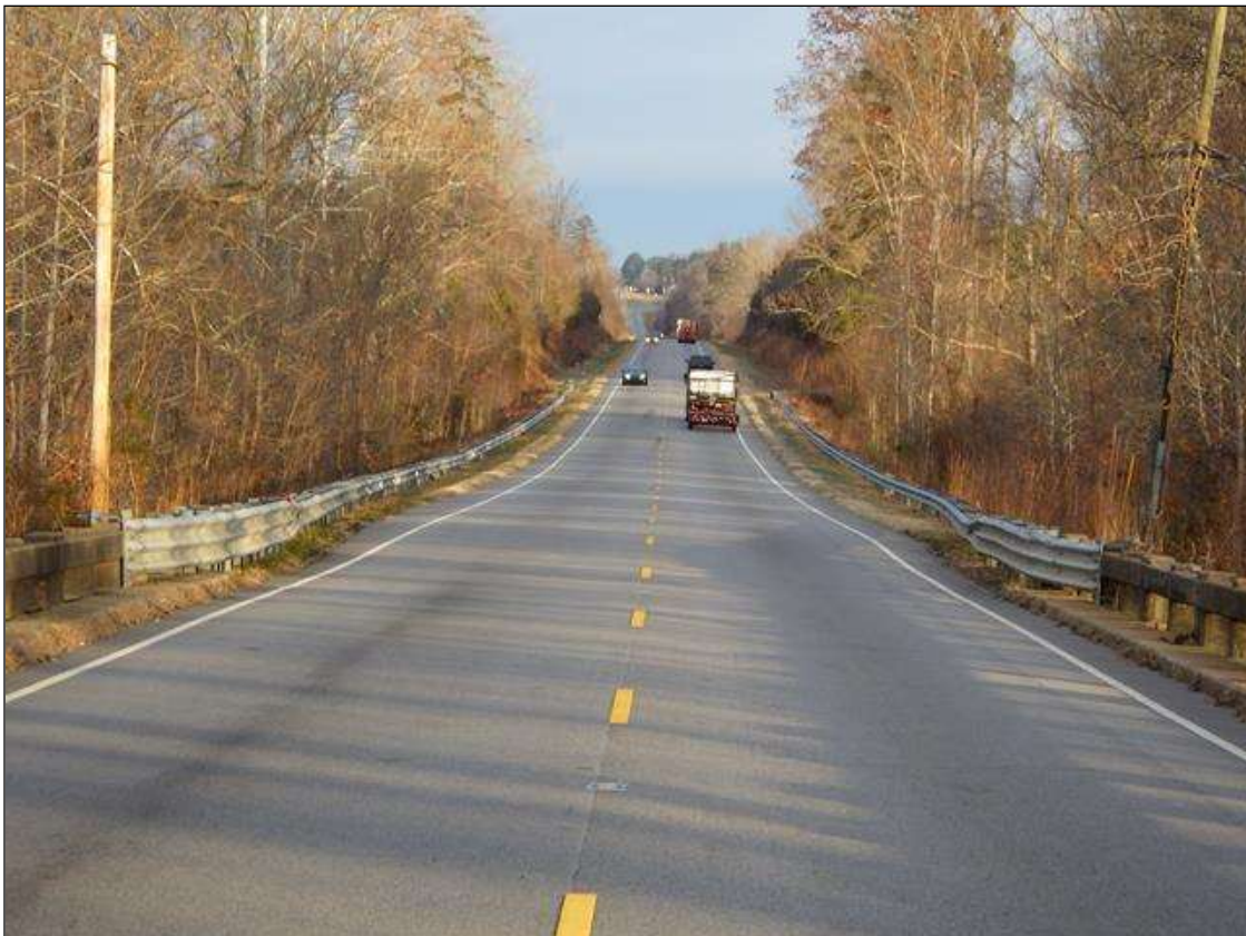
north approach, looking north (upstation)
