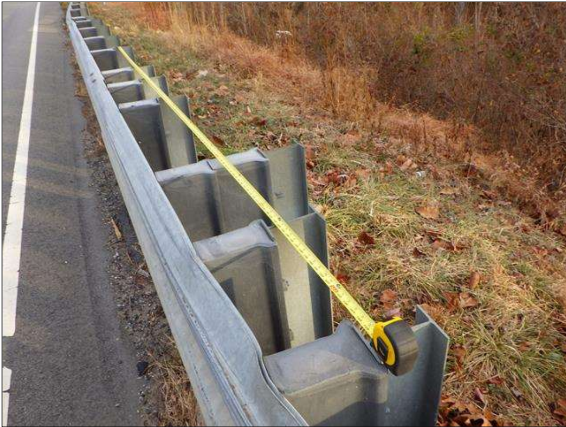
northeast guardrail and post spacing
