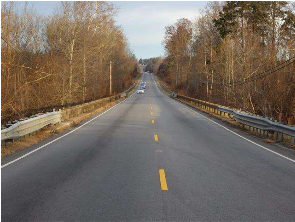
south approach, looking north
