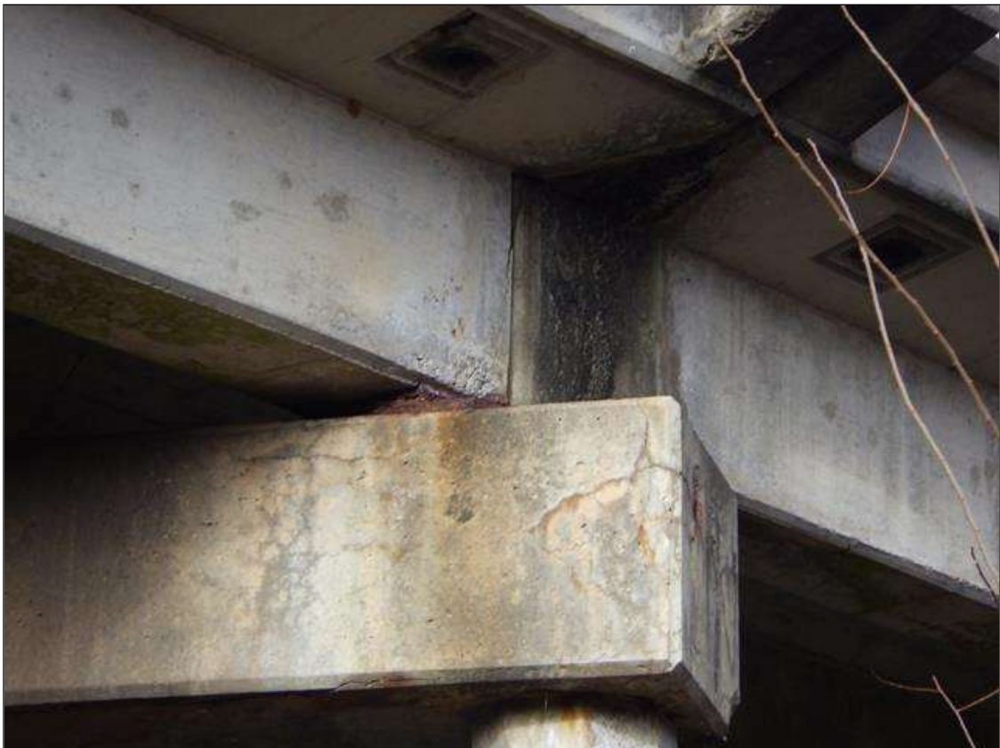
beams over bent 2
