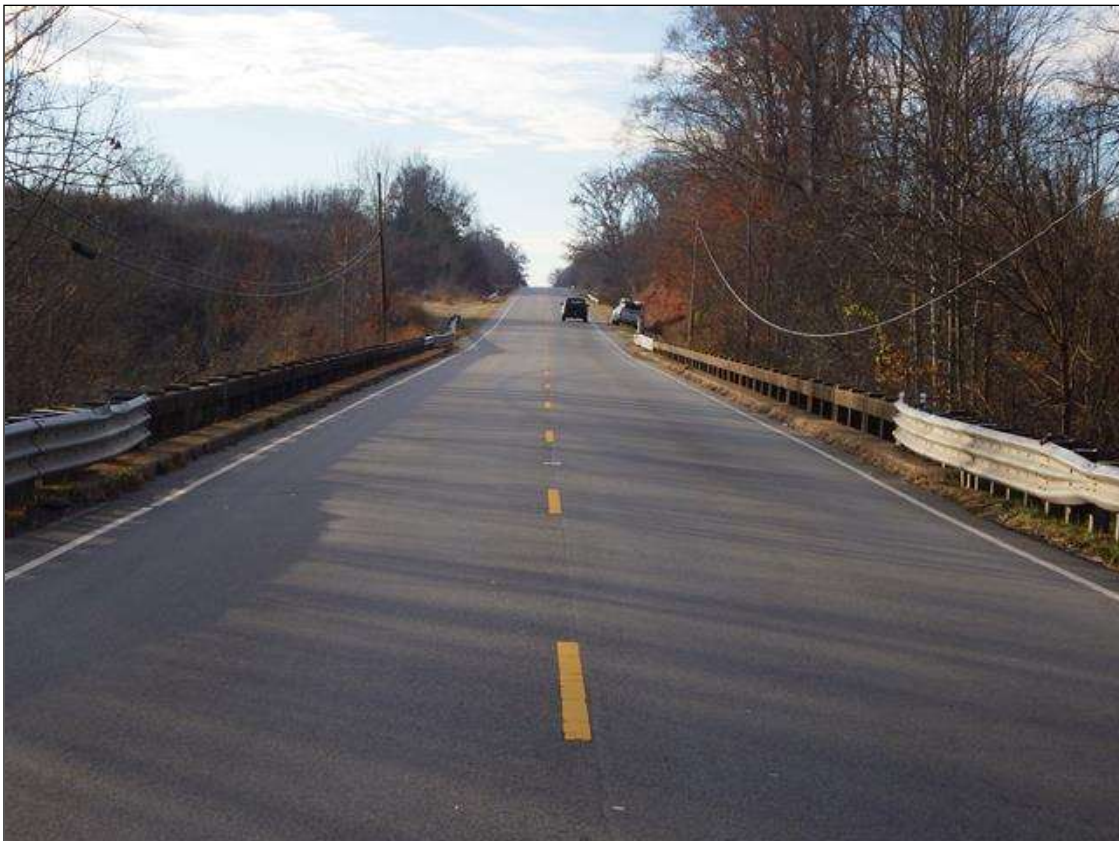
north approach, looking south
