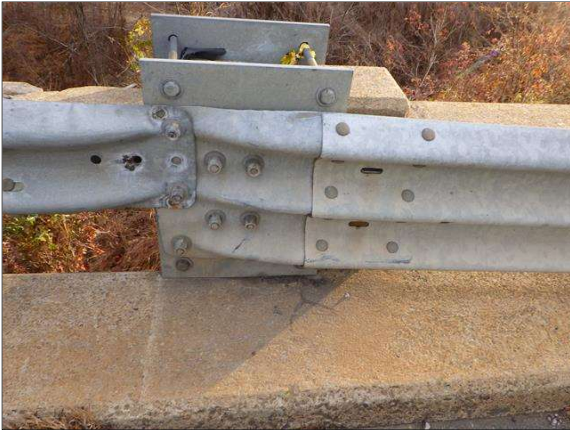
southeast guardrail attachment
