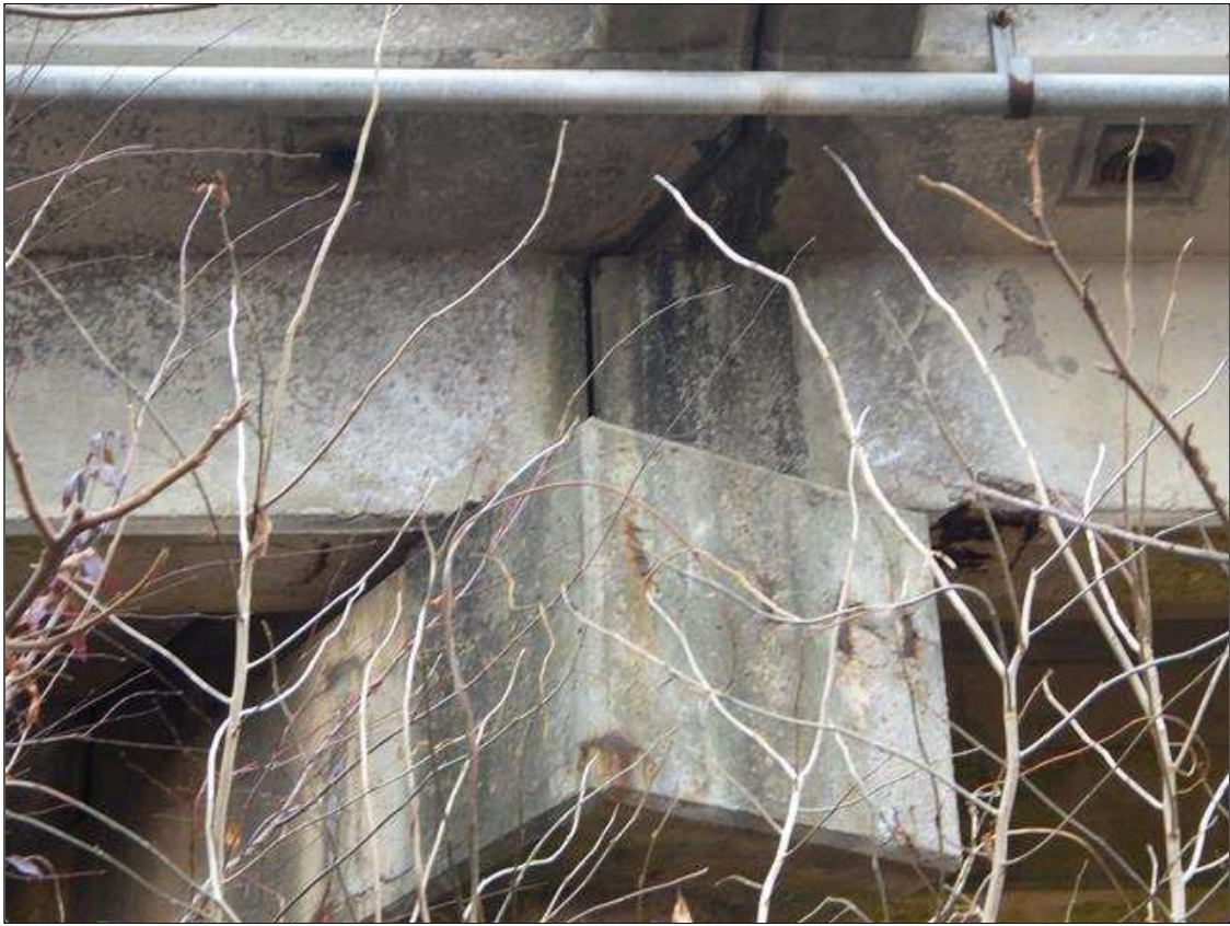
beams over bent 6
