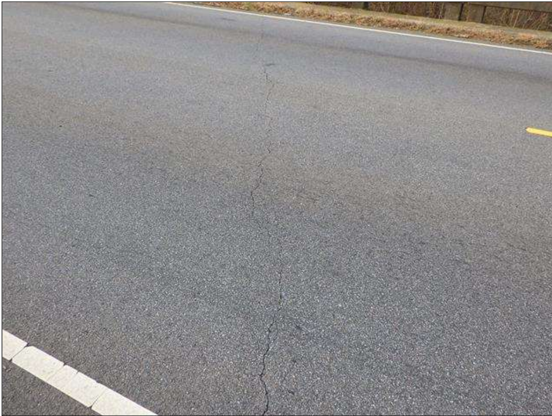
asphalt wearing surface over bent 6
