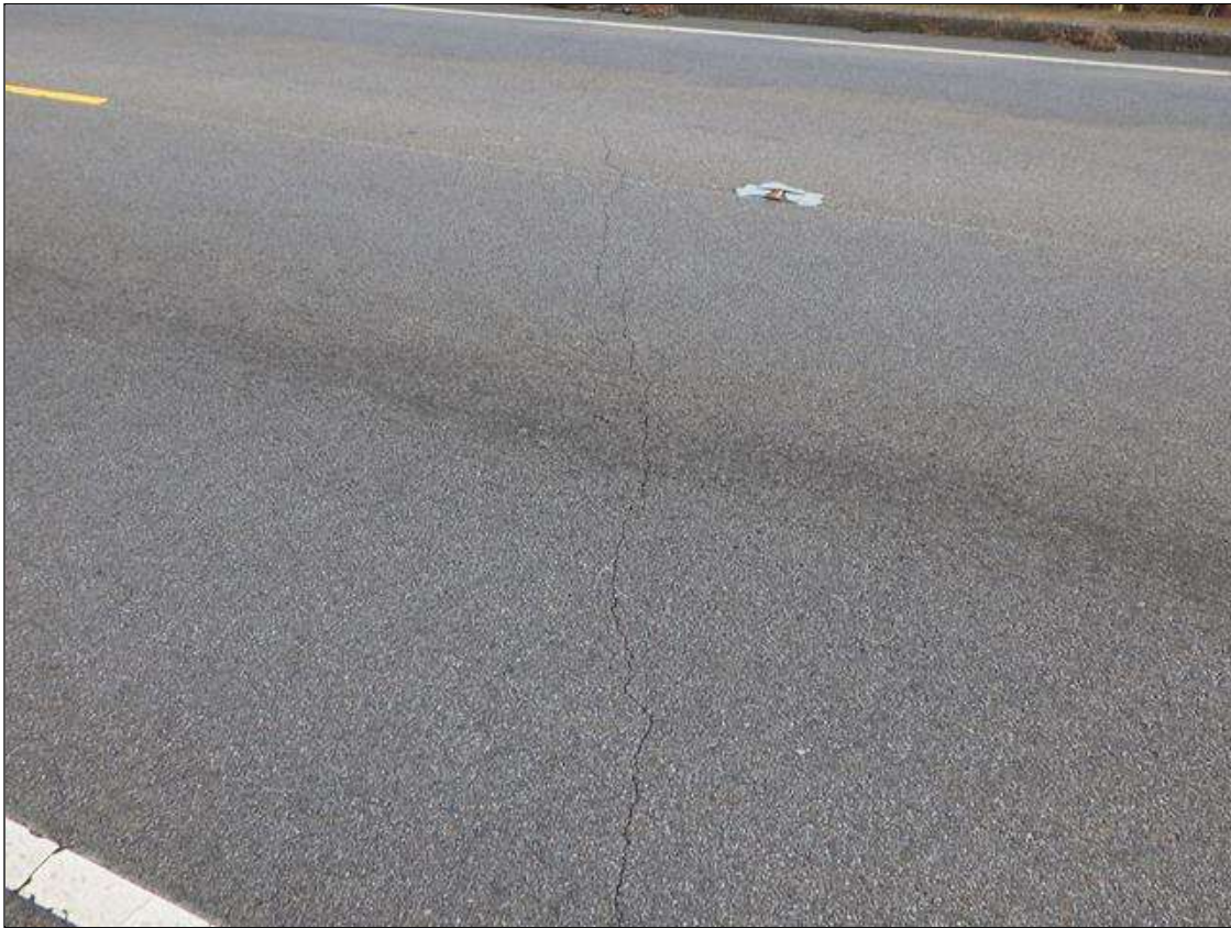
asphalt wearing surface over bent 3
