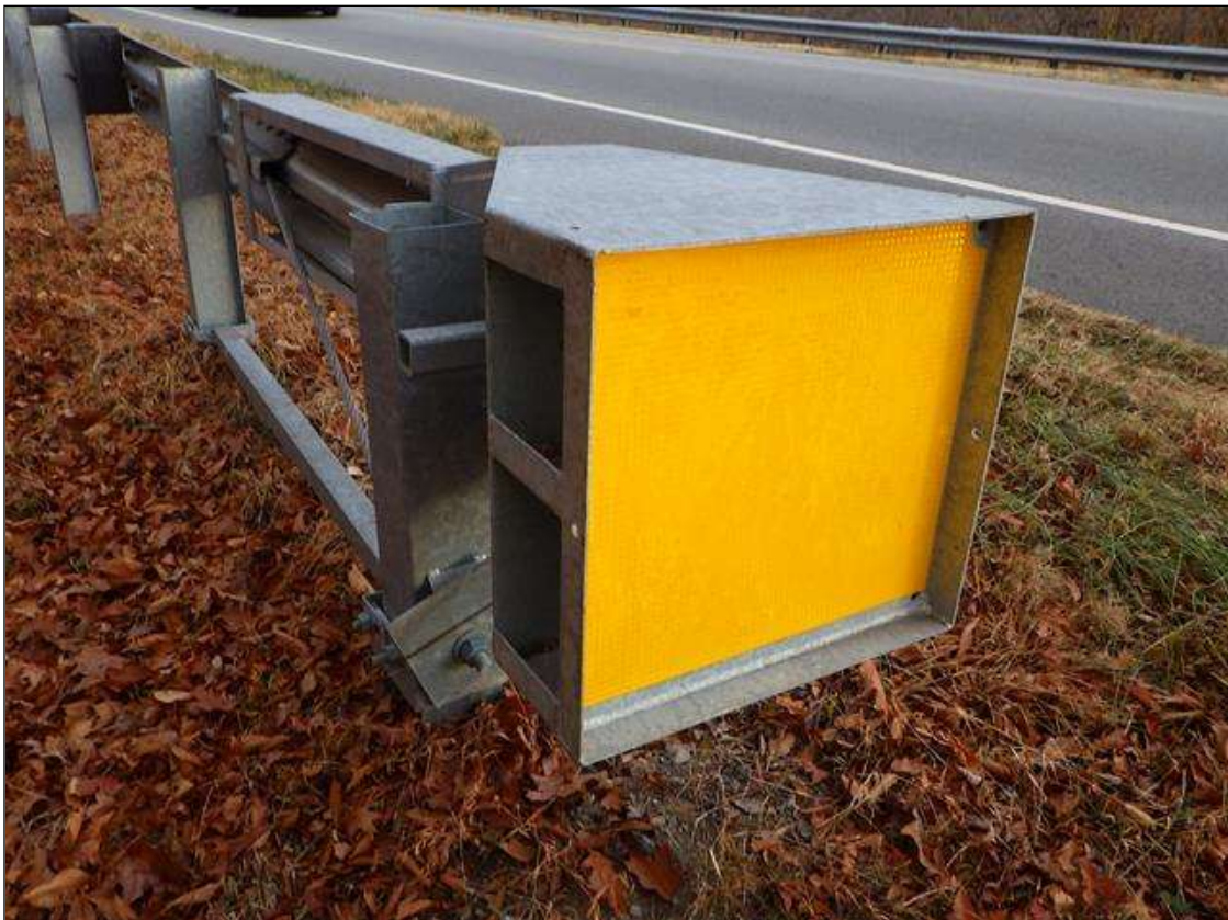
southwest guardrail termination
