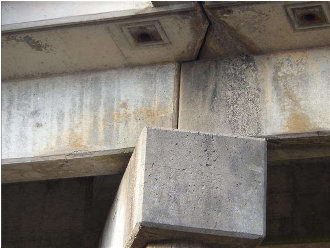
beams over bent 1
