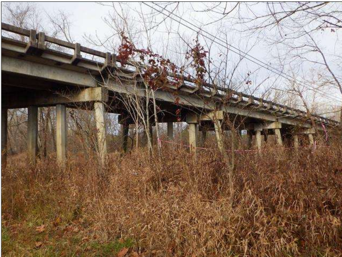
downstream profile, looking west
