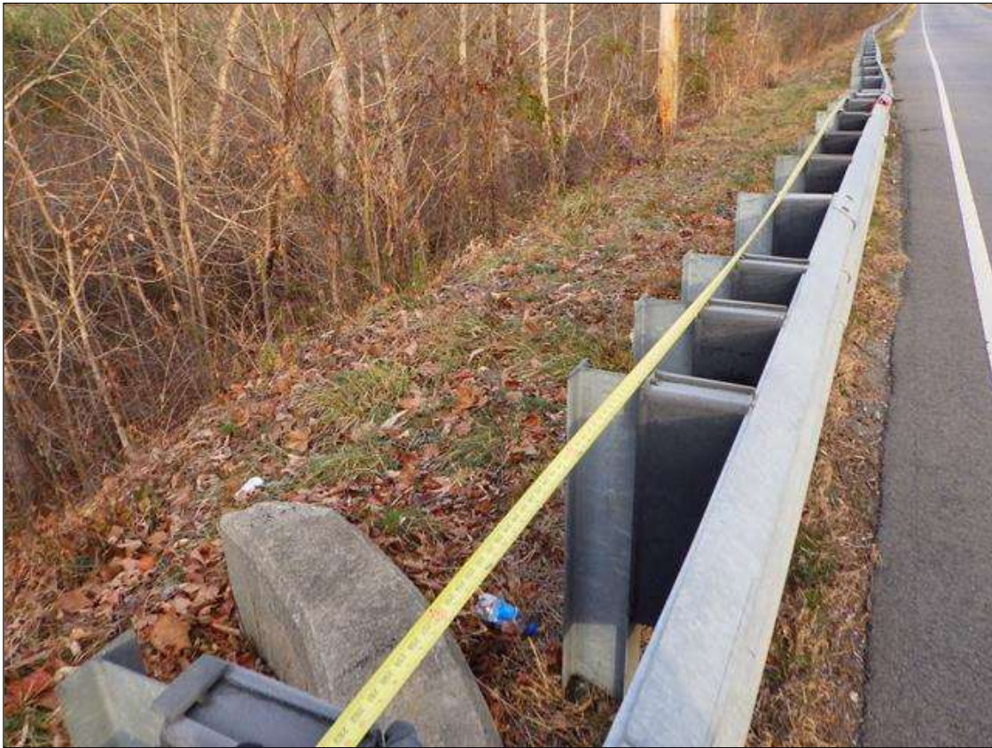
northwest guardrail and post spacing
