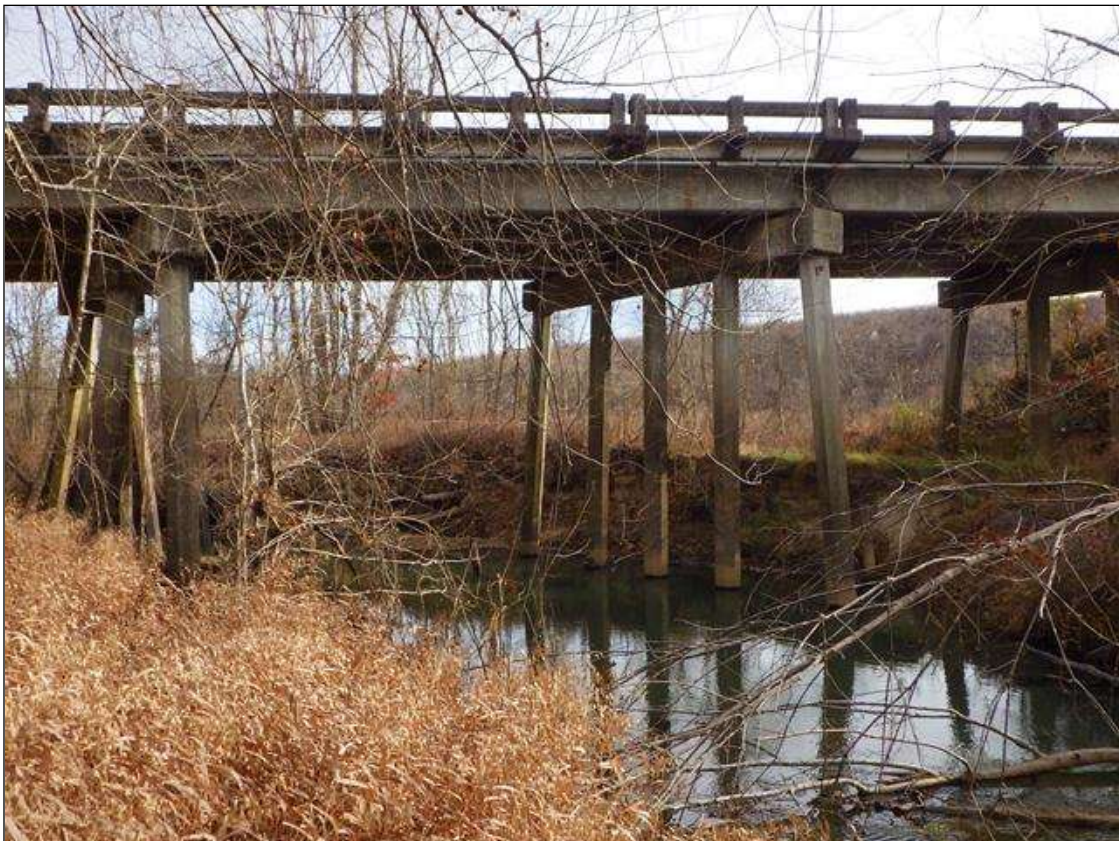
stream underview looking downstream, east (span 3)
