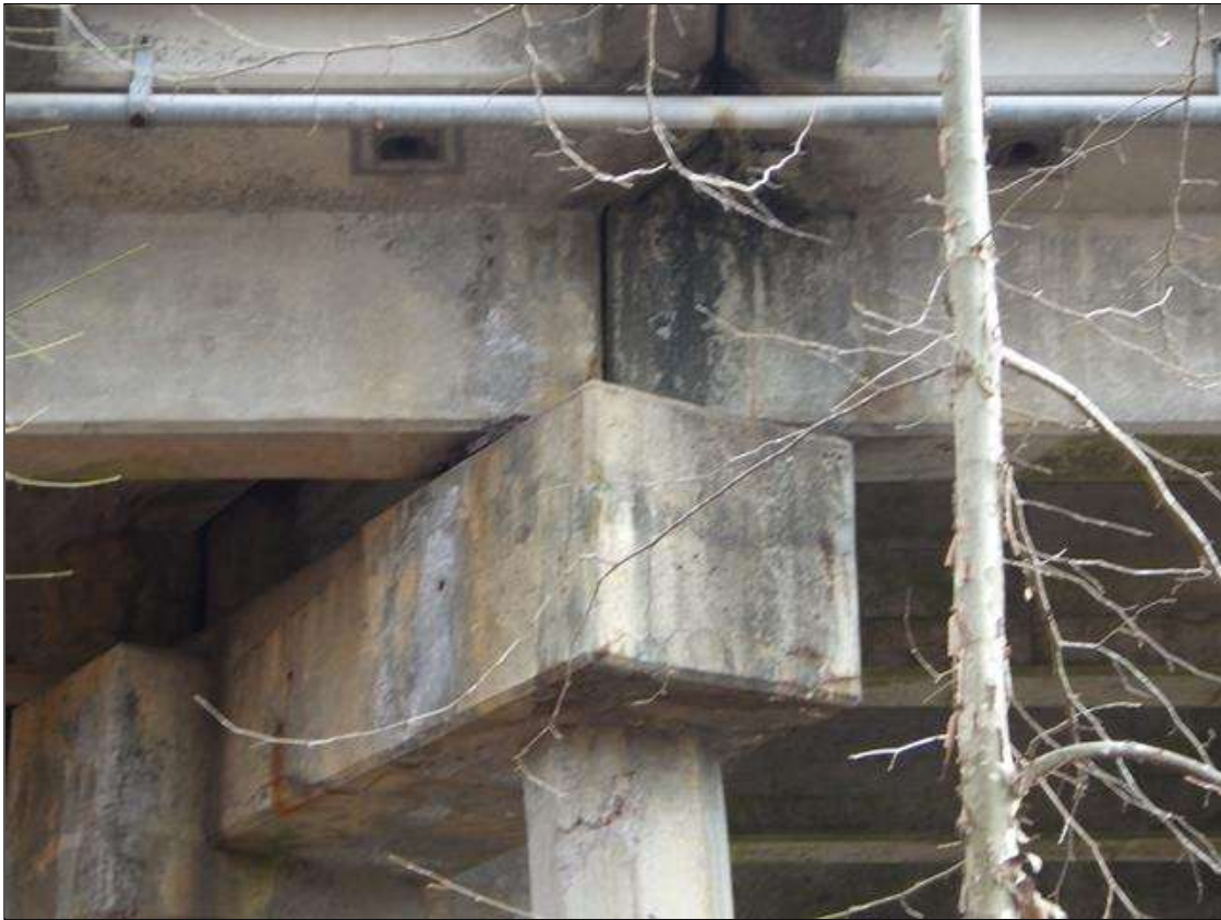
beams over bent 3
