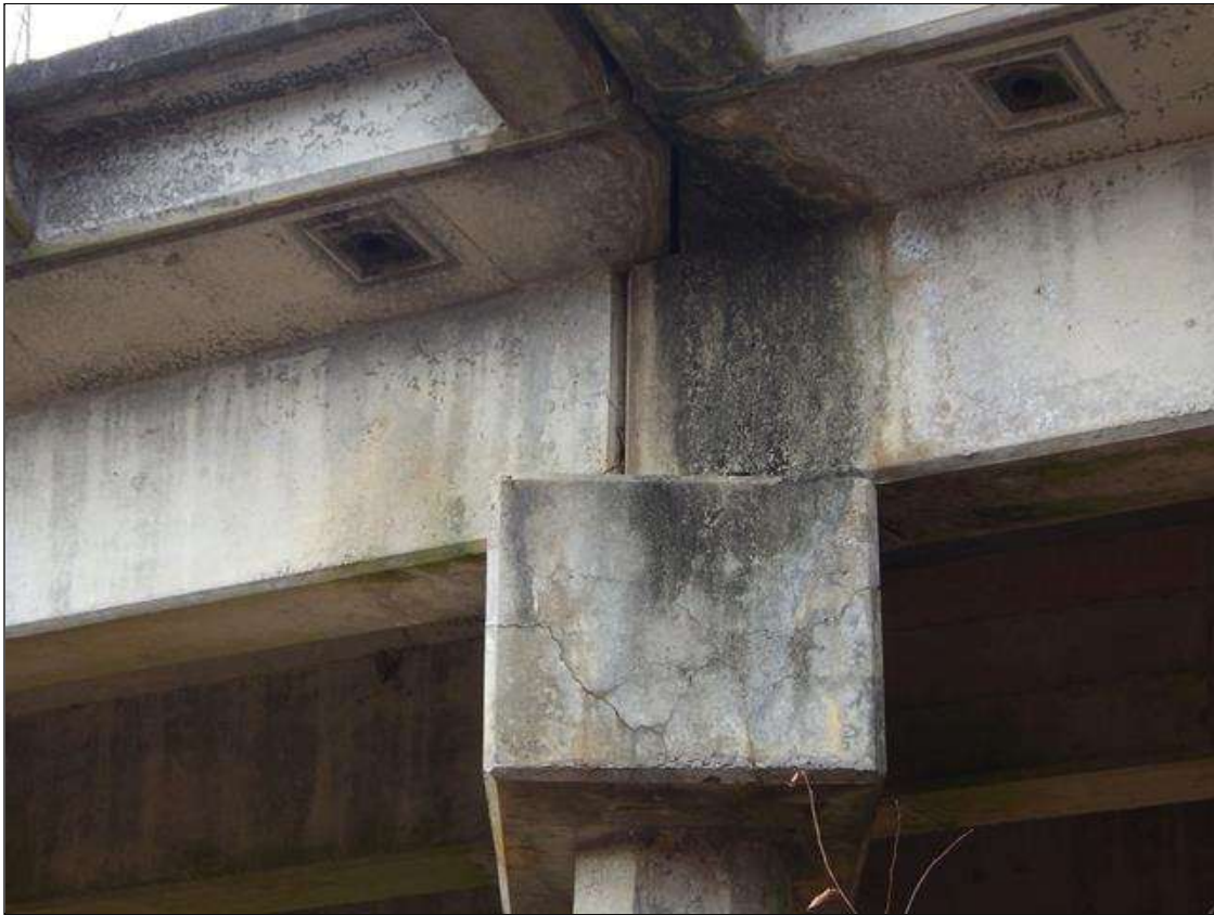
beams over bent 5
