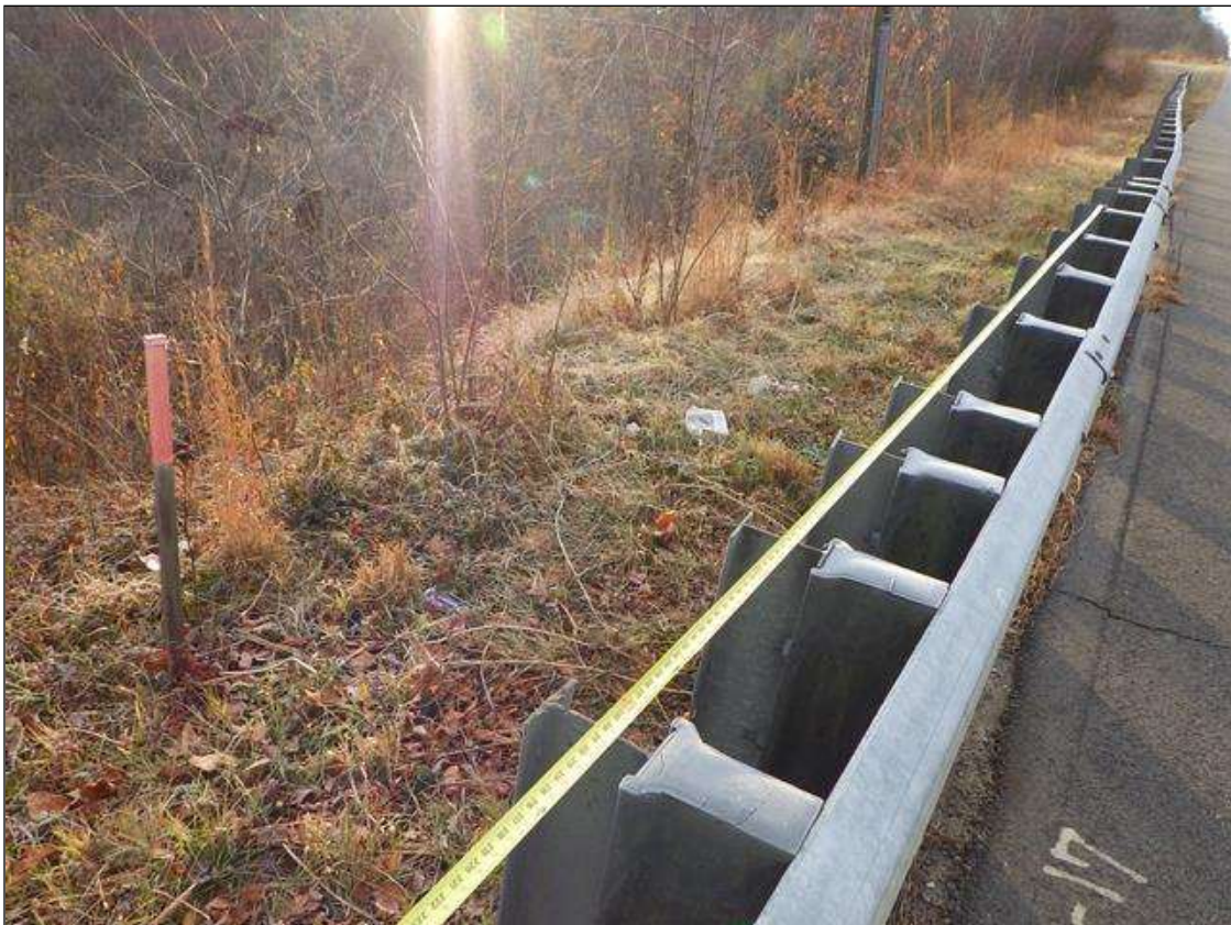
southeast guardrail and post spacing
