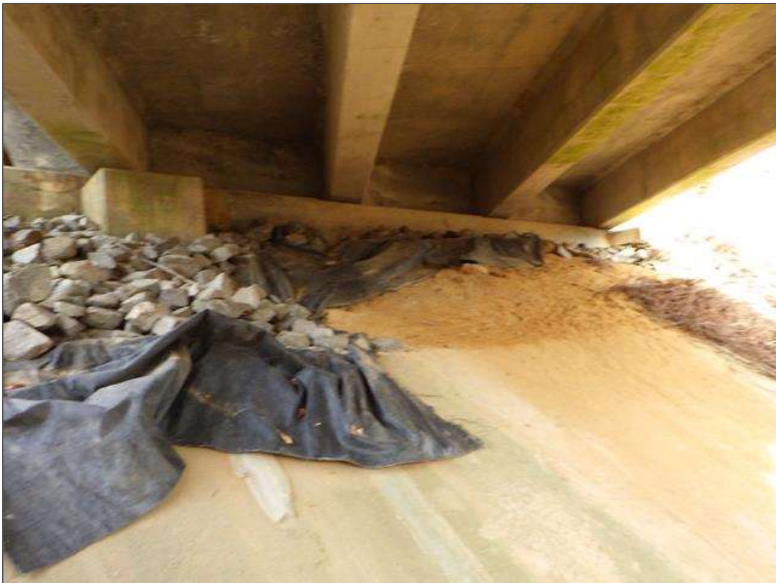
end bent 2 and slope protection
