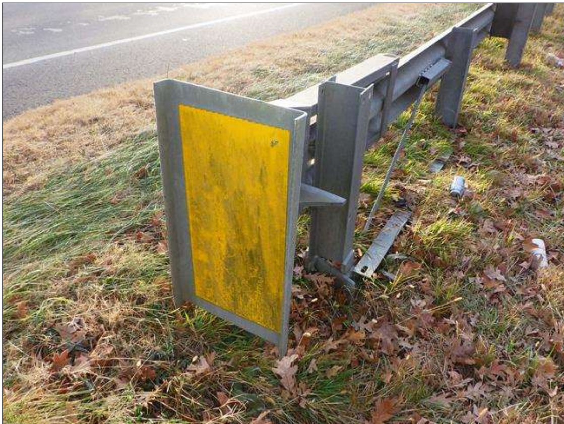
northwest guardrail termination
