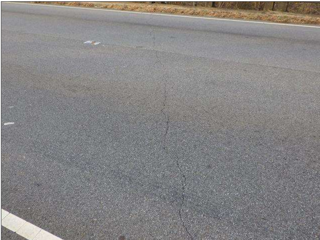
asphalt wearing surface over bent 5
