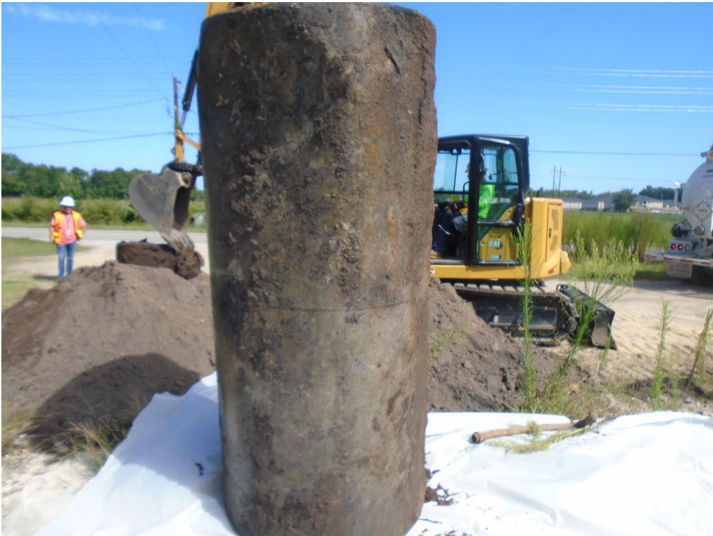
Photograph 5 – The 1,000-gallon capacity UST being positioned so the bottom can be inspected for holes.
