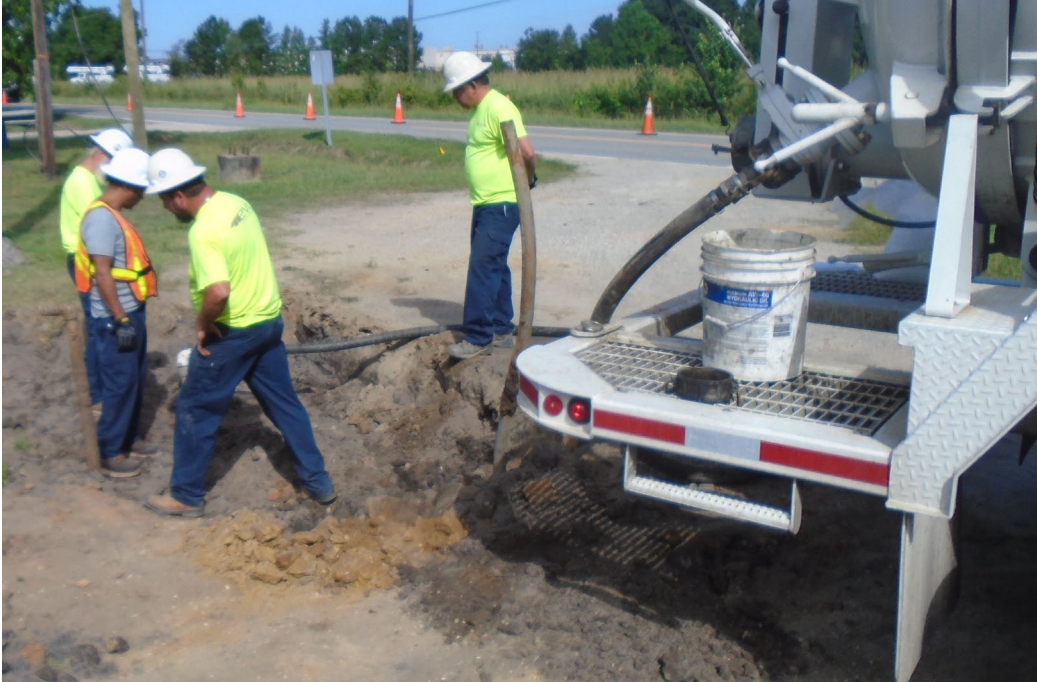
Photograph 3 – Vacuum truck evacuating the contents of the USTs.
