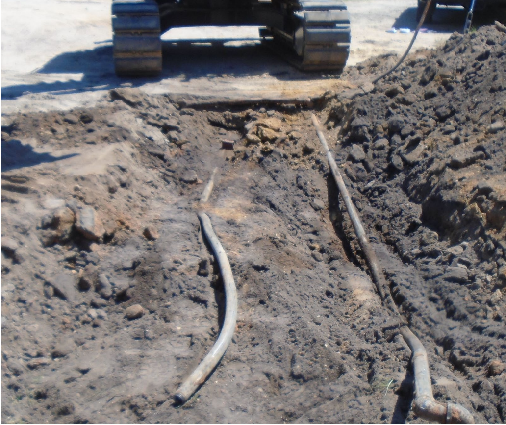
Photograph 7 – View of fuel lines being uncovered prior to sampling.
