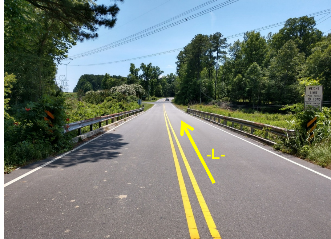
View of SR 2044 looking south.
