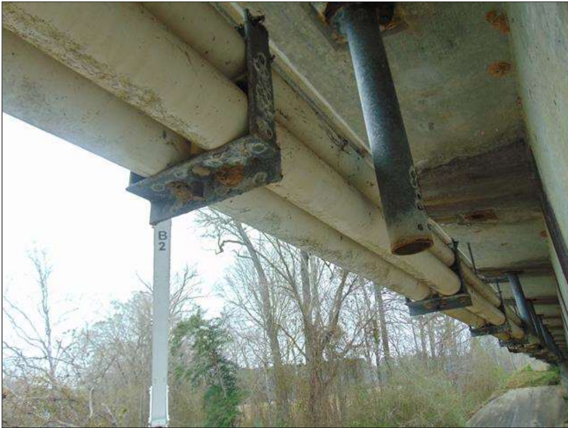
(4) 4" diameter utilities in North overhang
