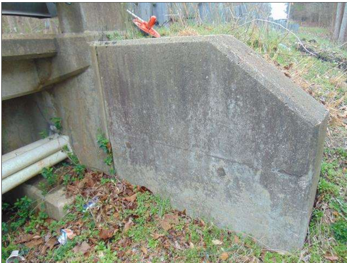
Northwest wingwall (All others similar)
