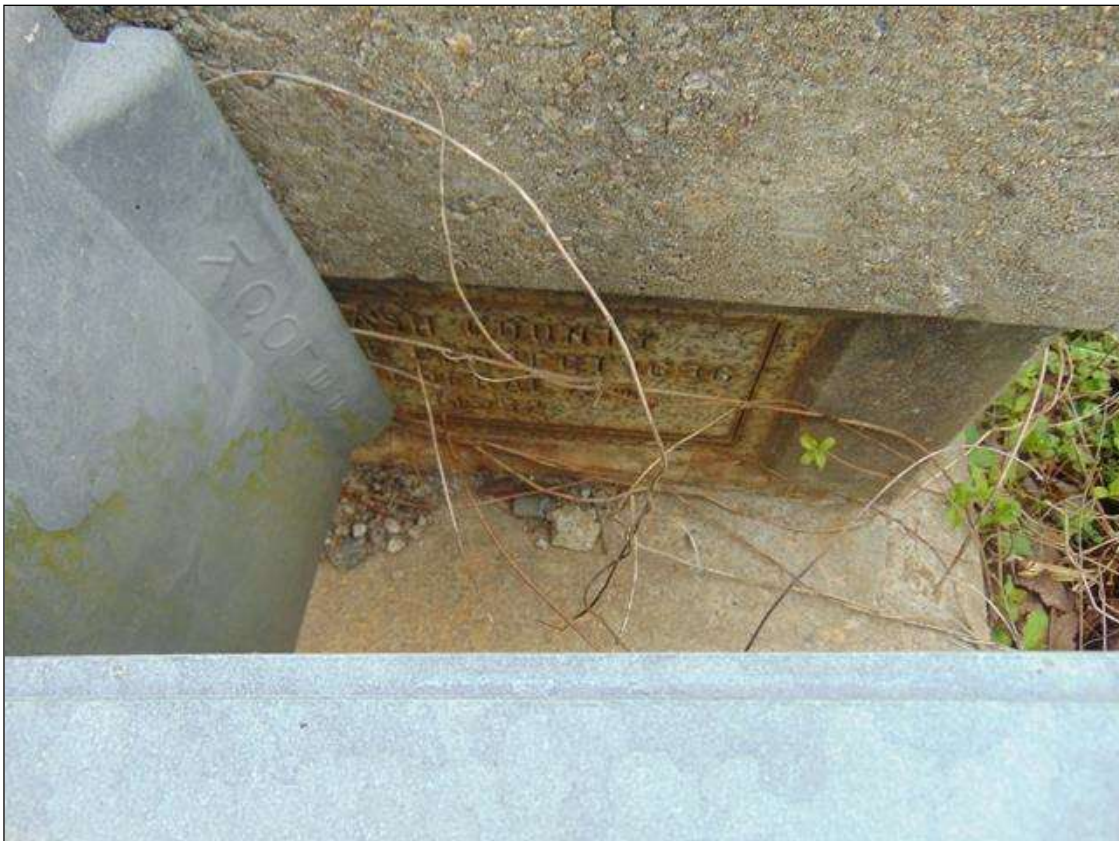
Bridge plaque at Northeast corner (Southwest corner similar)
