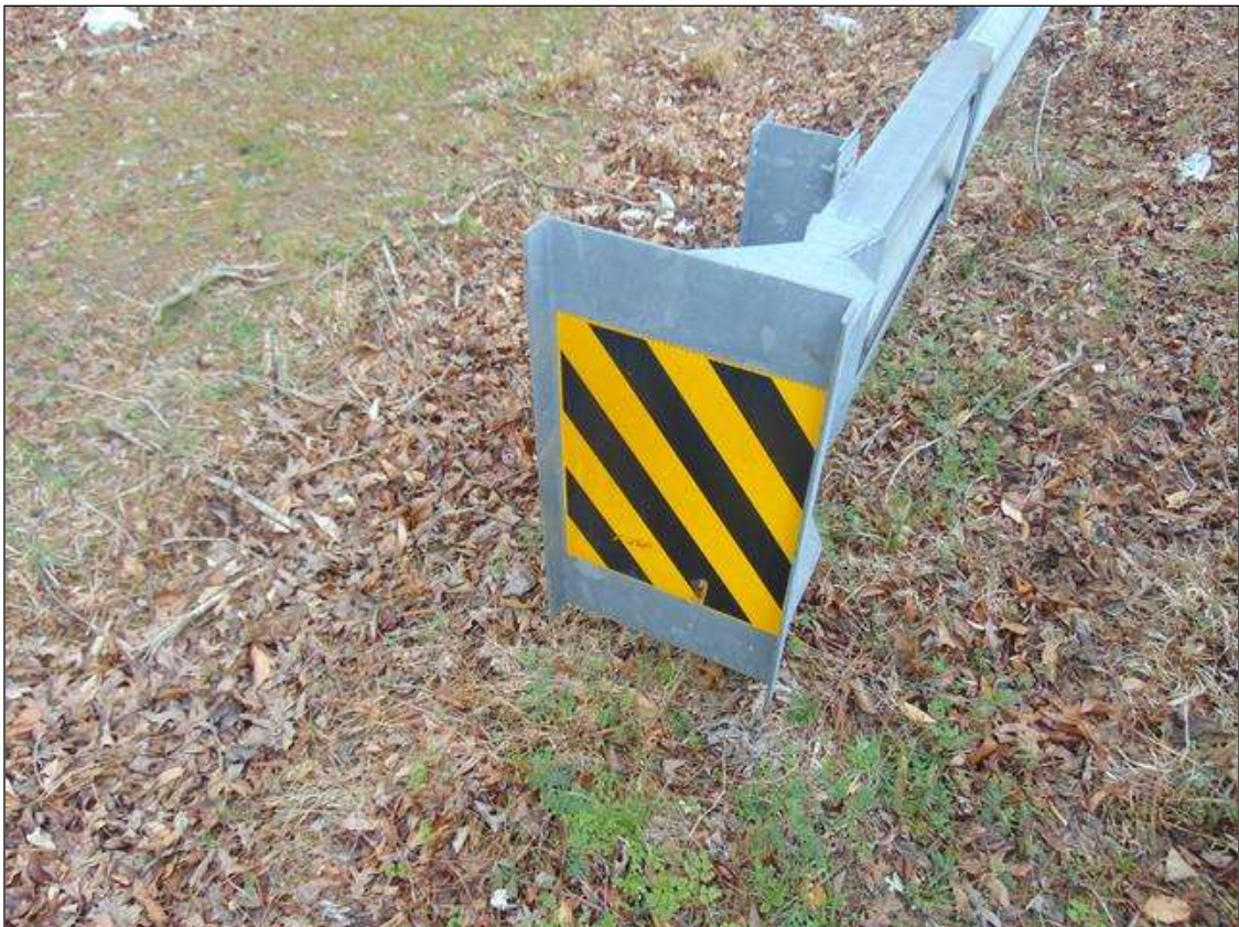
Northwest guardrail end treatment (All others similar)
