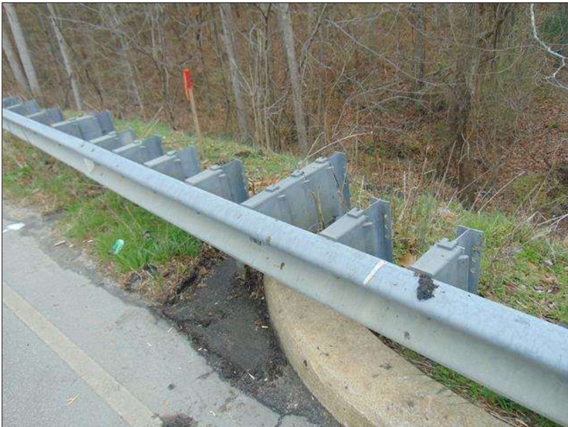
Northwest guardrail transition (All others similar)
