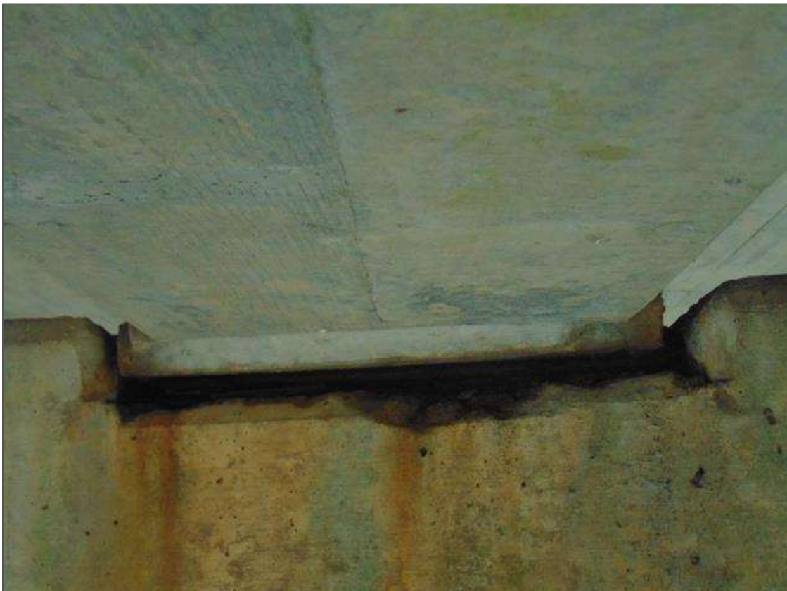
Bent bearing (Beam 3, Bent 6 shown)
