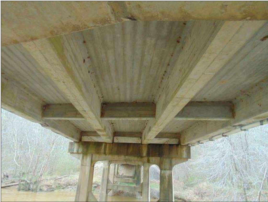
Underside of superstructure (Span 5 shown)
