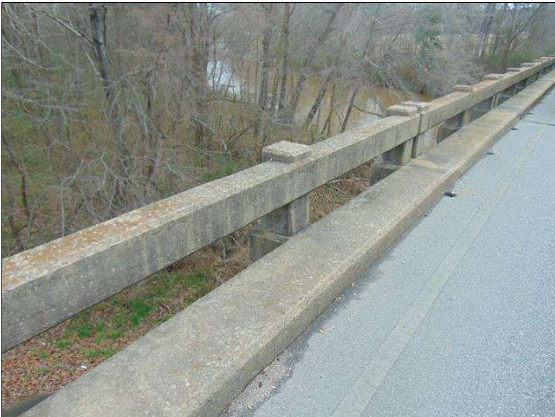
North bridge rail (South bridge rail similar)
