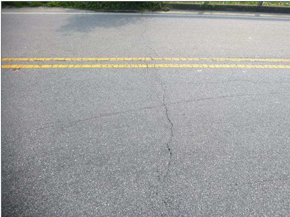
asphalt wearing surface over end bent 1
