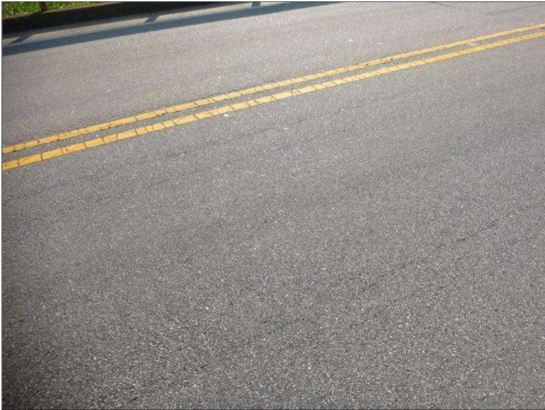
asphalt wearing surface
