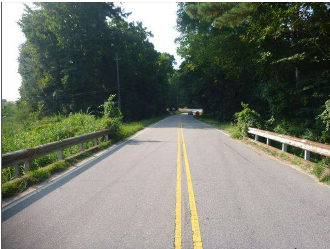
north approach, looking north (upstation)
