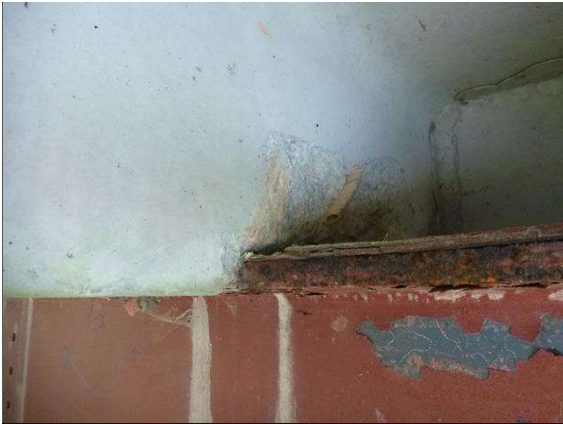
Span 2 Slab 5: (PAR) left and right leg at bent 1, two [2] spalls [up to 12in x 8in x up to full width], with exposed stirrup [no section loss noted] channel legs crushing and bottom of channel legs sits below top of crutch bent cap (photo 2 of 2)
