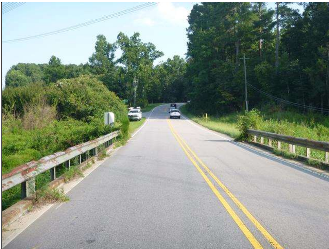
south approach, looking south (backstation)
