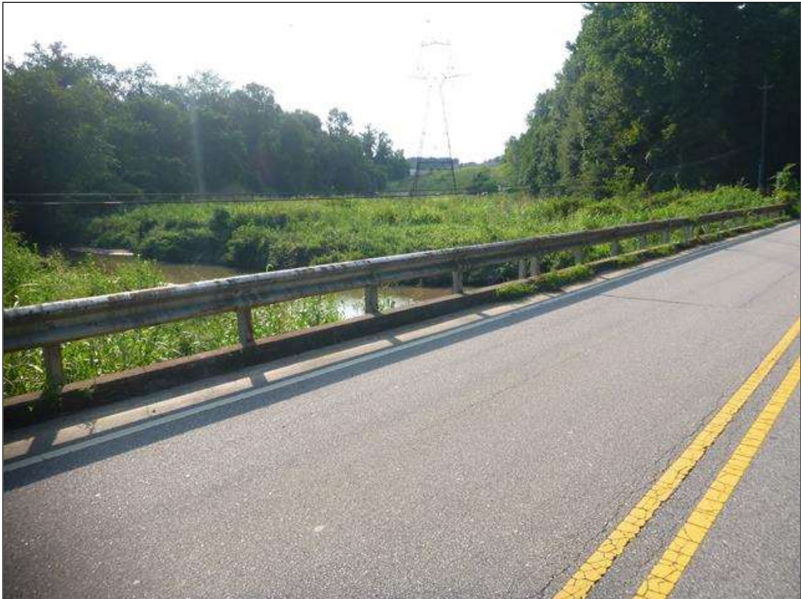
west bridge rail
