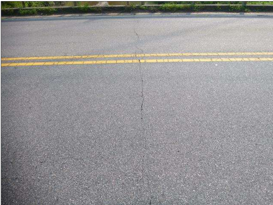
asphalt wearing surface over bent 2
