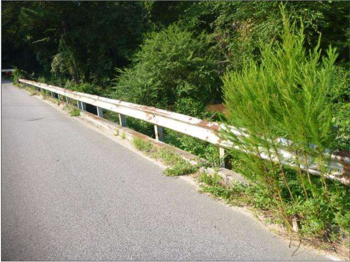
east bridge rail
