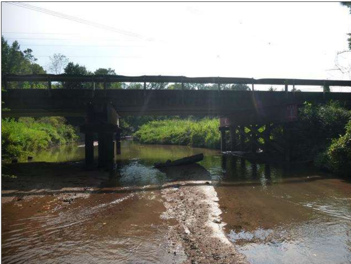
upstream profile, looking west
