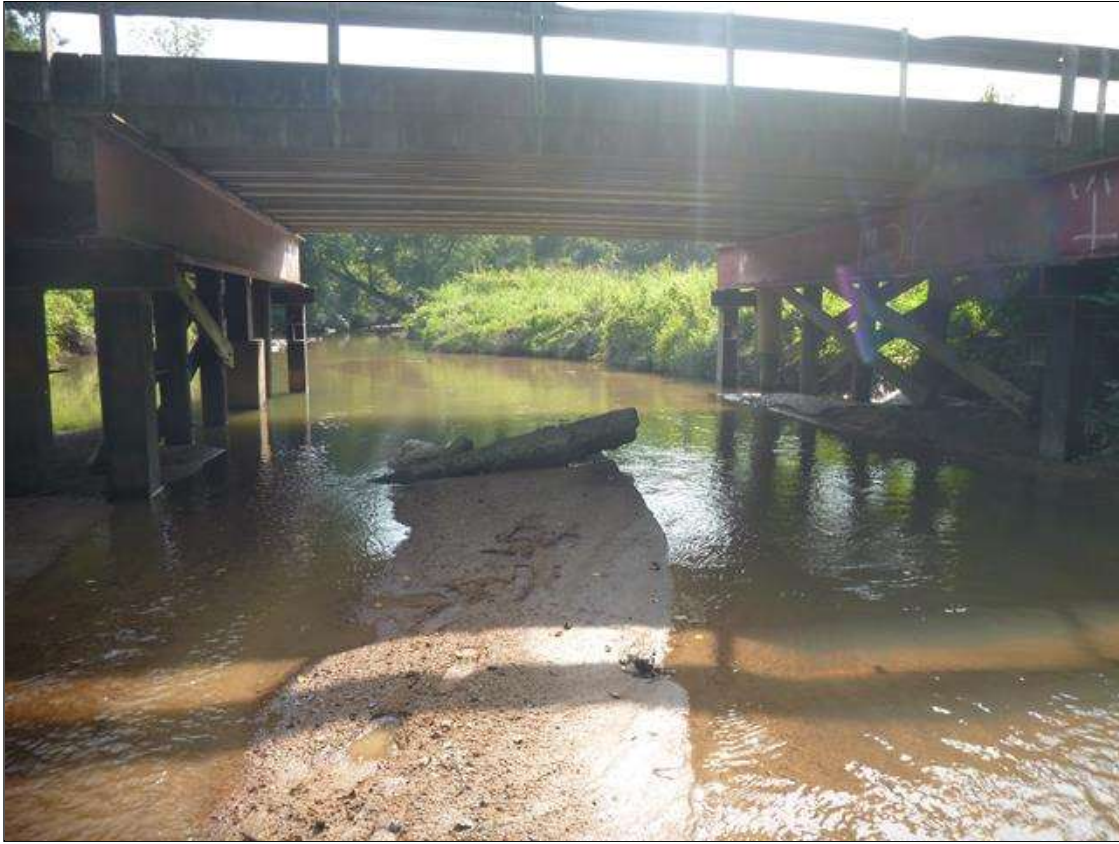
stream under view looking downstream, west (span 2)
