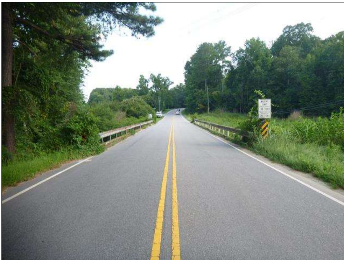
north approach, looking south
