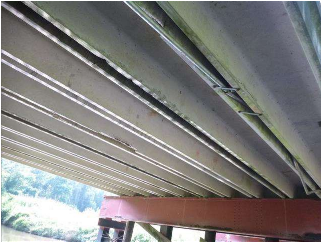
underside of channels (span 2)
