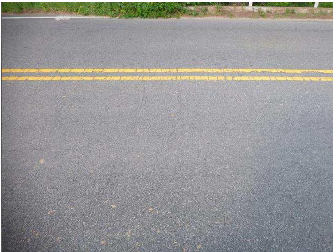
asphalt wearing surface over end bent 2
