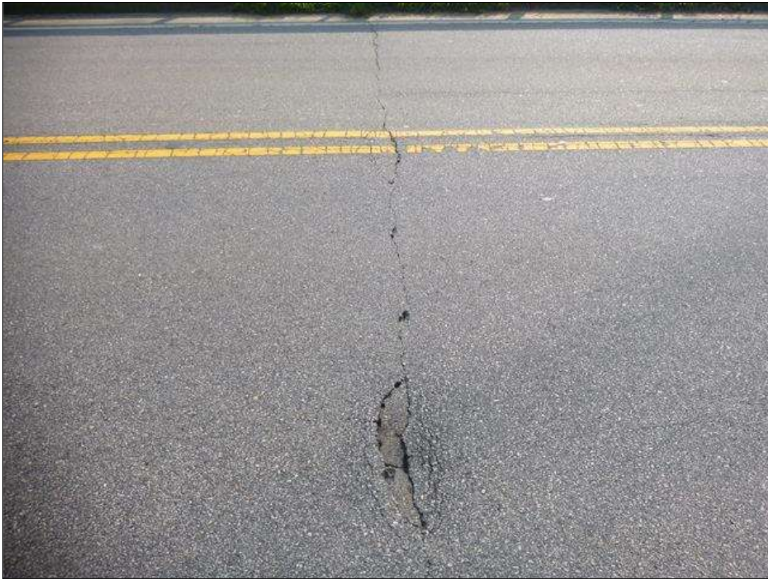
asphalt wearing surface over bent 1
