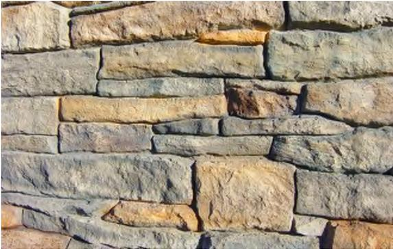
All texture is to be in addition to the nominal thickness of each element within tolerances. Relief of any texture is to have a minimum depth of  $\frac{1}{2}$  inch, a maximum depth of 4 inches, and an average of  $2\frac{1}{2}$  inches.
