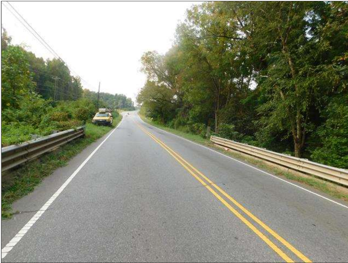
LOOKING SOUTH FROM DECK
