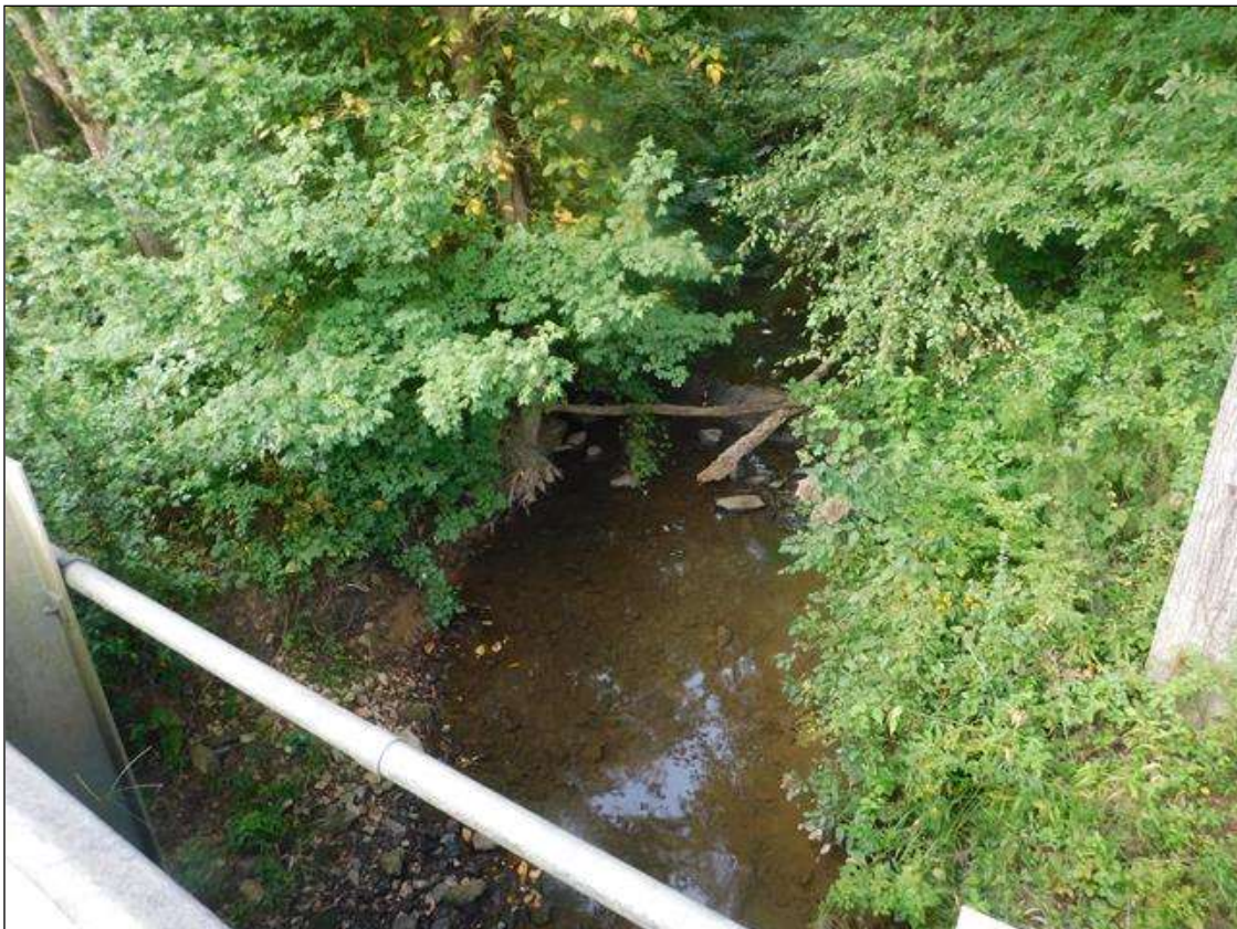
LOOKING UPSTREAM WEST FROM TOP
