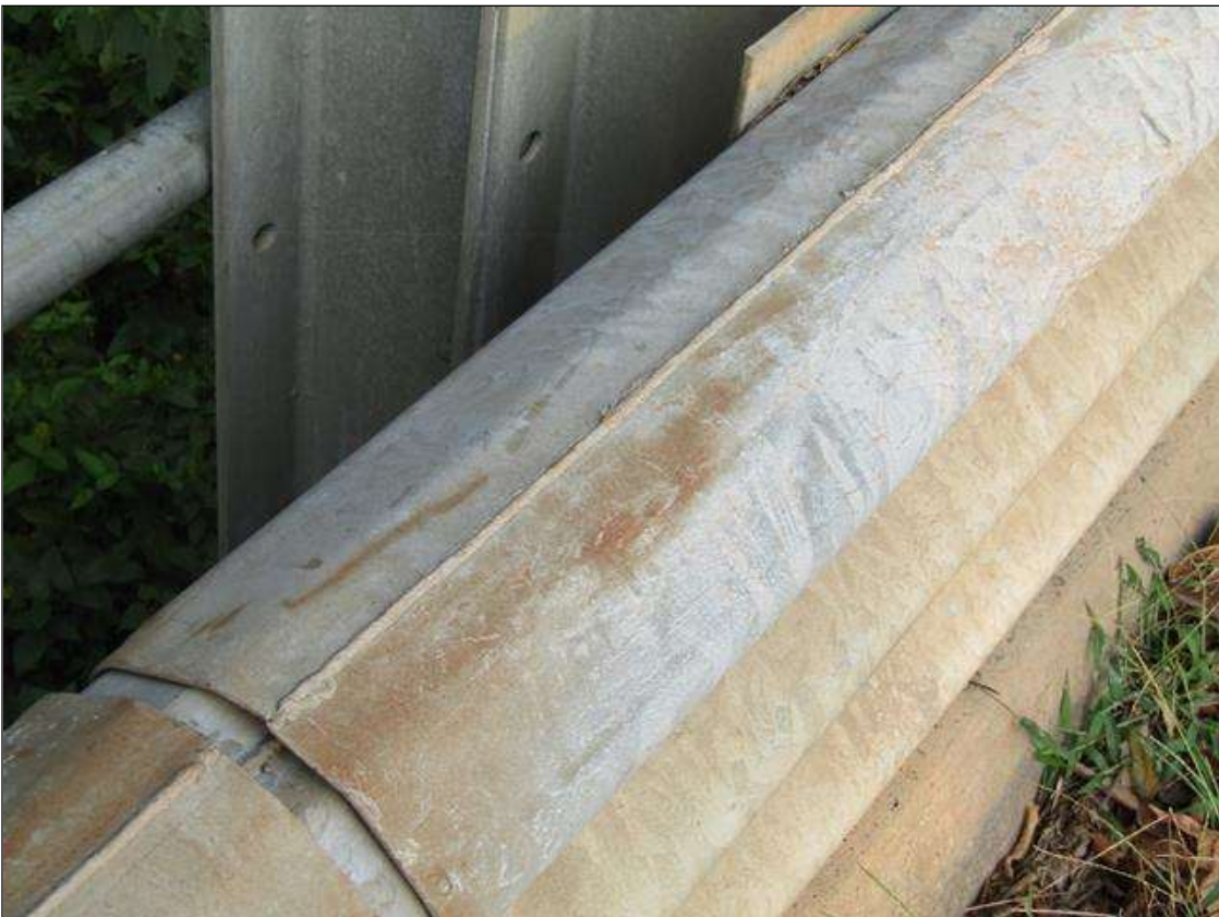
Span 1 Left Bridge Rail - Protective System: SUBSTANTIALLY EFFECTIVE ON TOP
