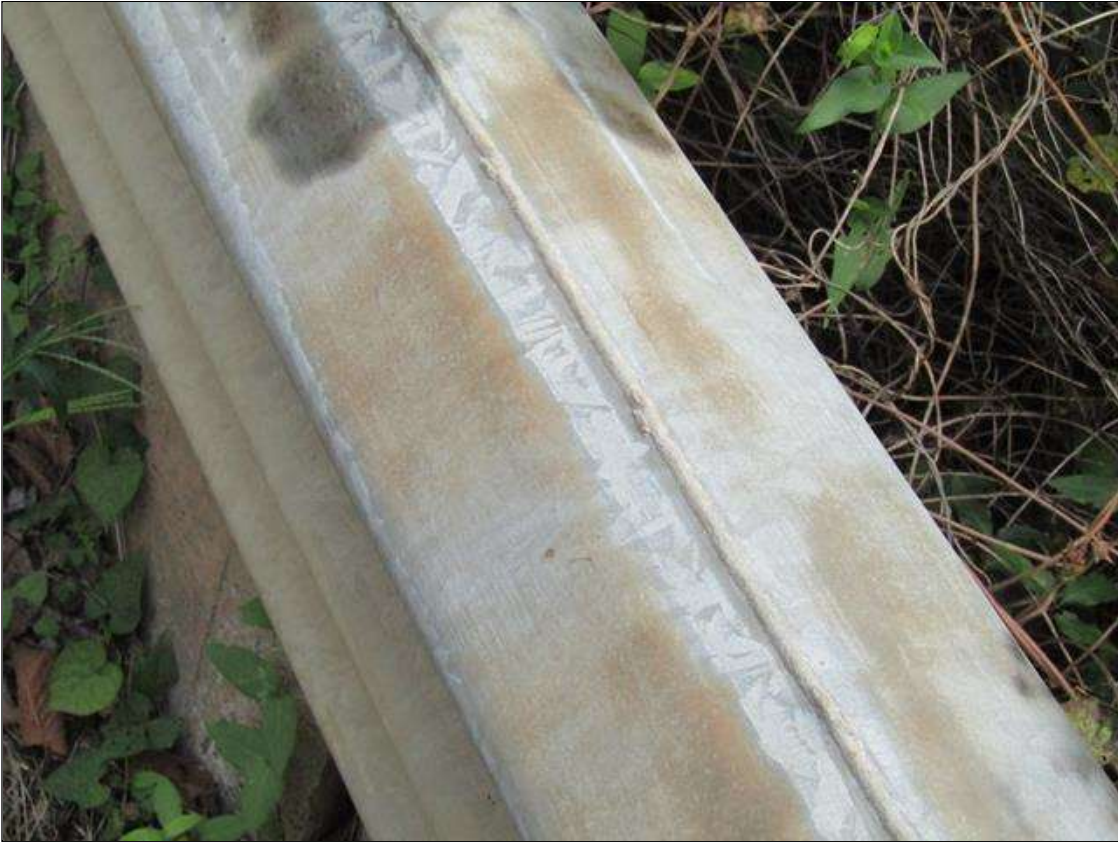
Span 1 Right Bridge Rail - Protective System: SUBSTANTIALLY EFFECTIVE ON TOP
