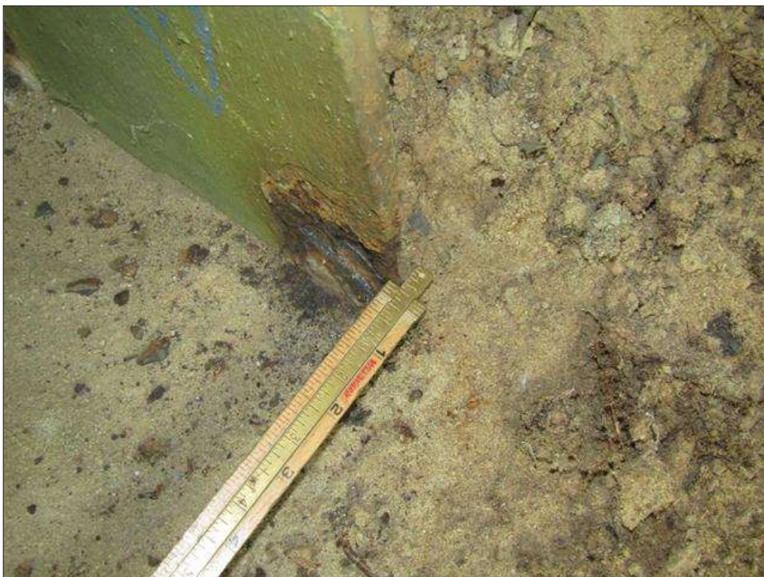
Bent 2 Pile 5: RUST SCALE ON BOTTOM OF SOUTH FLANGE ON EAST SIDE UP 3" X 2" WIDE WITH 1/8" STEEL REMAINING ON 1/2" FLANGE/PAR
