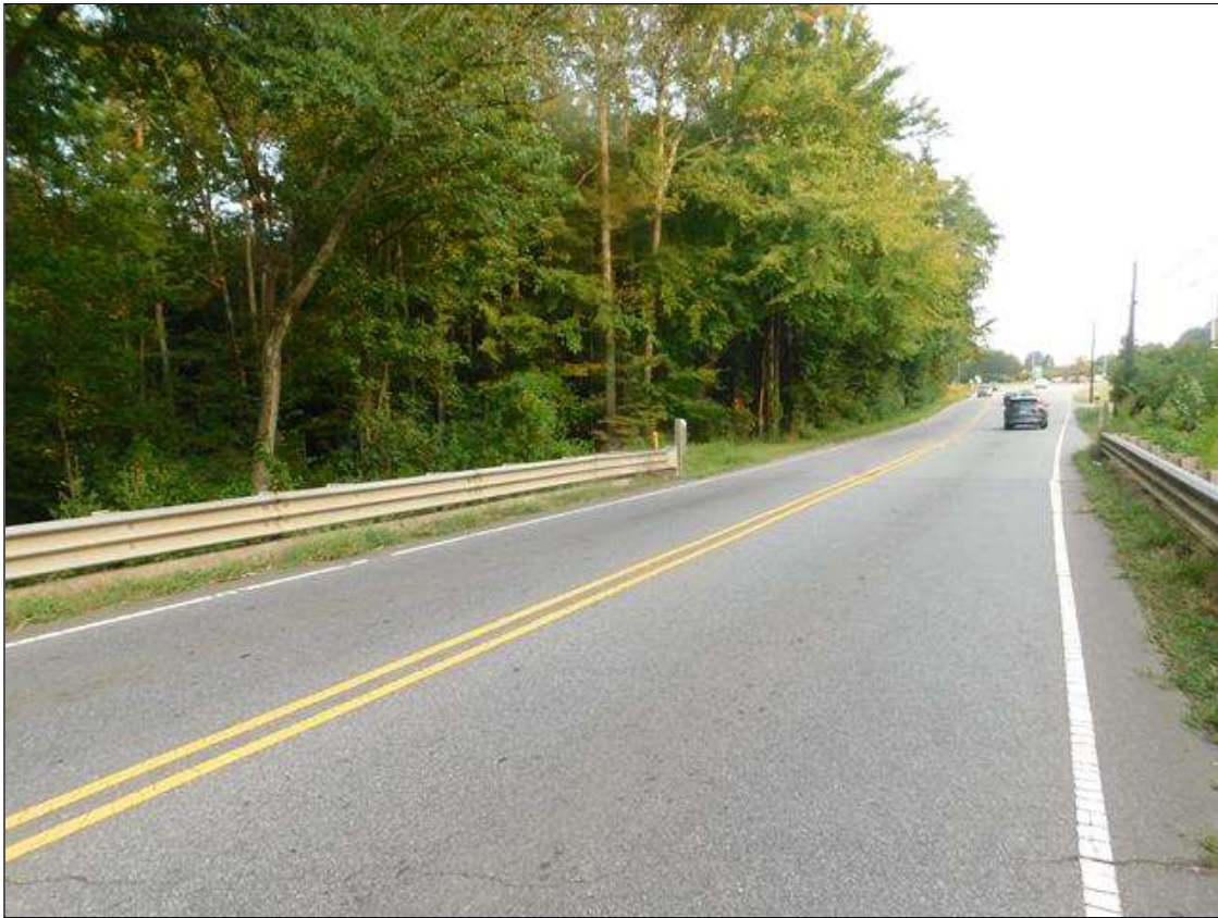
LOOKING NORTH FROM DECK
