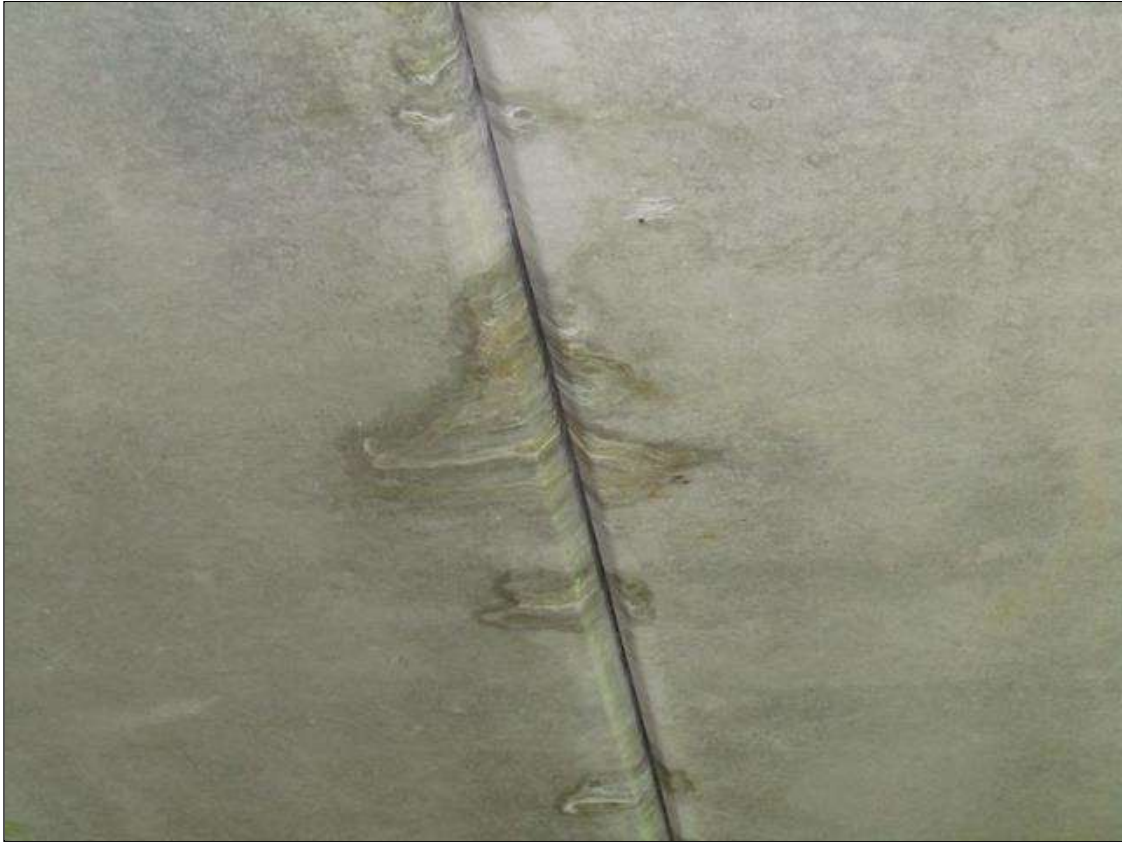
Span 2 Slab 11: EFFLO ON BOTTOM FROM BETWEEN SLABS
