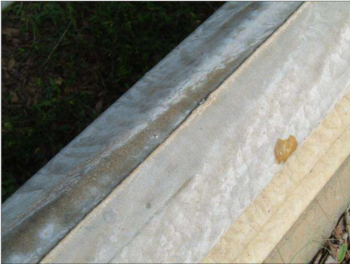
Span 3 Left Bridge Rail - Protective System: SUBSTANTIALLY EFFECTIVE ON TOP
