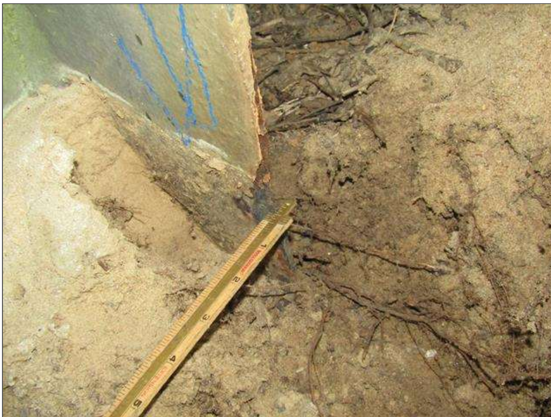
Bent 2 Pile 5: RUST SCALE ON BOTTOM OF NORTH FLANGE ON EAST SIDE UP 4" X 2" WIDE WITH 1/8" STEEL REMAINING ON 1/2" FLANGE/PAR
