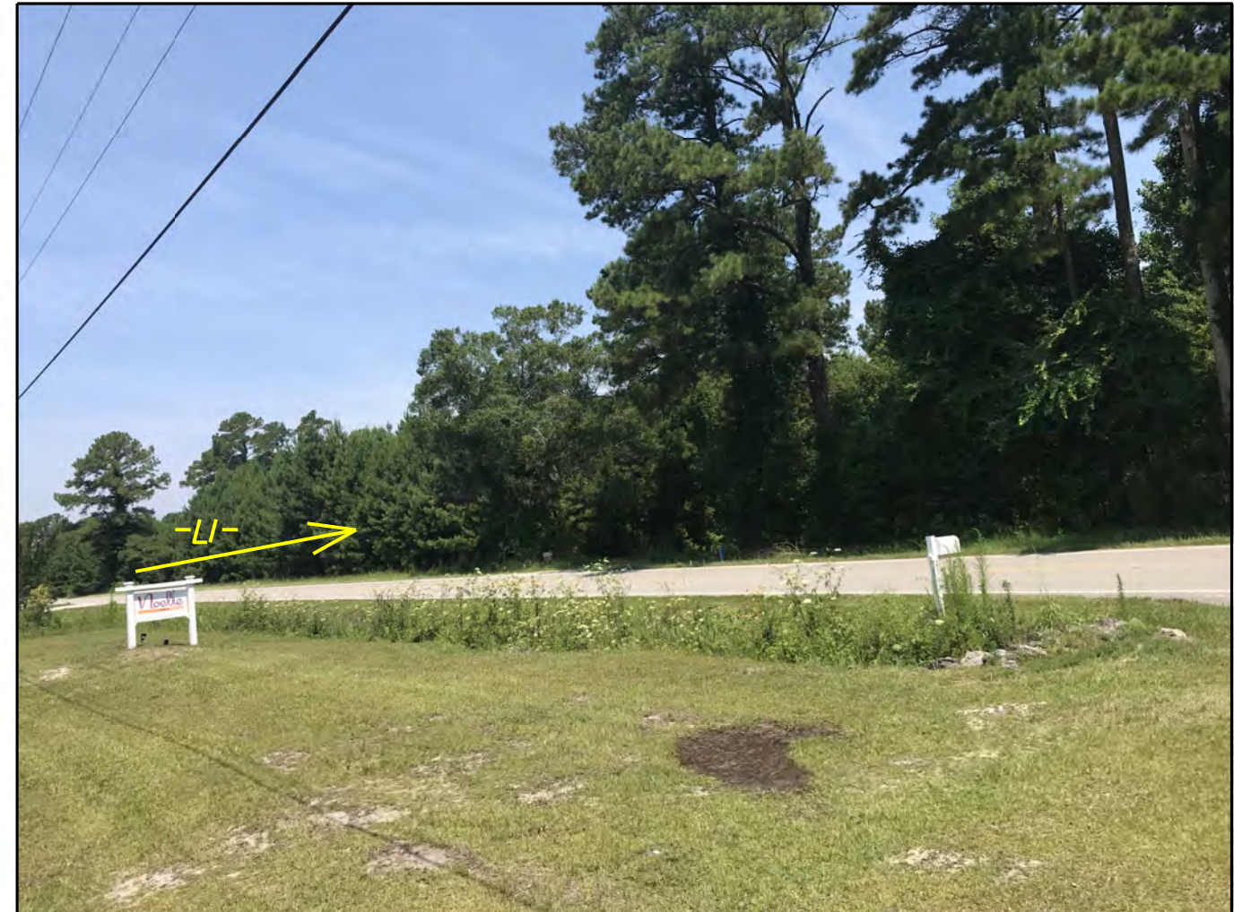
LOOKING AT BRIDGE NO.257 BENT 1 FROM RIGHT OF -Y30- CENTERLINE
