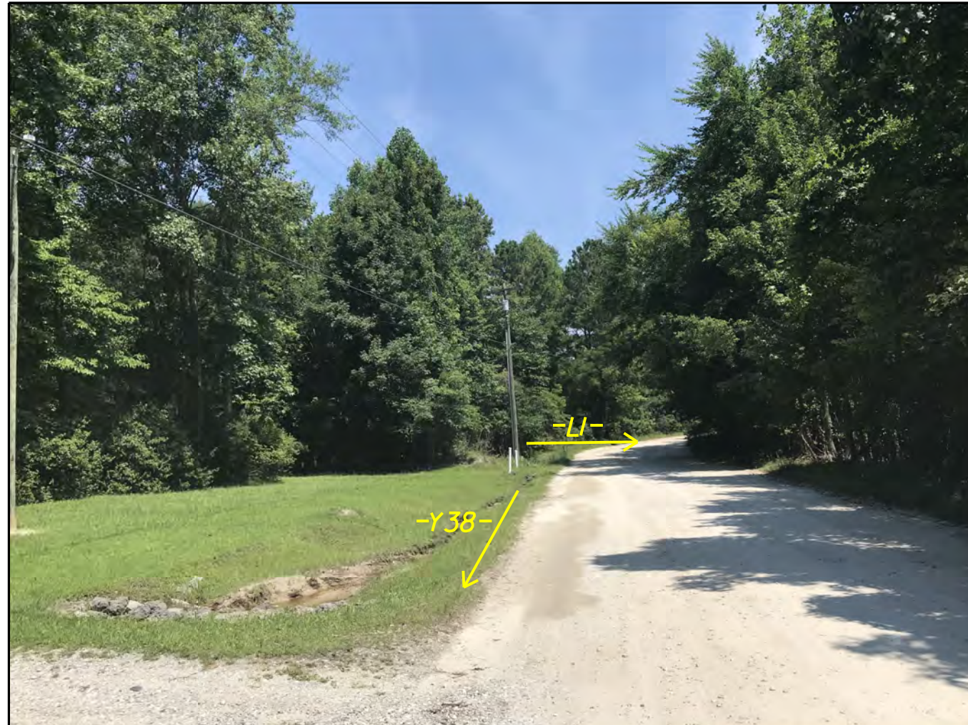
-Y38-, LOOKING DOWNSTATION FROM STATION 23+00
