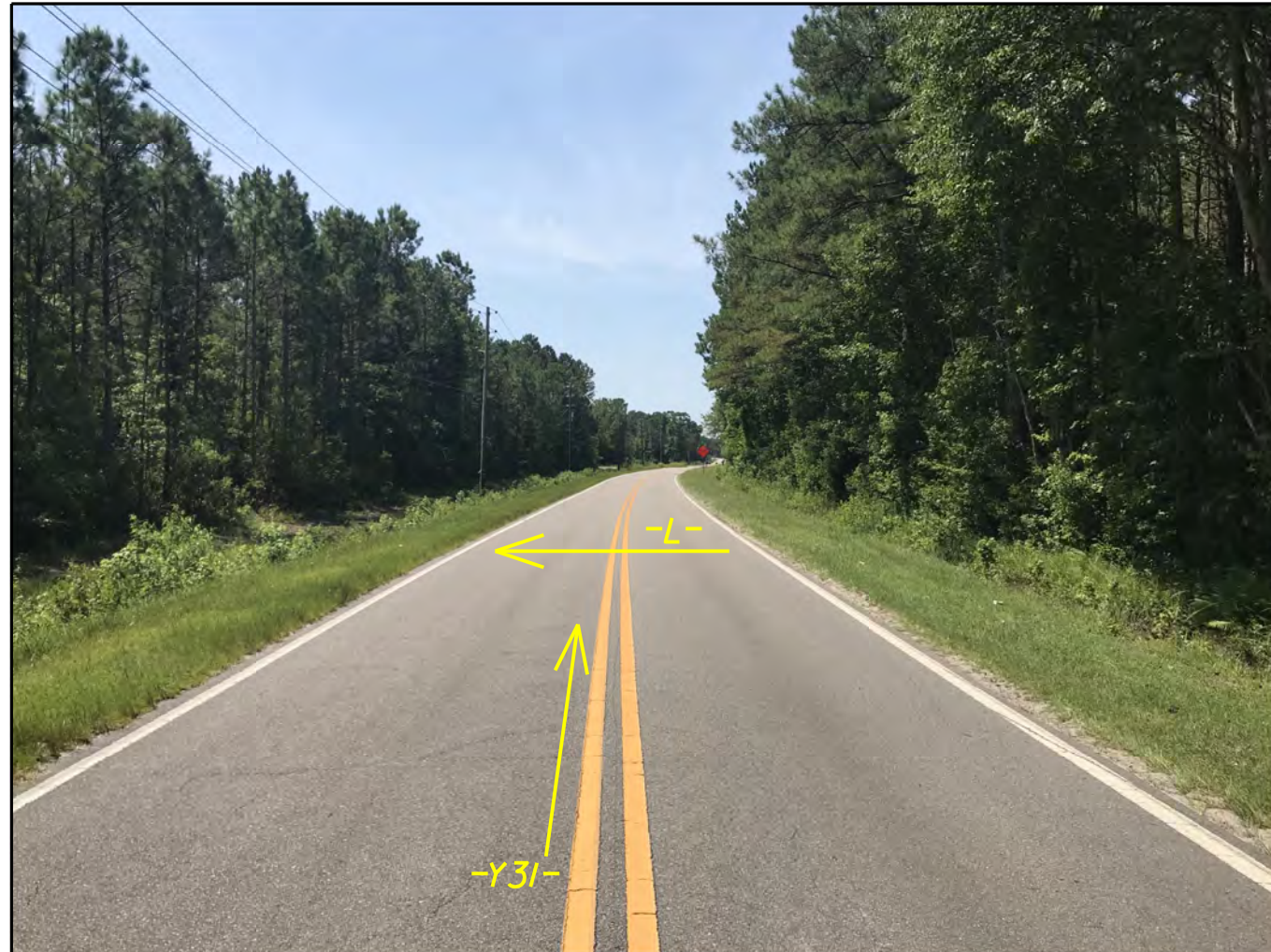
-Y31-, LOOKING UPSTATION FROM STATION 29+00
