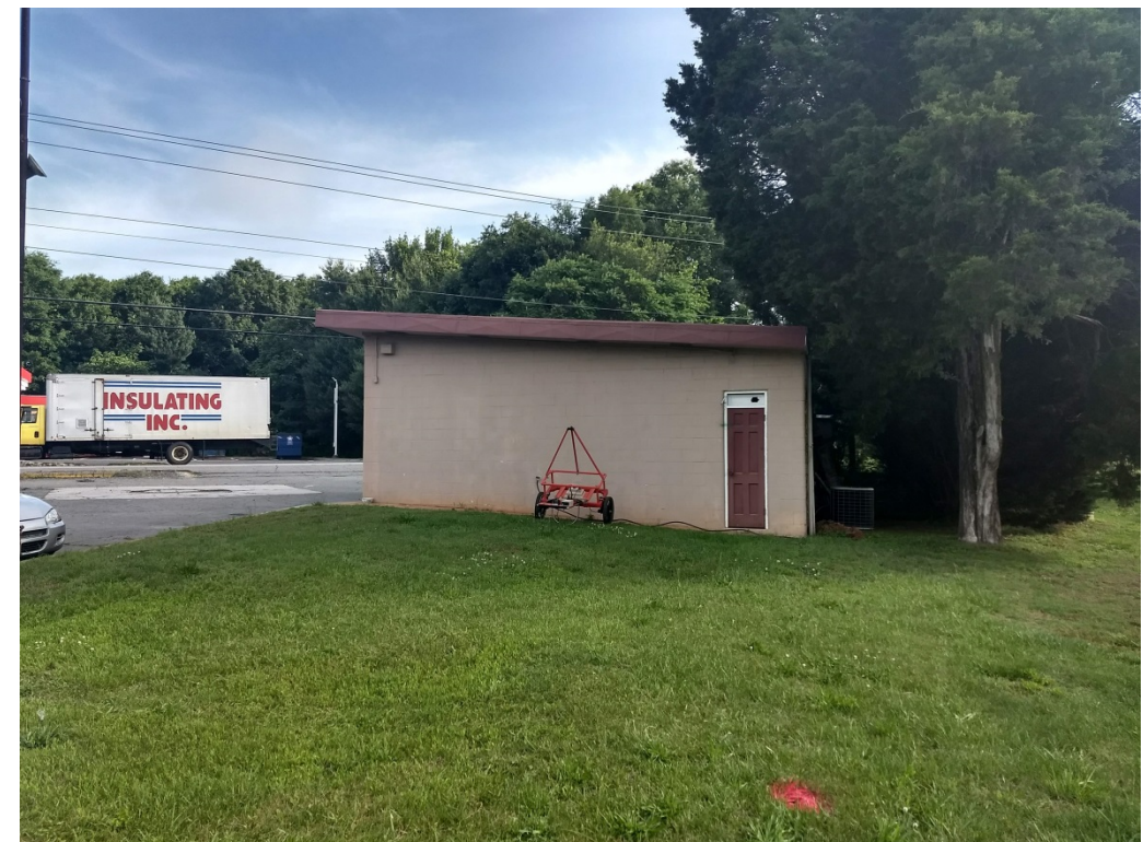
d. Photo from south side of site looking north.
