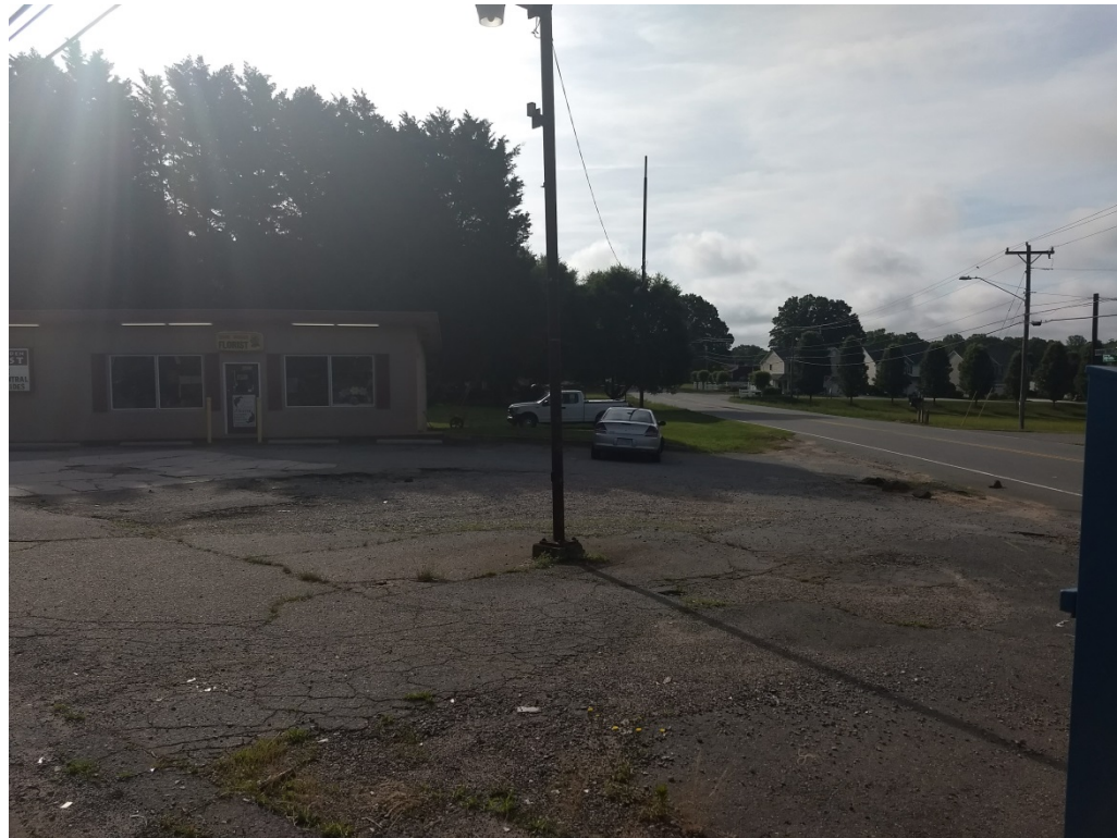
a. Photo from north side of site looking south.
