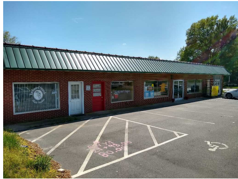
A. Photograph of front of Parcel 39 business and study area, facing southwest.
