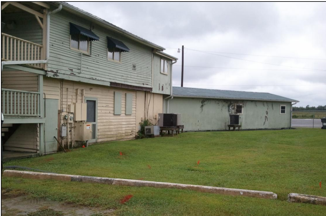
From northeastern portion of site looking southwest.
