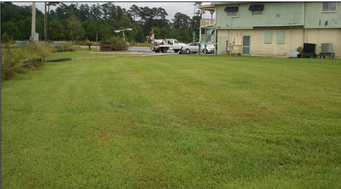
From northwestern portion of site looking east.
