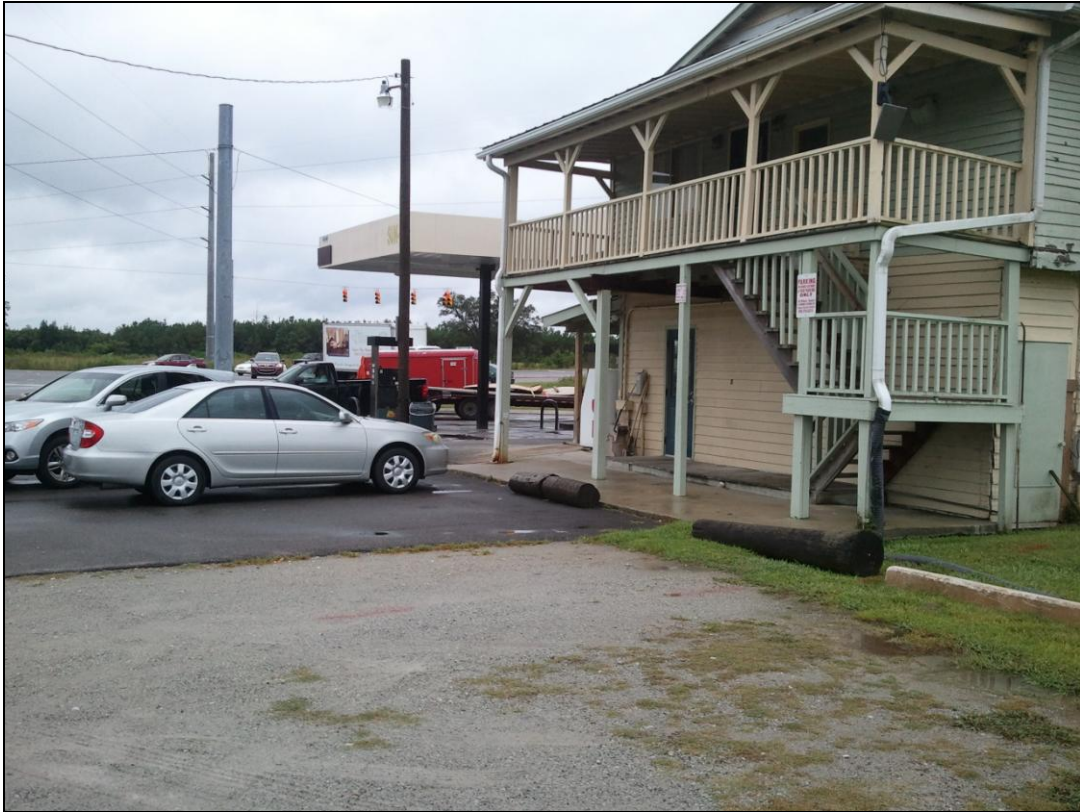
From northeastern portion of site looking south.
