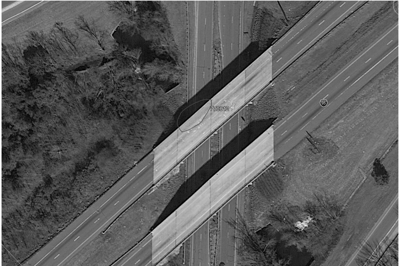
Figure 2: Beam 1 of Span 2 Location
