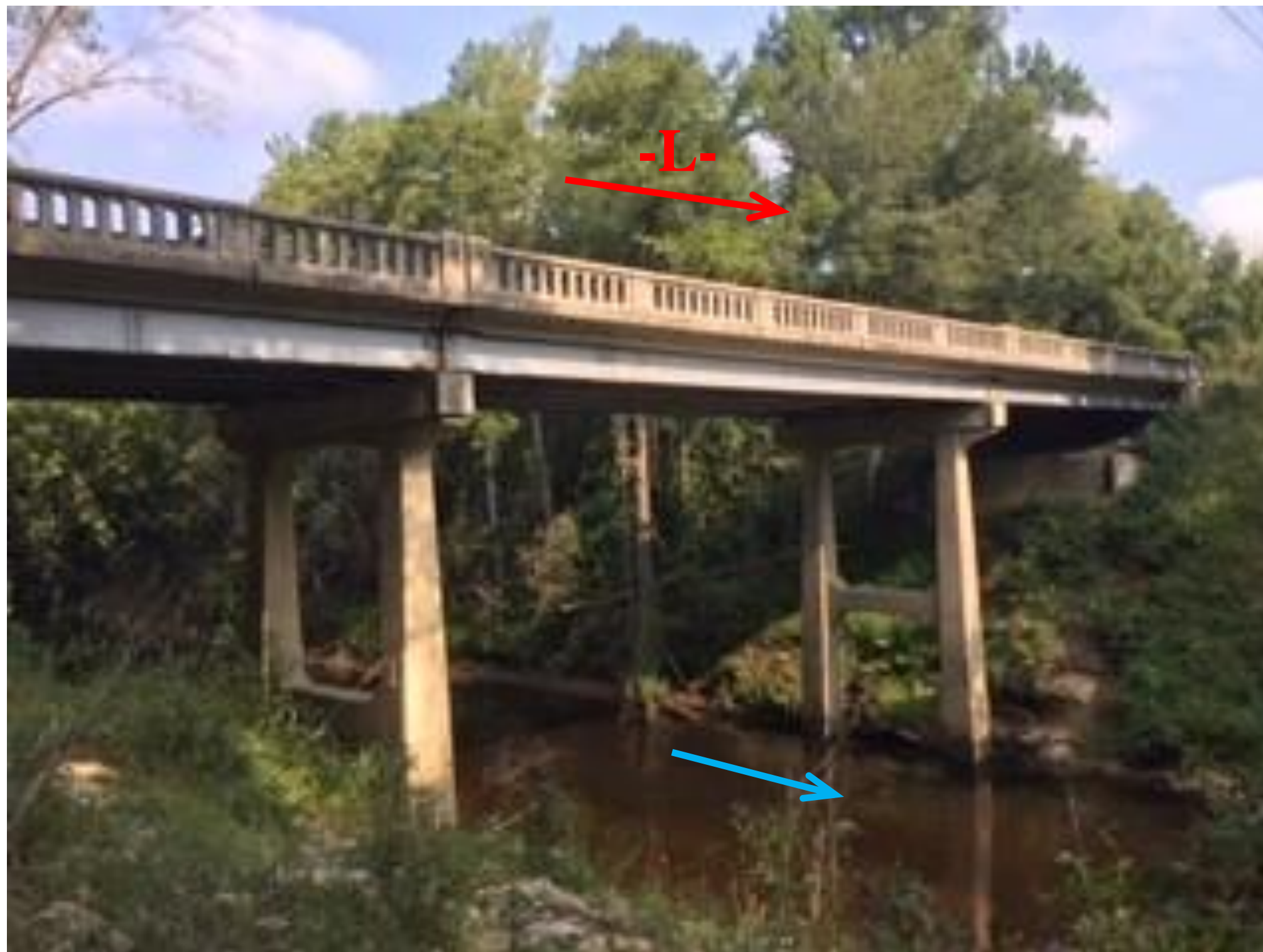
Looking North towards End Bent 2
