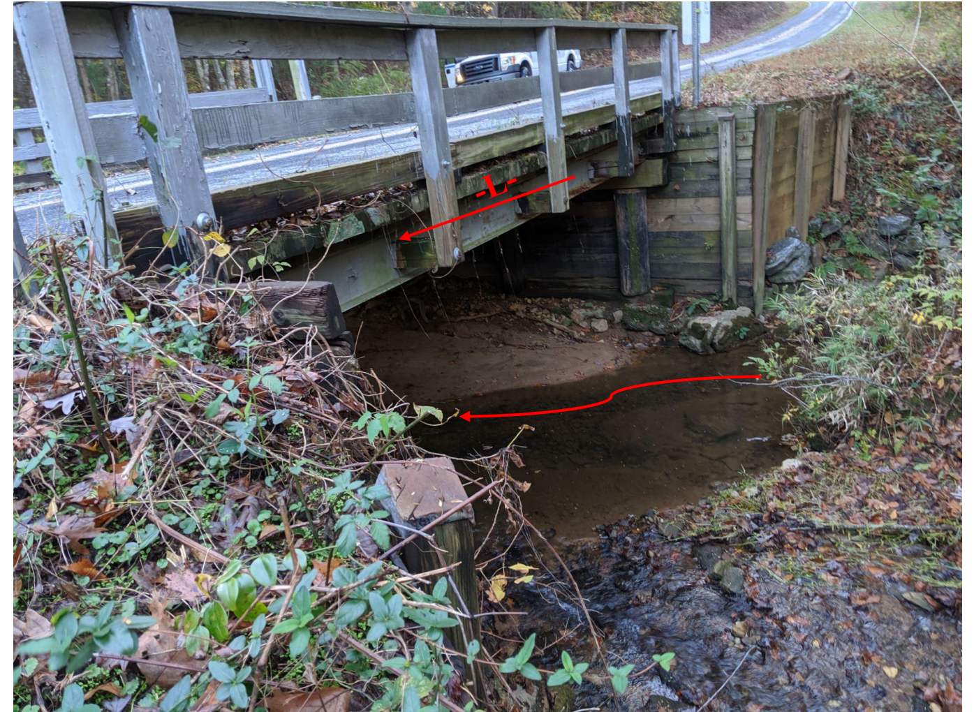
Photograph No. 2: Looking Downstream
