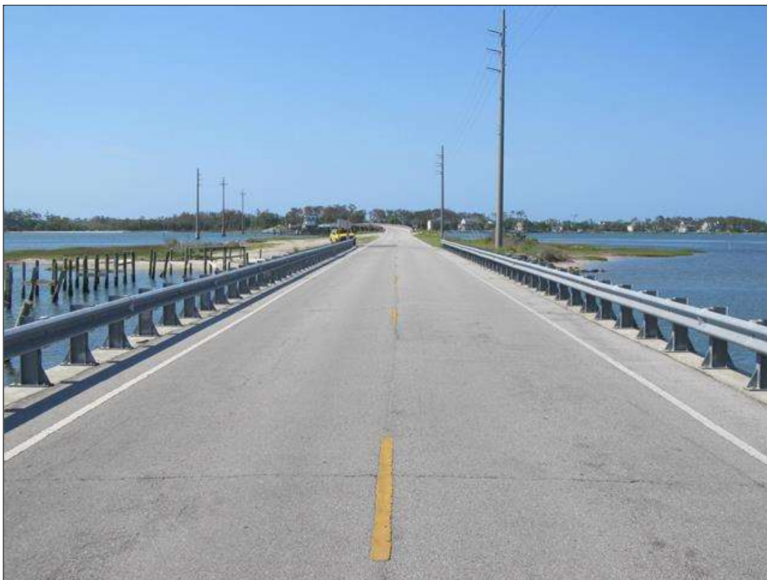
LOOKING SOUTH OFF STRUCTURE.
