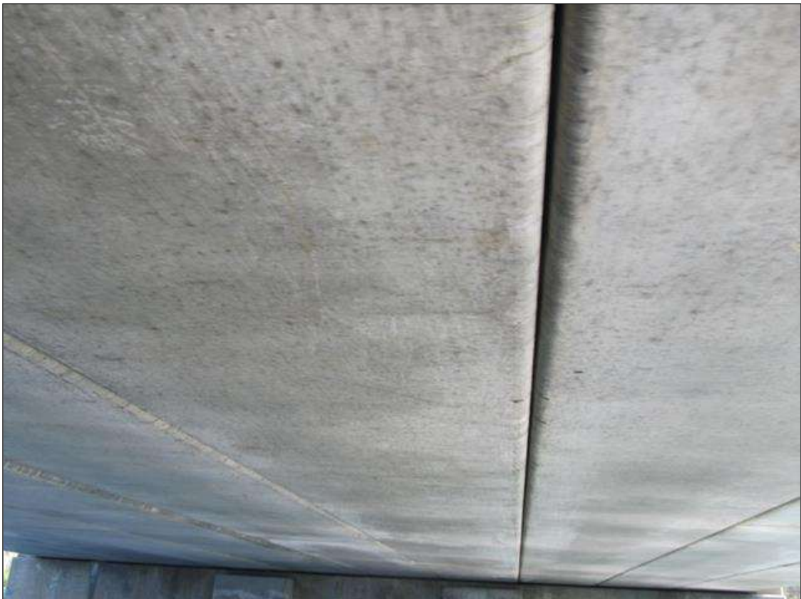
SPAN UNDERSIDE. SIMILAR IN ALL SPANS.
