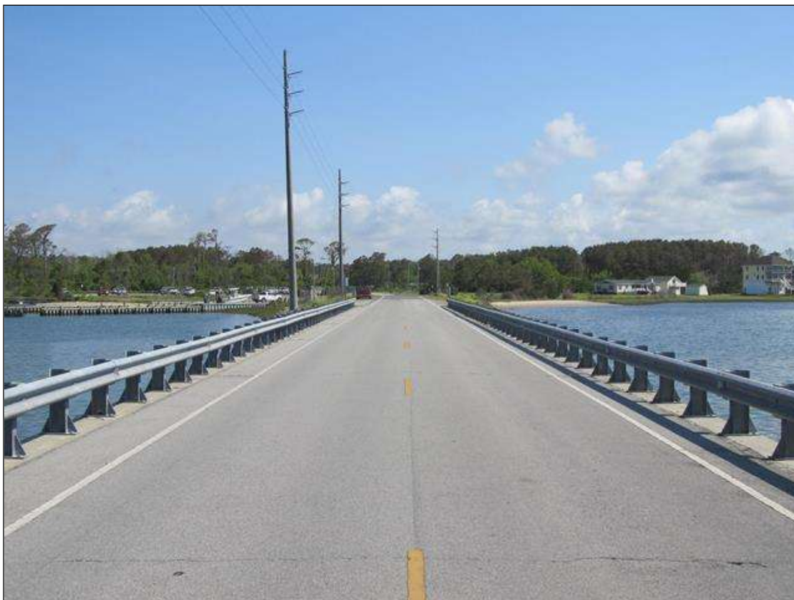
LOOKING NORTH OFF STRUCTURE.
