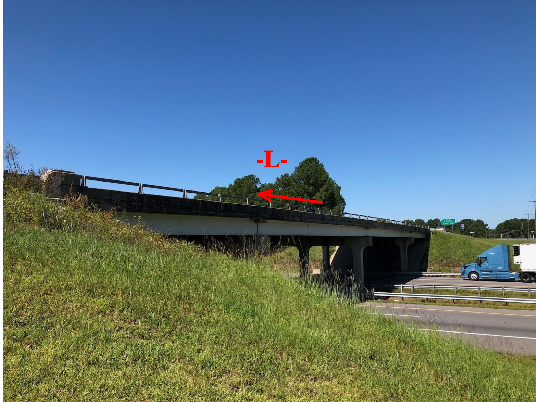
Looking Southwest towards End Bent 1
