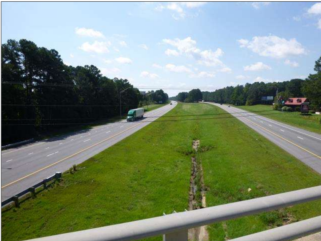
ROADWAY VIEW FROM BRIDGE DECK, LOOKING SOUTH
