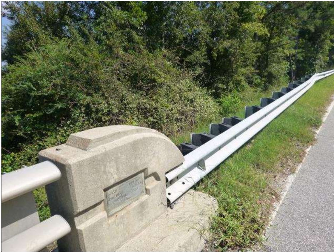
NORTHEAST GUARDRAIL ATTACHMENT
