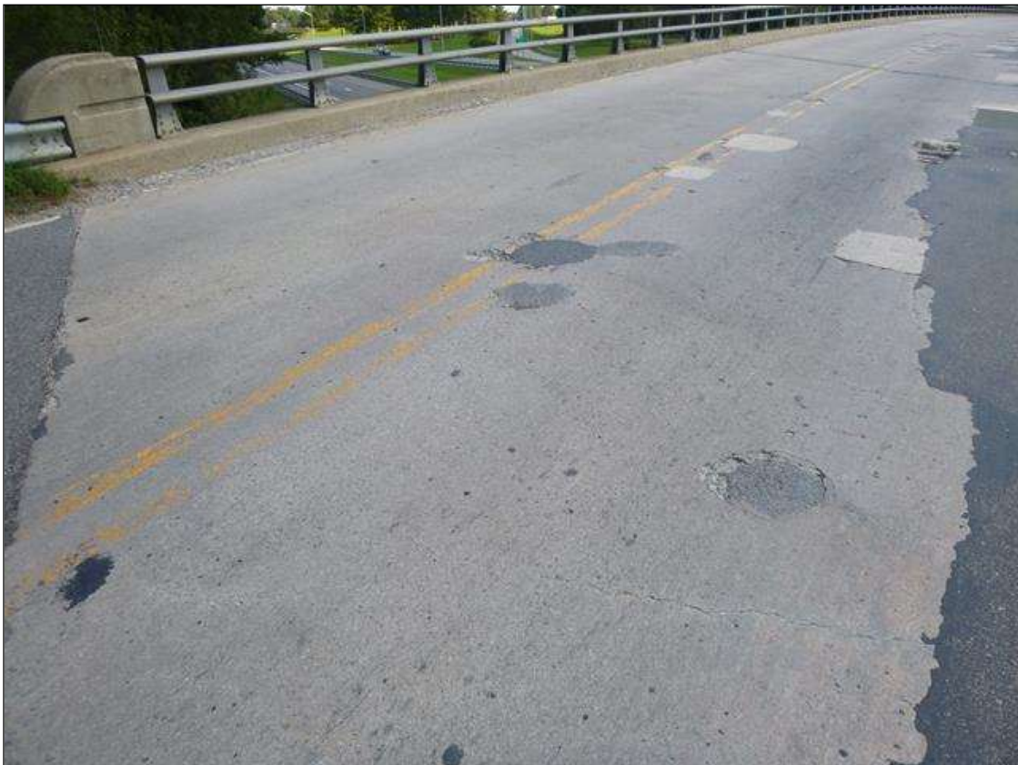
CONCRETE BRIDGE DECK, SPAN 1, LOOKING EAST
