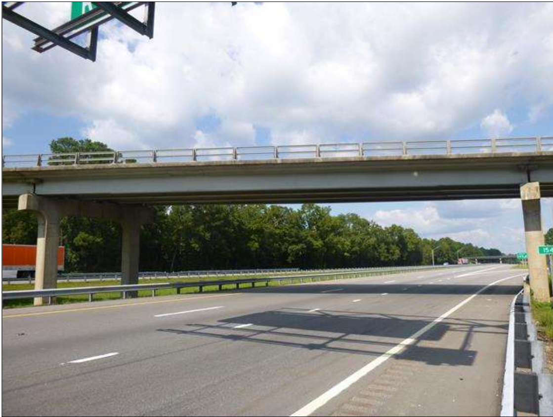
SPAN 4 CLEARANCE, LOOKING NORTH
