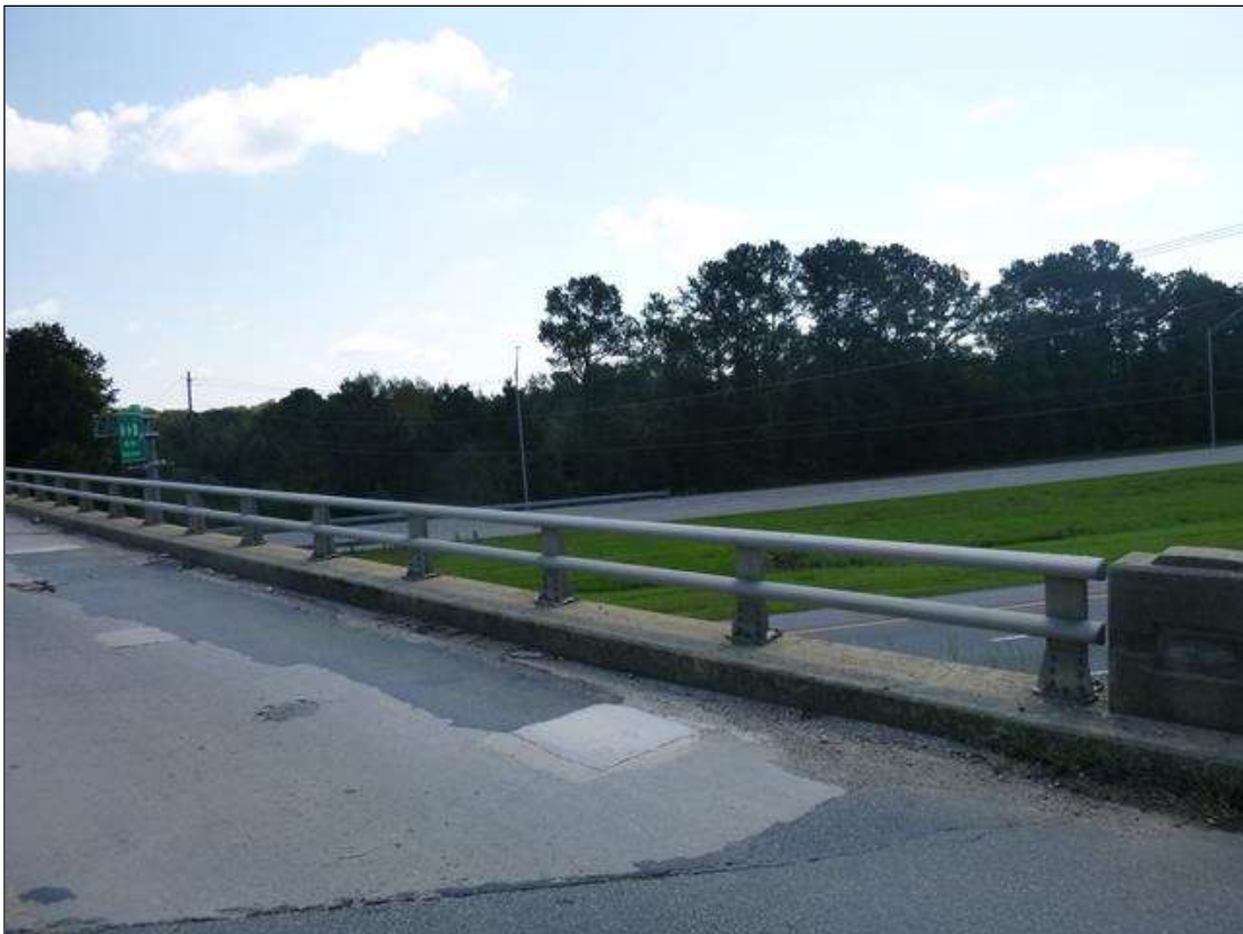
SOUTH BRIDGE RAIL
