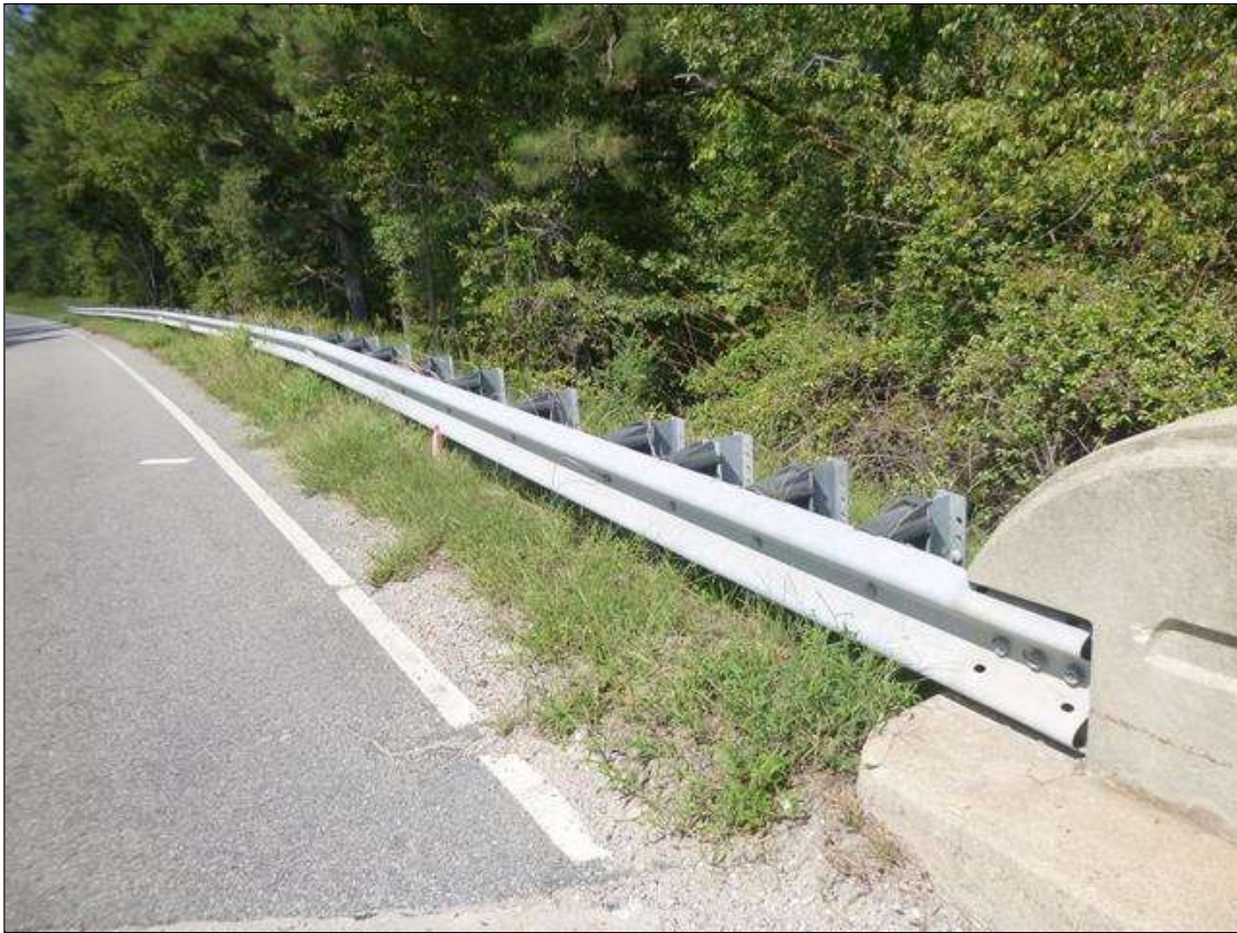
NORTHWEST GUARDRAIL ATTACHMENT
