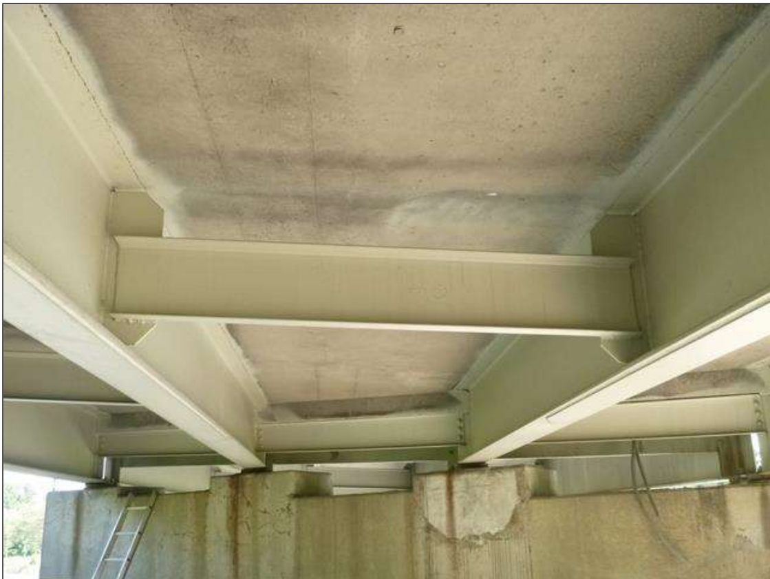
INTERMEDIATE DIAPHRAGM, SPAN 1, AT 1/2 POINT, LOOKING EAST
