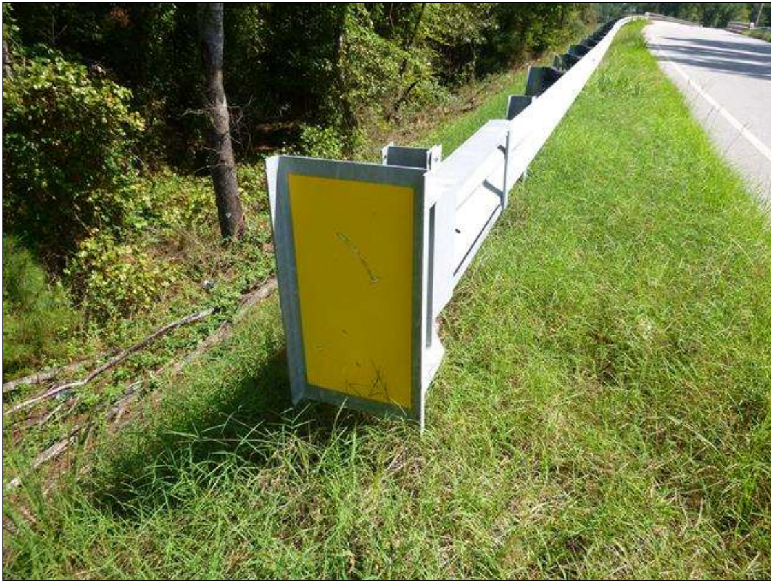
NORTHWEST GUARDRAIL TERMINAL
