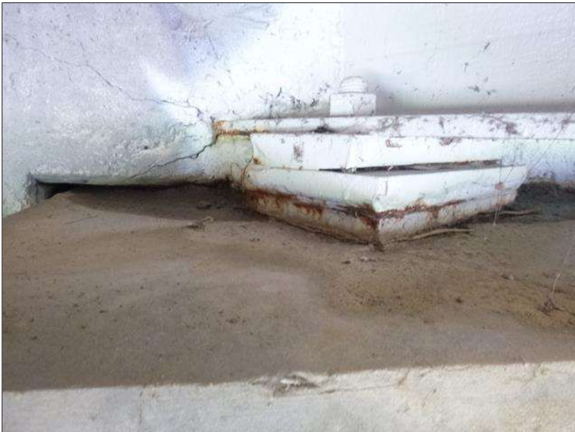
BEARING ASSEMBLY, END BENT 1, BEAM 2, LOOKING WEST
