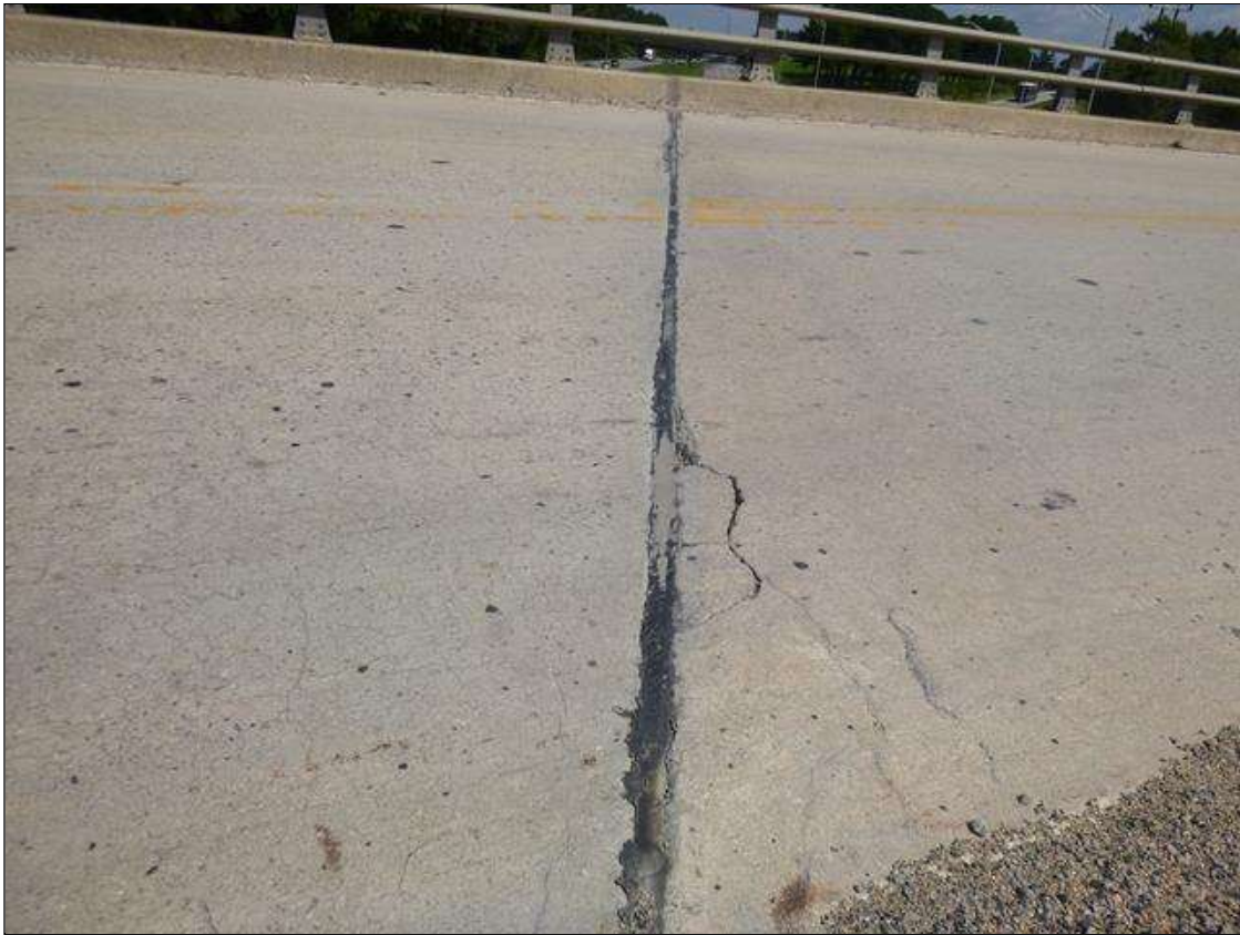
JOINT OVER BENT 3, LOOKING NORTH
