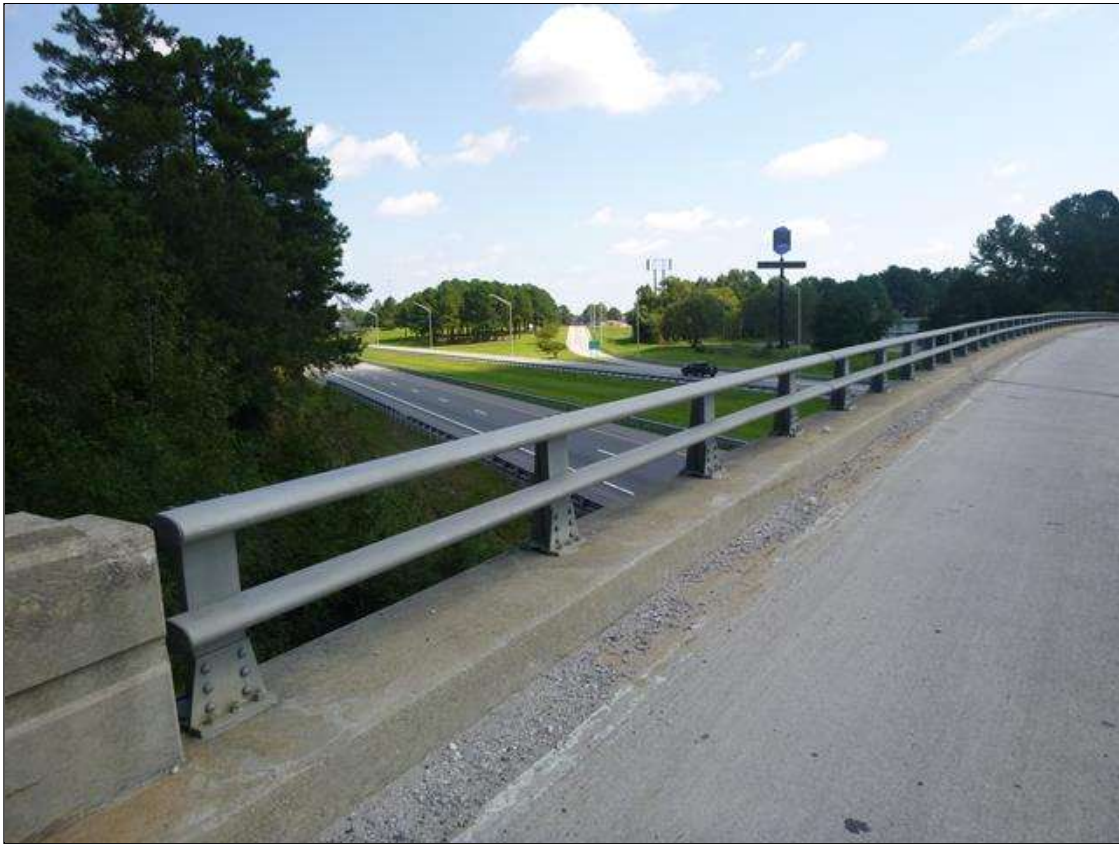
NORTH BRIDGE RAIL
