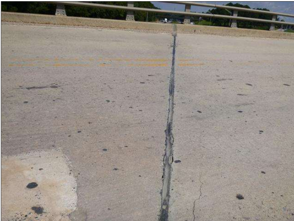
JOINT OVER BENT 2, LOOKING NORTH
