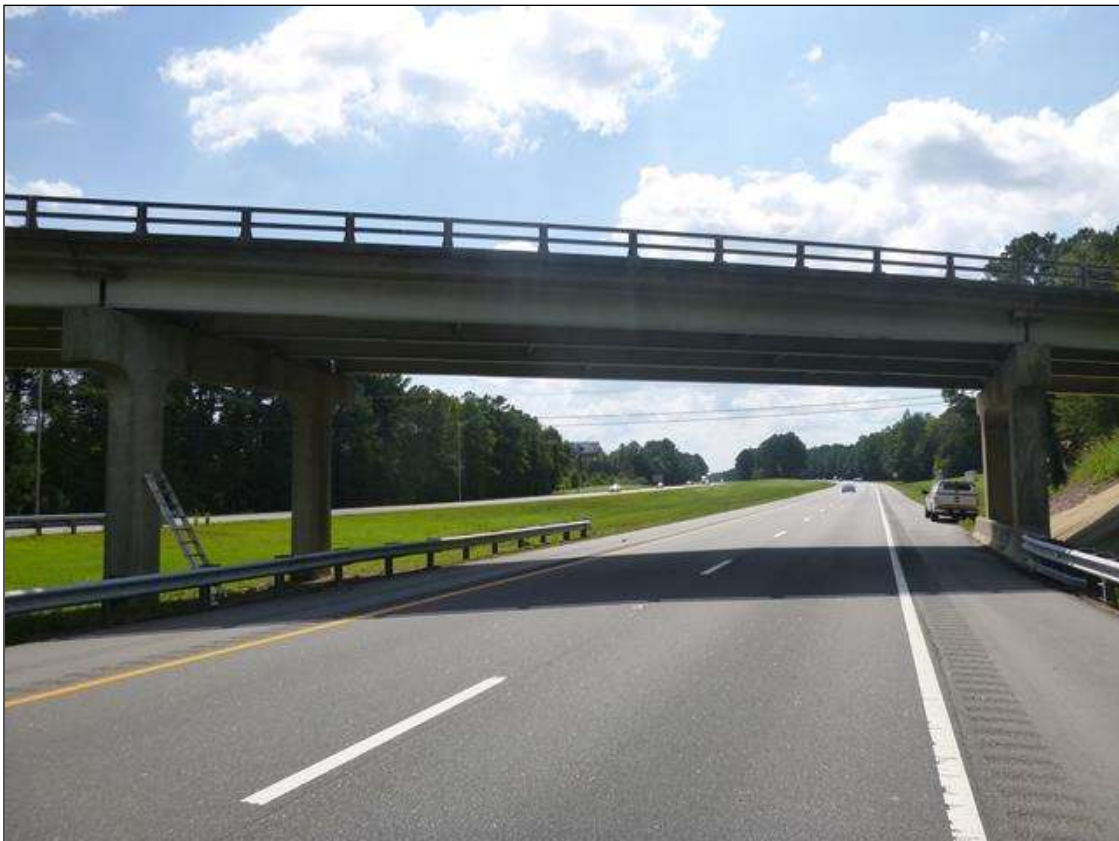
SPAN 2 CLEARANCE, LOOKING SOUTH
