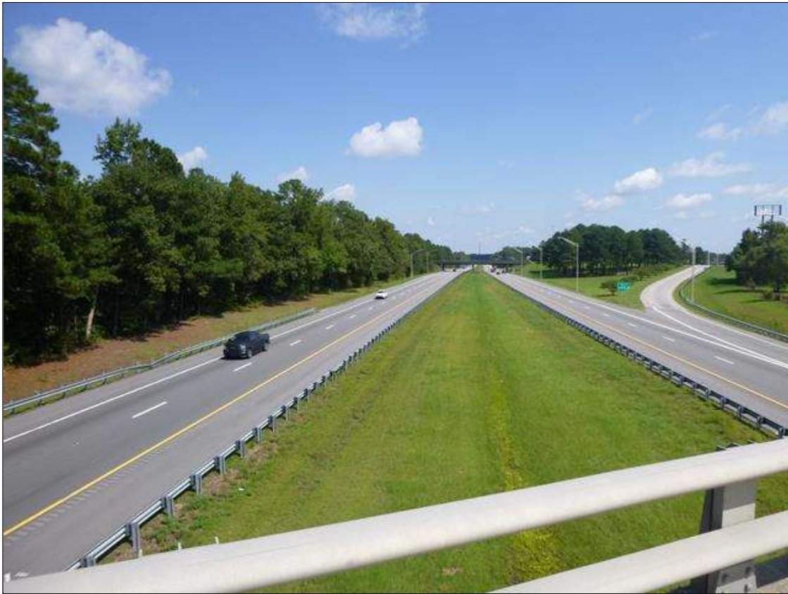
ROADWAY VIEW FROM BRIDGE DECK, LOOKING NORTH
