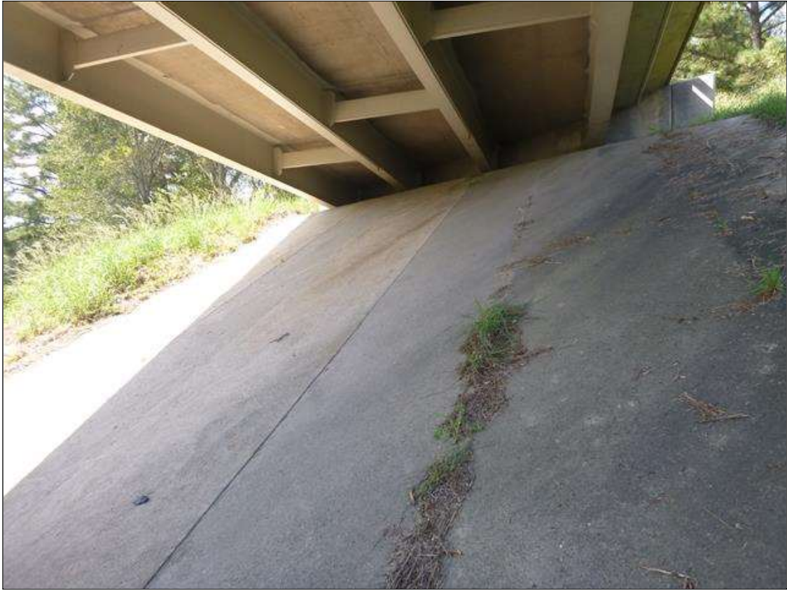
END BENT 1 SLOPE PROTECTION, LOOKING WEST
