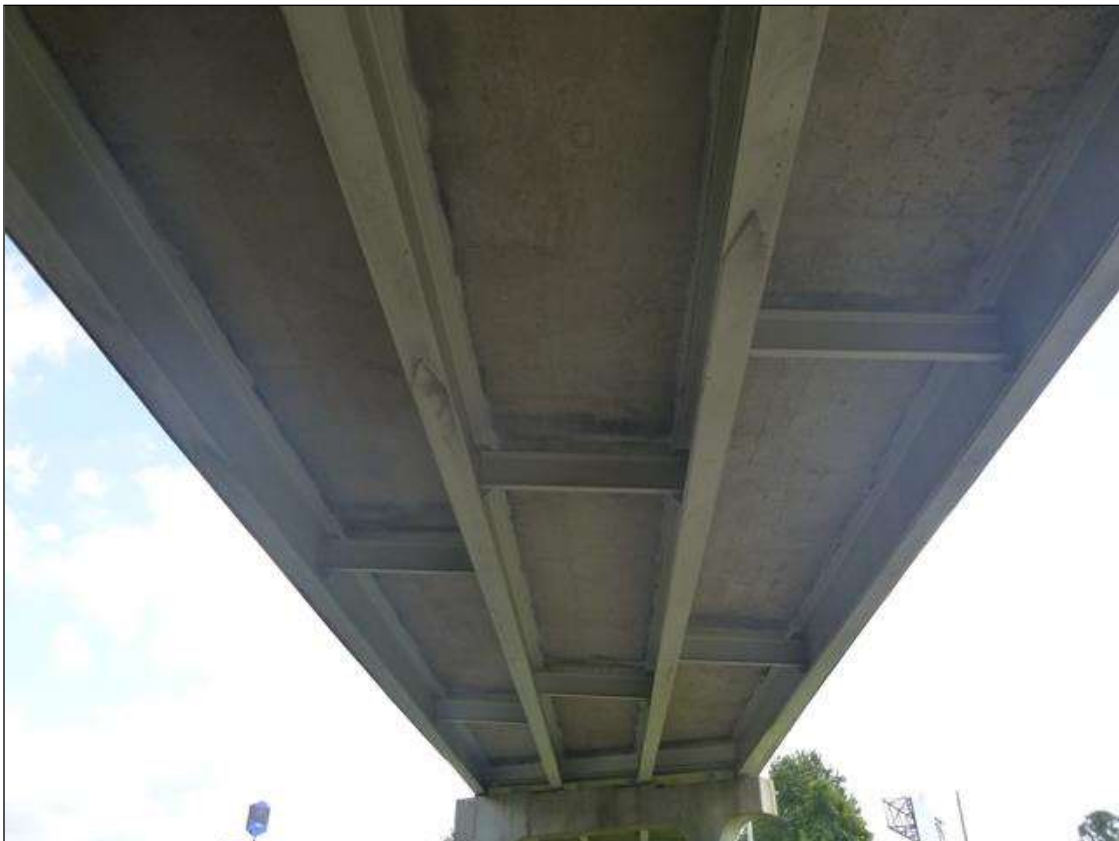
SUPERSTRUCTURE UNDERSIDE, SPAN 2, LOOKING EAST
