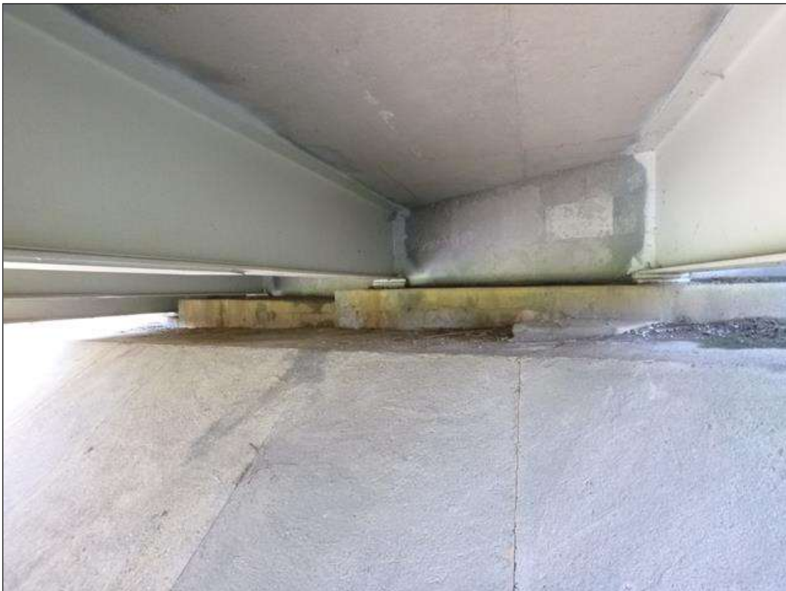
END BENT 1 ELEVATION, LOOKING WEST
