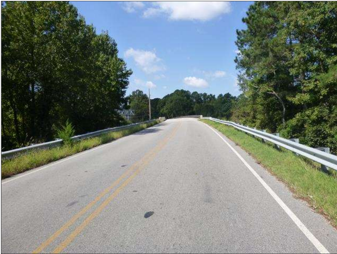
EAST APPROACH, LOOKING WEST
