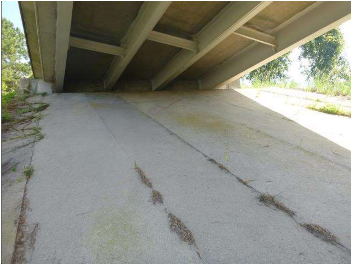
END BENT 2 SLOPE PROTECTION, LOOKING EAST
