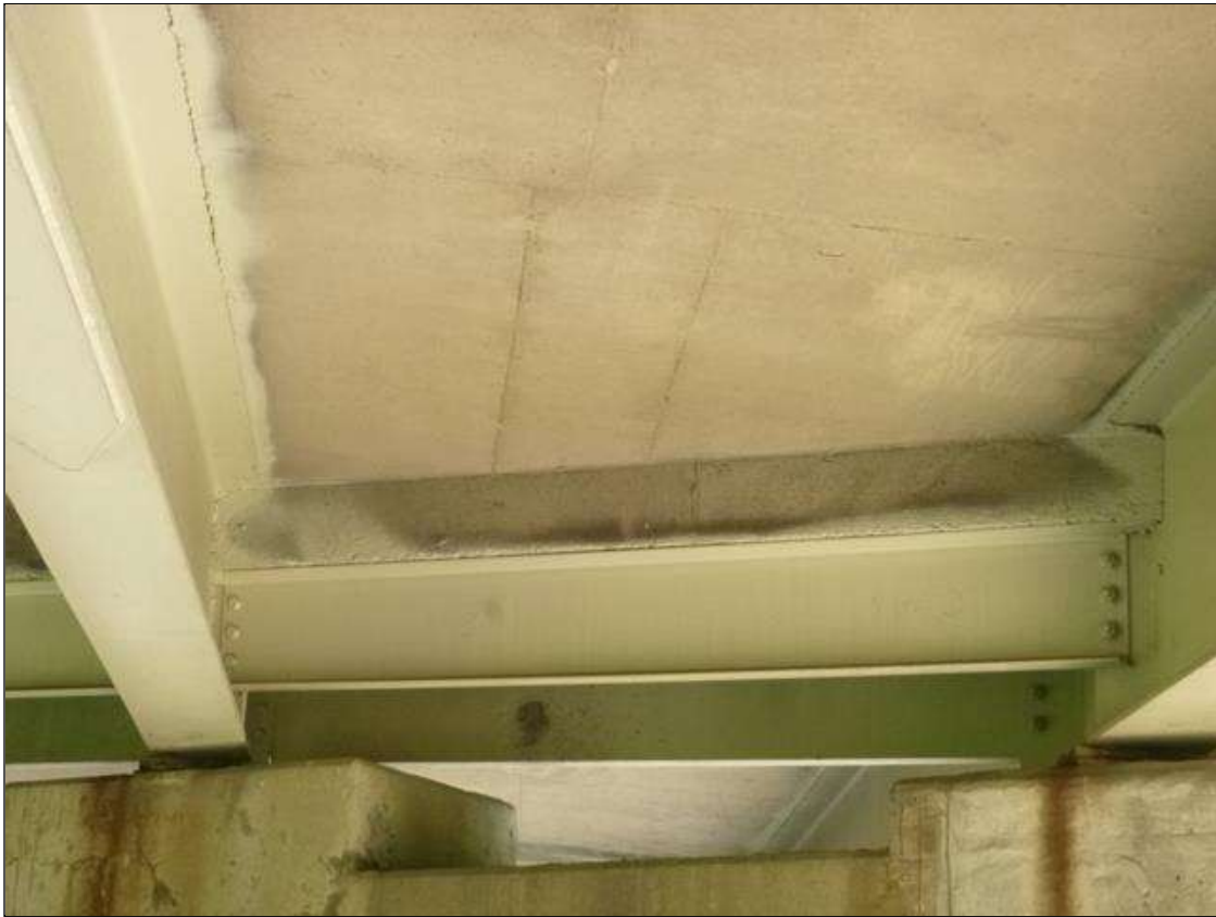
END DIAPHRAGM, BENT 1, BAY 2, LOOKING EAST
