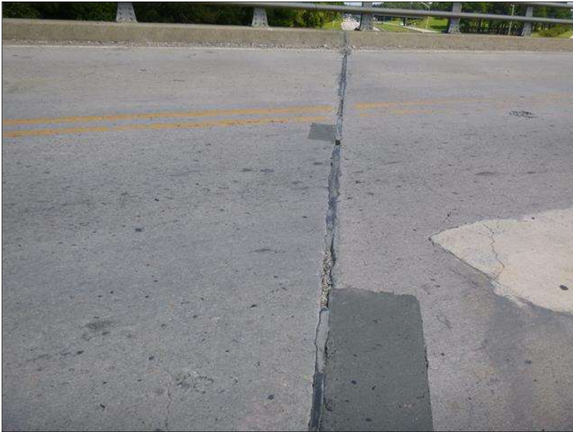
JOINT OVER BENT 1, LOOKING NORTH
