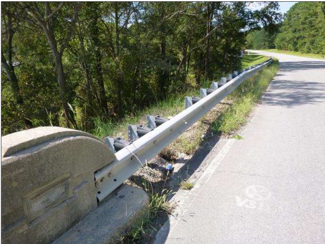
SOUTHWEST GUARDRAIL ATTACHMENT
