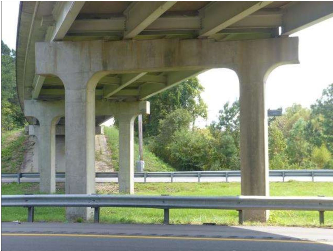
BENT 2 ELEVATION, LOOKING EAST
