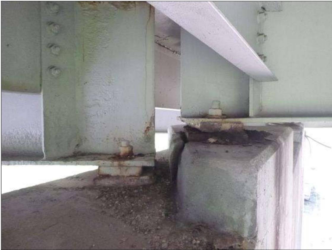
BEARING ASSEMBLY OVER BENT 1, BEAM 2, LOOKING SOUTH
