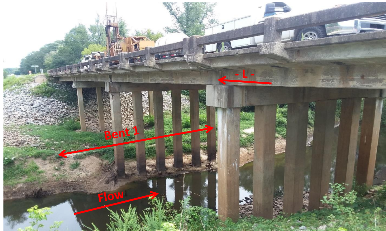
Photograph No. 1: View from West Side of Bridge looking North
