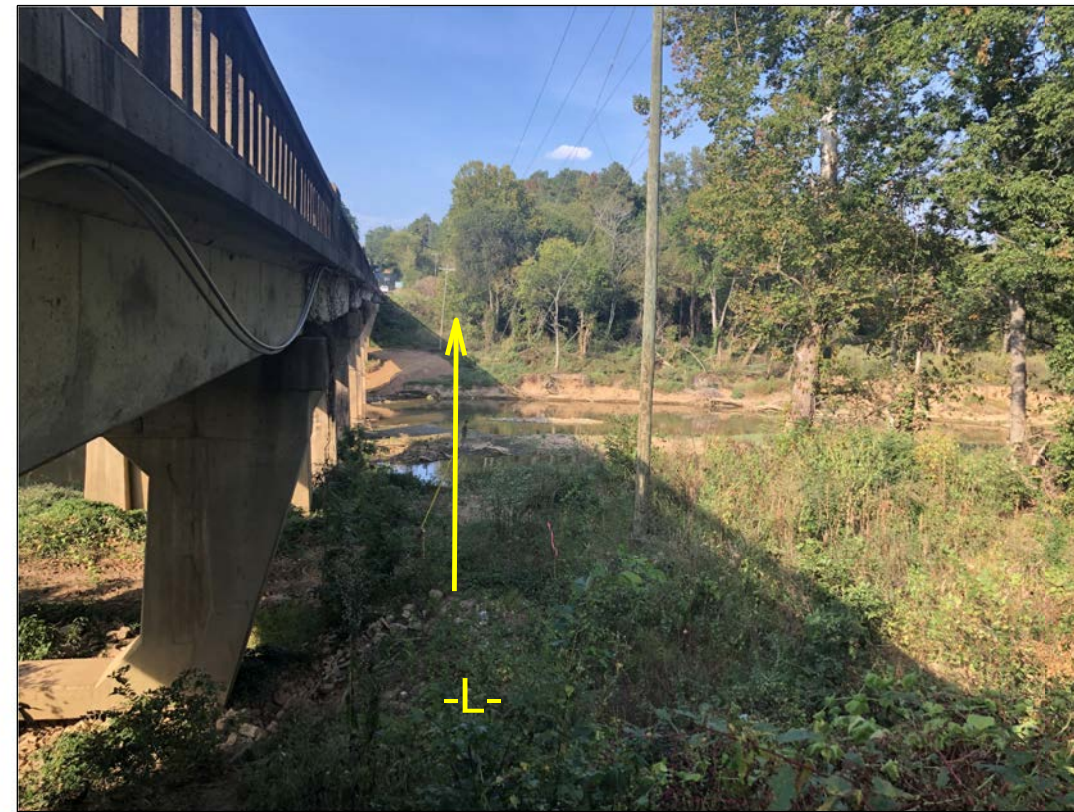
PHOTO 2: VIEW NEAR BENT 1, FACING UPSTATION.
