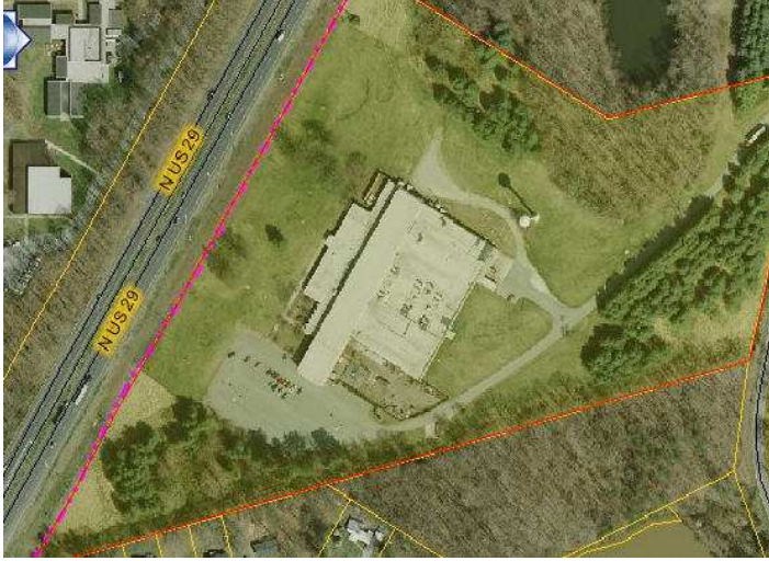
Site # 7: Wysong & Miles. Photo take from the Guilford Co GIS.
