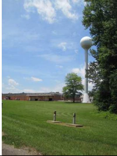
Site # 7: Wysong & Miles. View looking west from back side of property.
