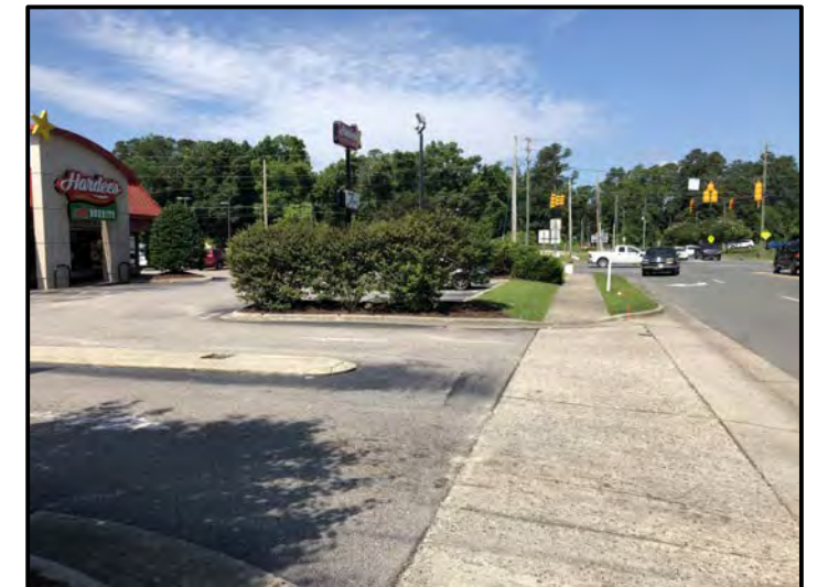
View of Survey Area (Facing Approximately West)
