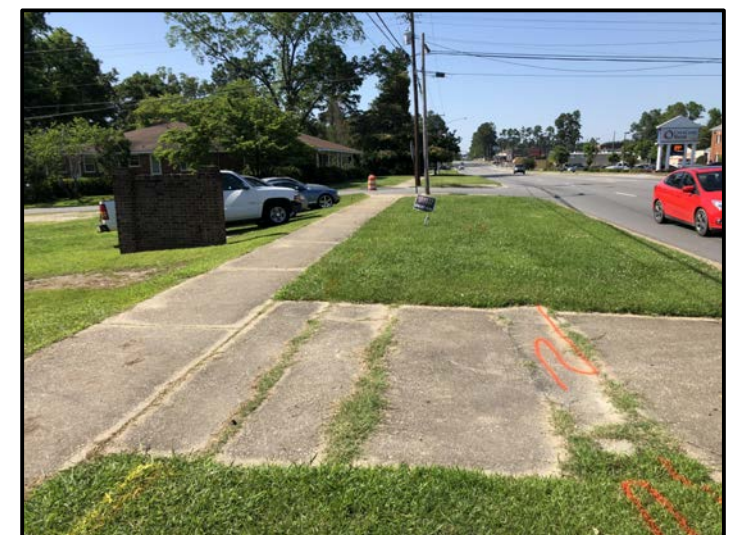
View of Survey Area (Facing Approximately North)
