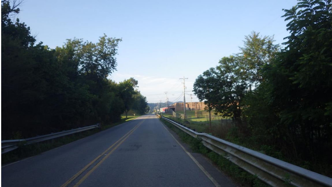
View on NC 141 looking to the South (red brick building is site #3, superfund site).
