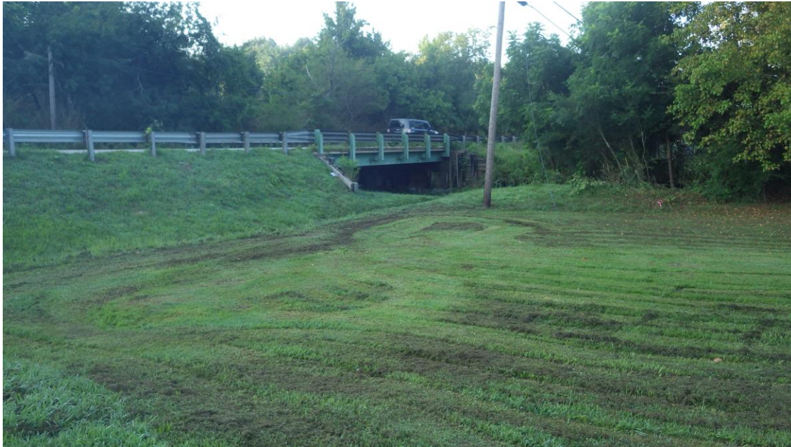
View of the downstream of the bridge.
