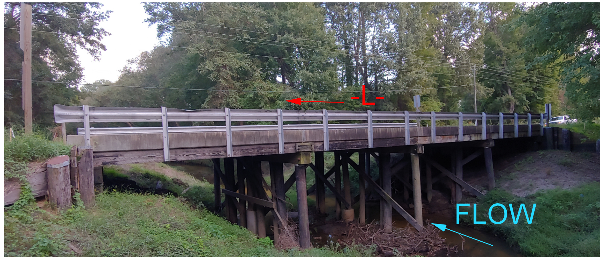
END BENT 2 LOOKING DOWNSTREAM
