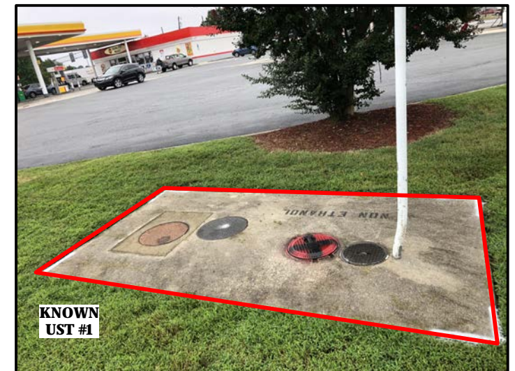
View of One Known UST Facing Approximately East
