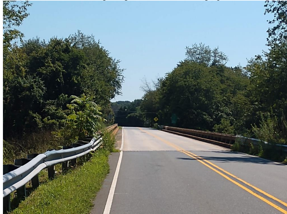
View of Existing Bridge No. 10 – -L- Looking Upstation
