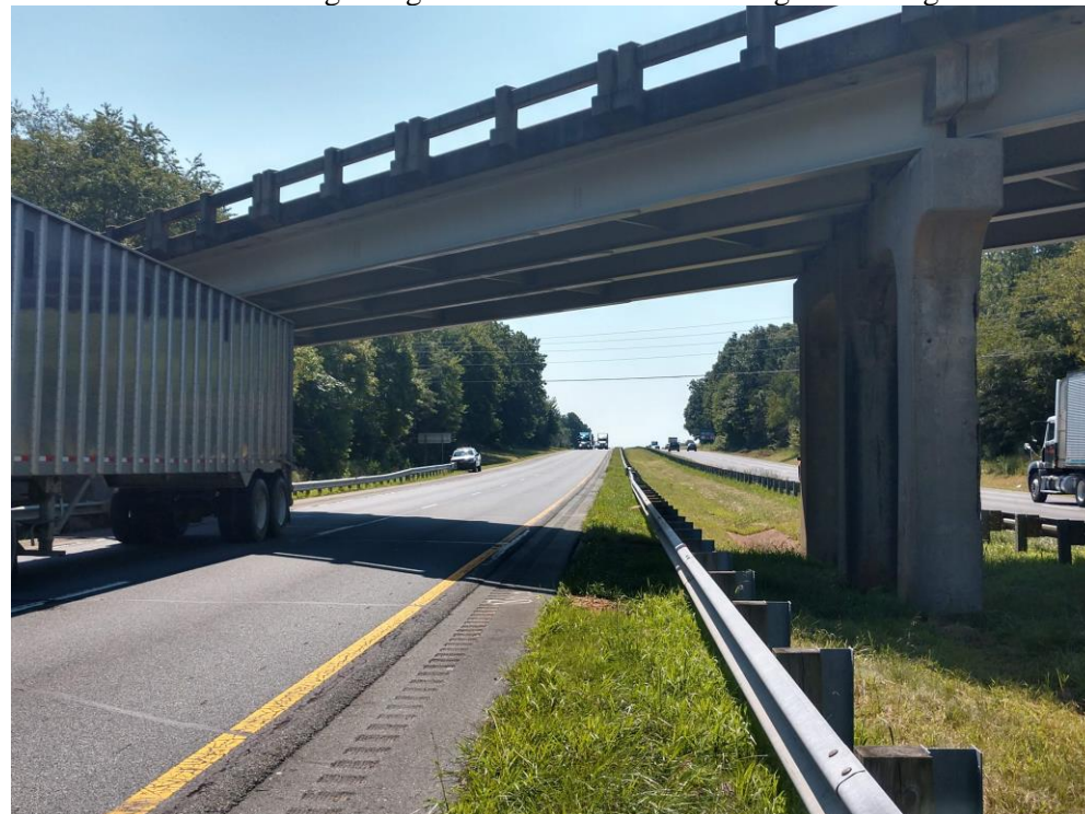
View of Existing Bridge No. 10 – Bent 1 – Looking Left to Right
