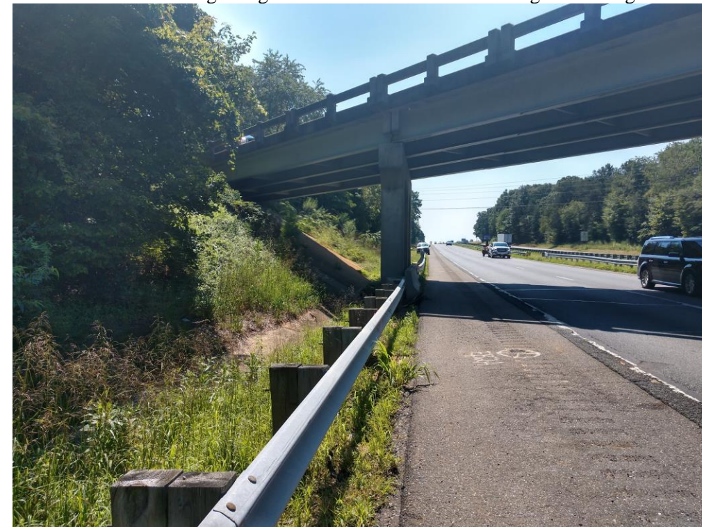
View of Existing Bridge No. 10 – End Bent 2 – Looking Left to Right
