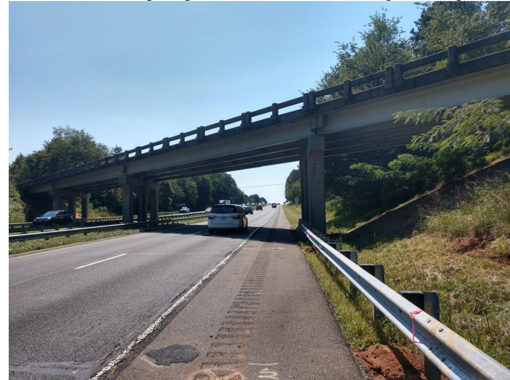
View of Existing Bridge No. 10 – End Bent 1 – Looking Left to Right
