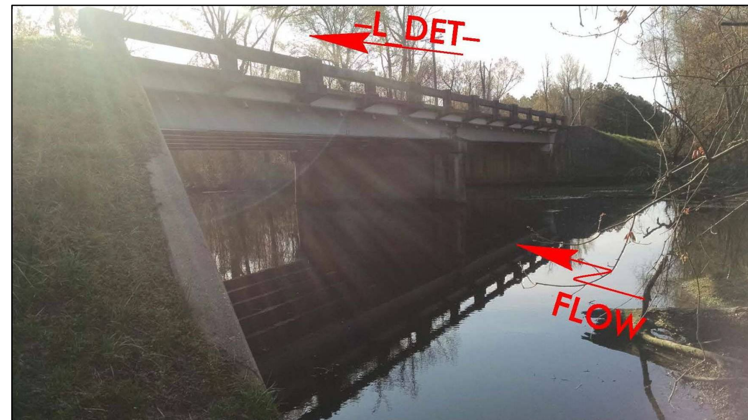
BRIDGE NO. 36 DETOUR OVER MAXWELL CREEK
