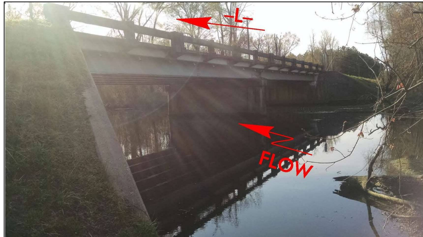
BRIDGE NO. 36 ON US 11 OVER MAXWELL CREEK
