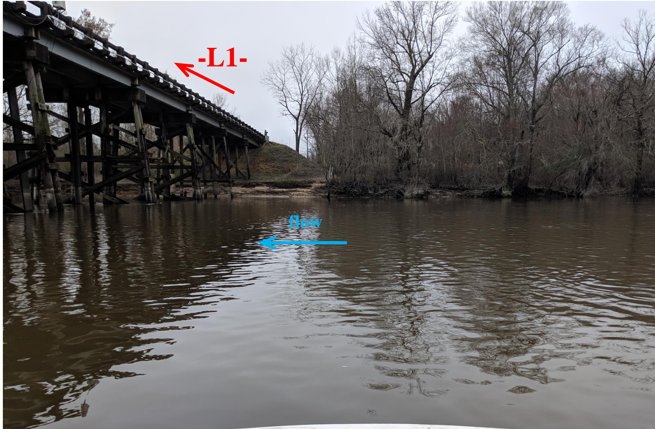
Looking Southwest towards End Bent 1
