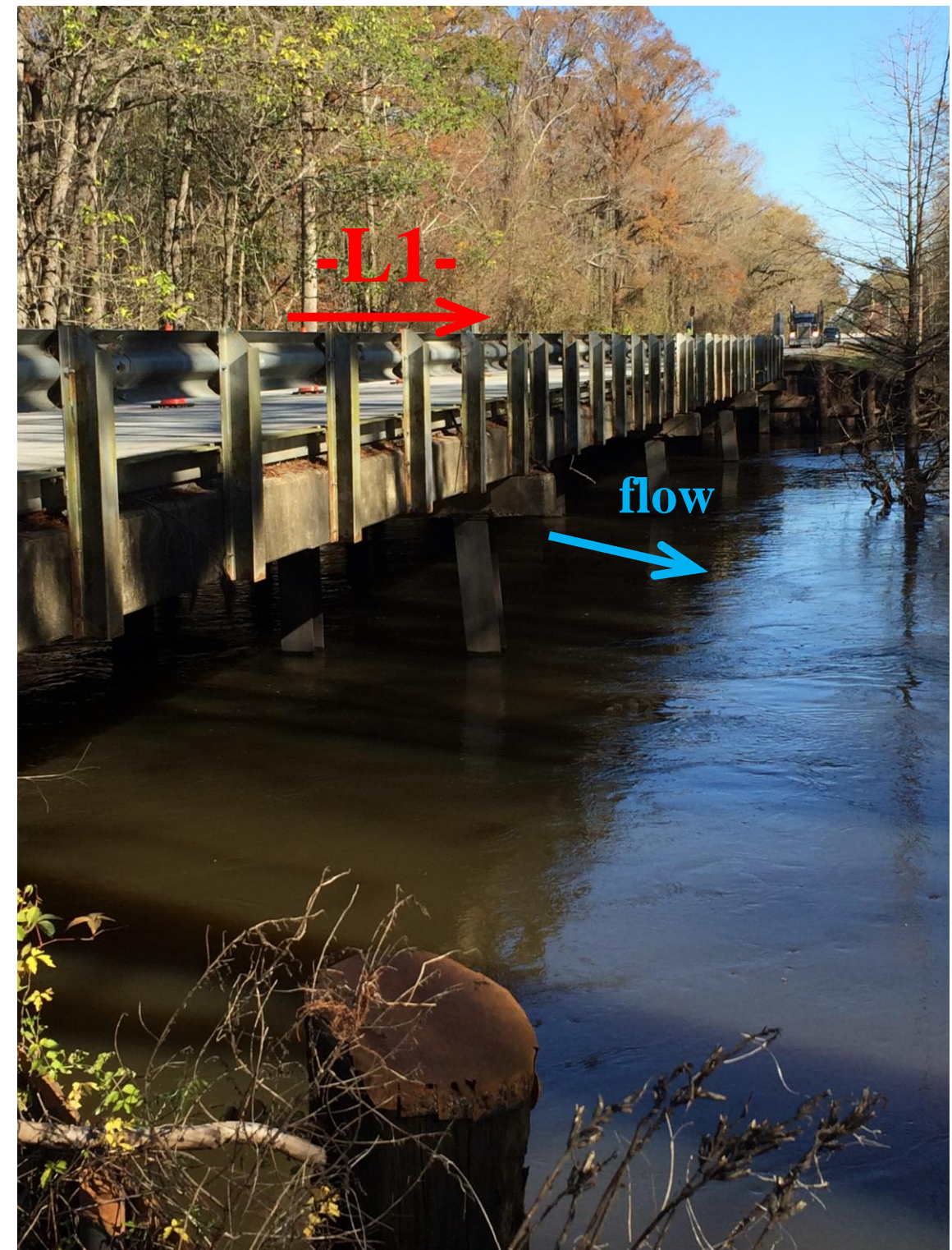
Looking North towards End Bent 2
