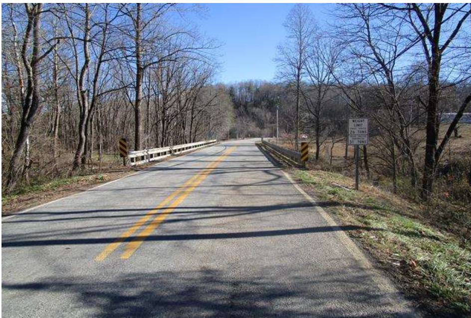
WEST APPROACH LOOKING EAST
