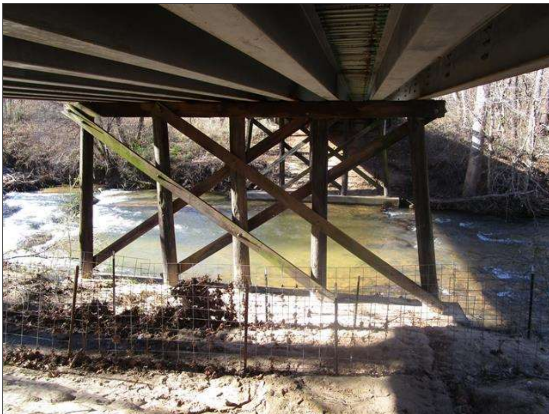
BENT 2 LOOKING WEST
