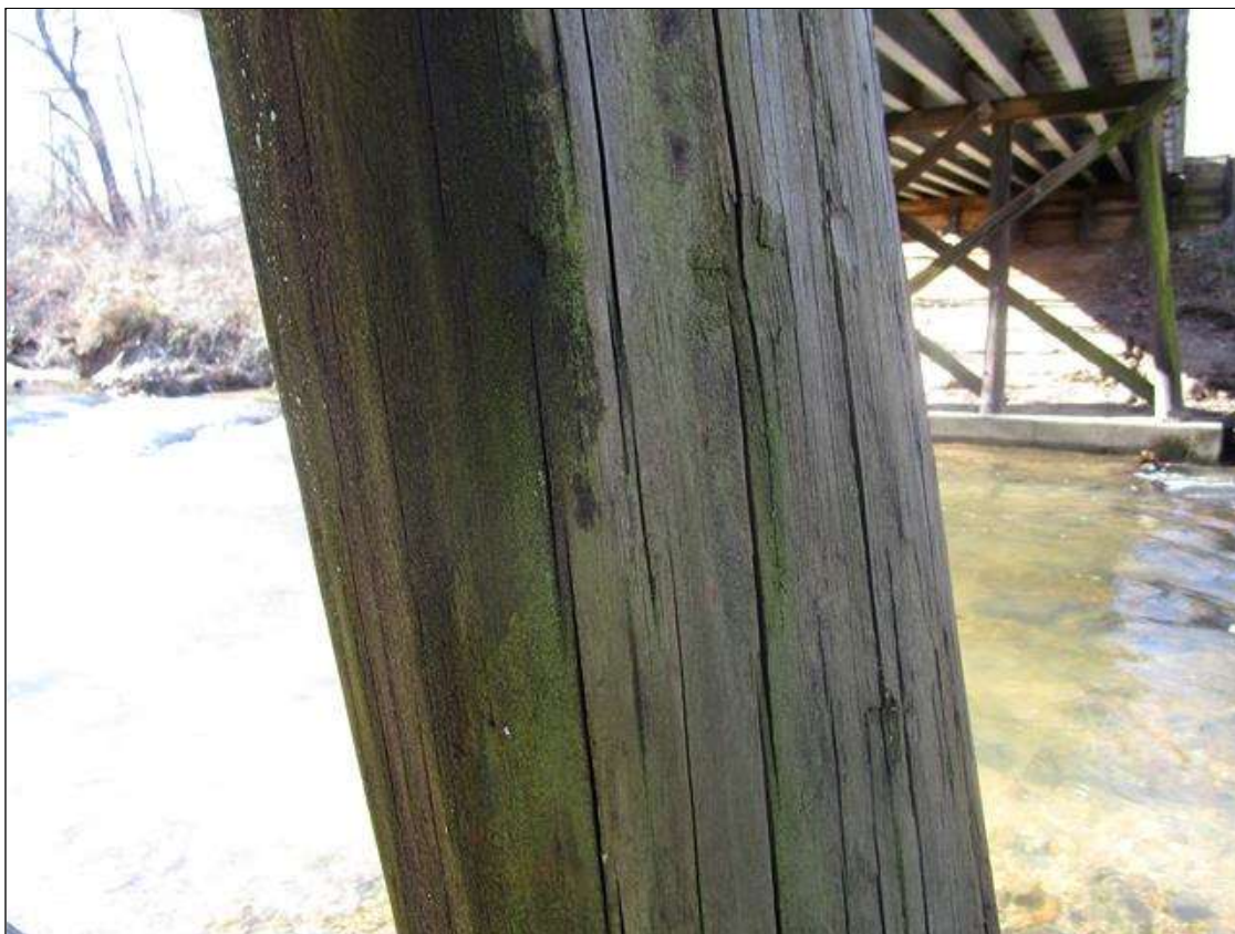
TYPICAL CHECKING IN PILES
