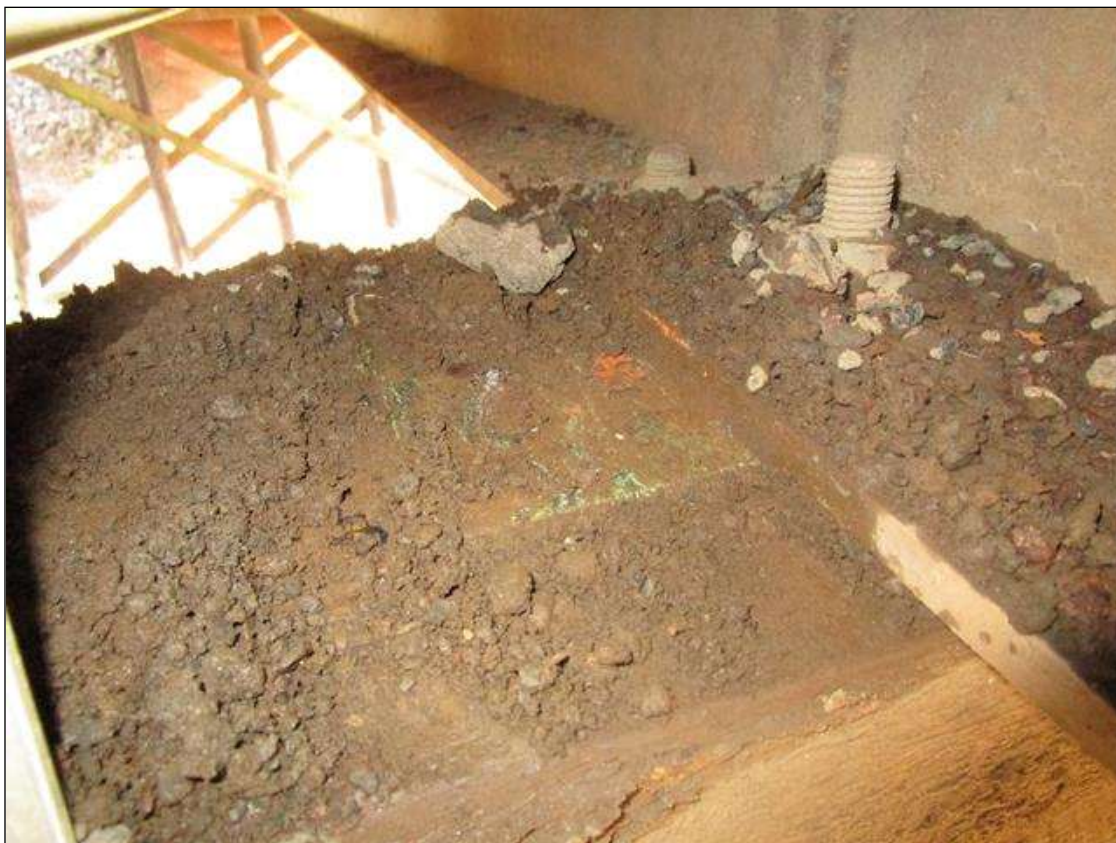
SURFACE CORROSION ON INTERIOR BENT BEARINGS FOR BEAMS WITH CORROSION AT ENDS
