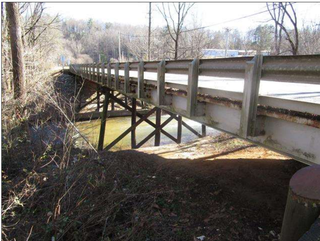
DOWNSTREAM STRUCTURE ELEVATION
