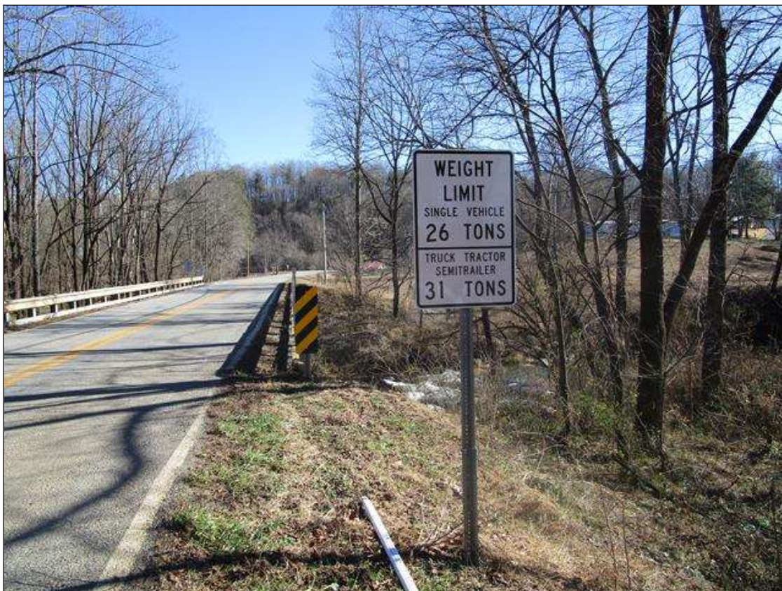
TYPICAL WEIGHT LIMIT SIGN
