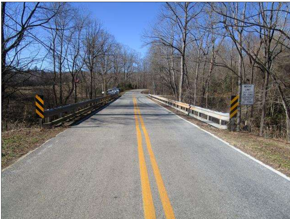
EAST APPROACH LOOKING WEST
