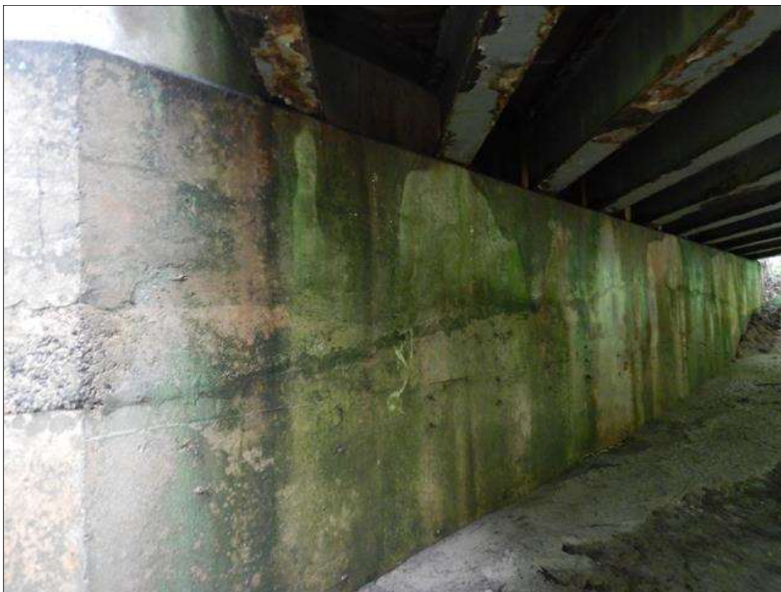
typical end bent [End Bent 2 in view]
