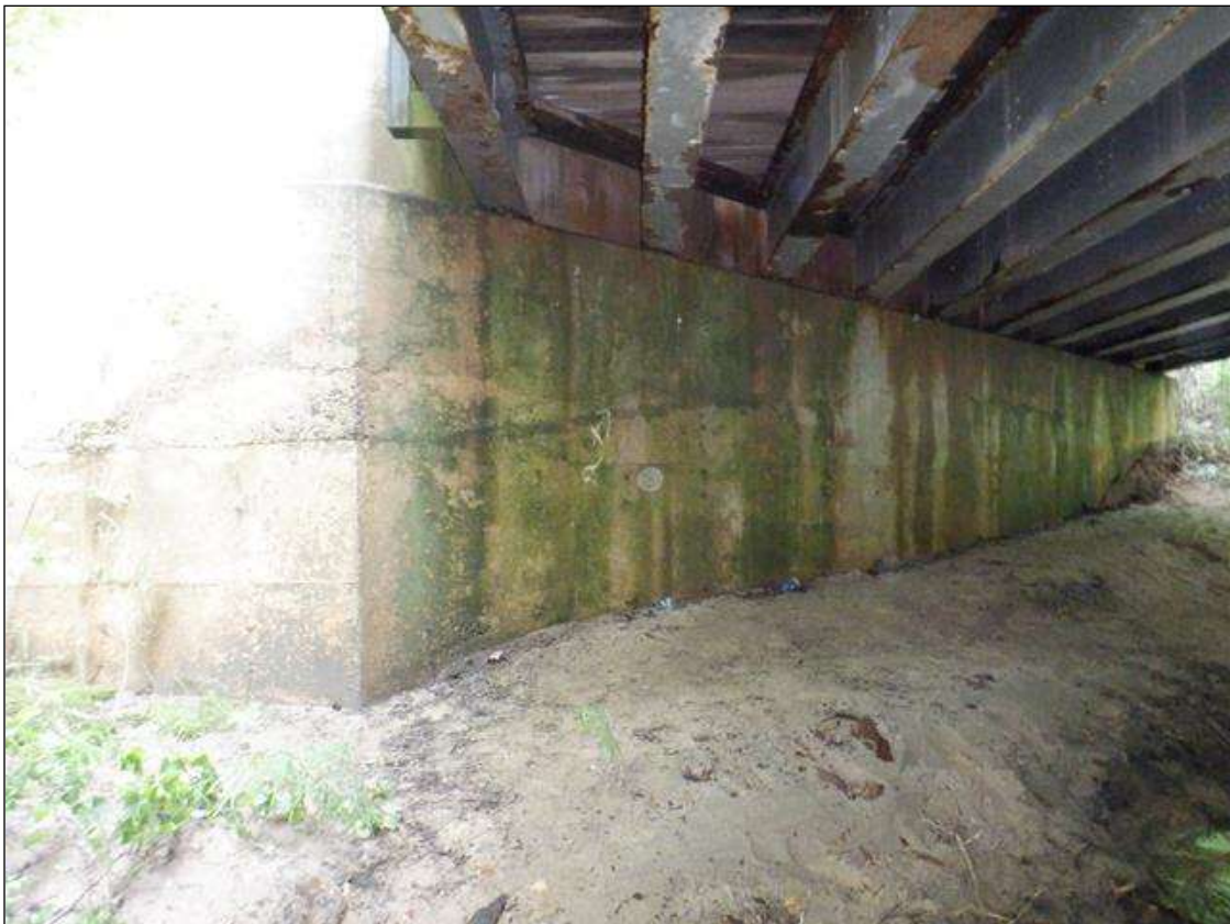
typical end bent [End Bent 2 in view]
