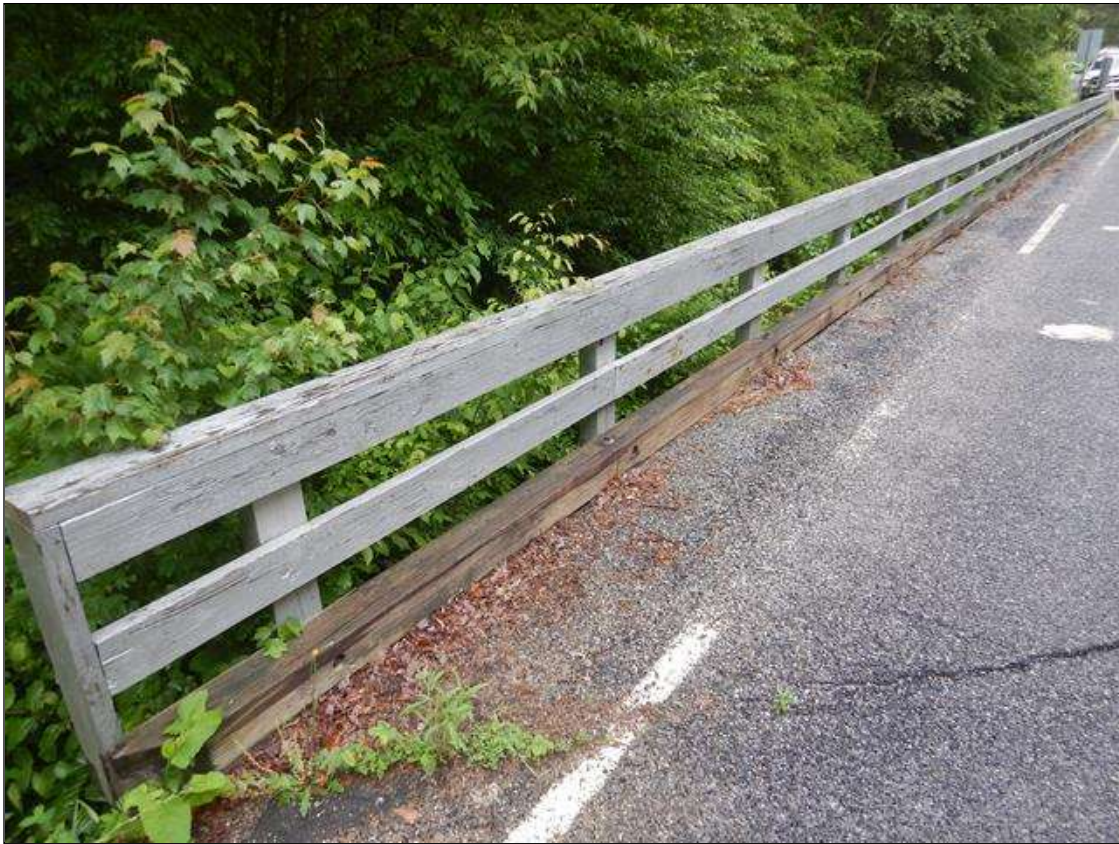
left bridge rail
