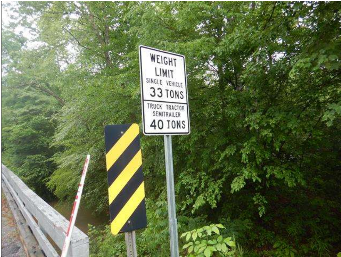
far approach load posting
