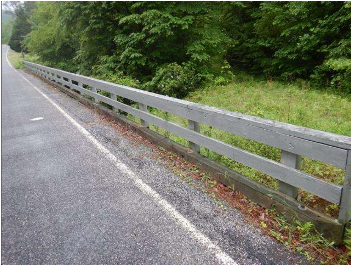
right bridge rail
