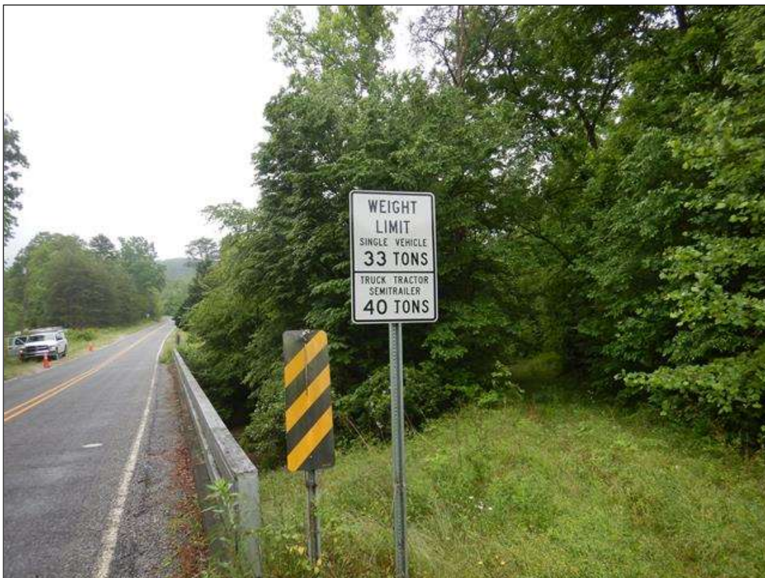
near approach load posting
