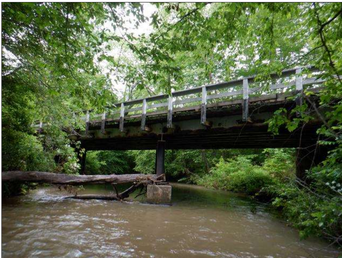
South profile looking North
