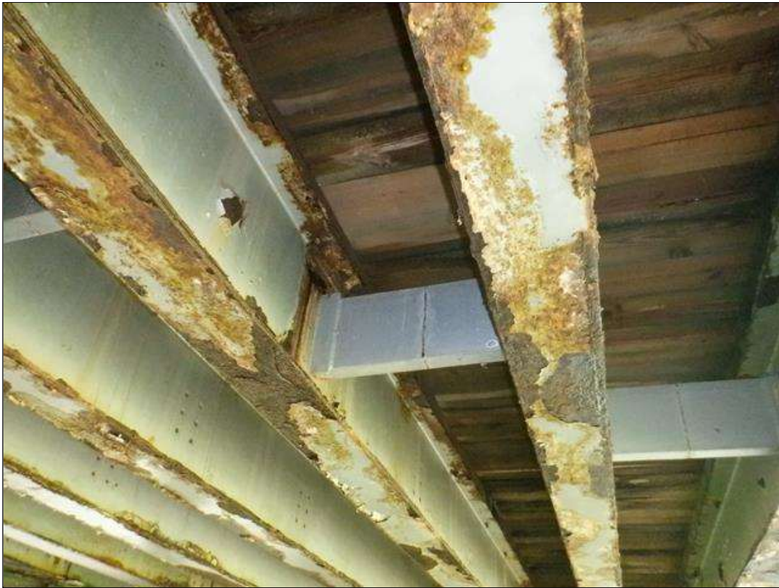
typical underside of deck
