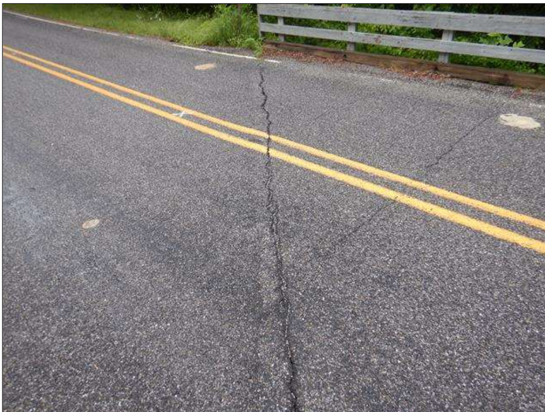
typical asphalt over end bent [asphalt over end bent 1 in view]
