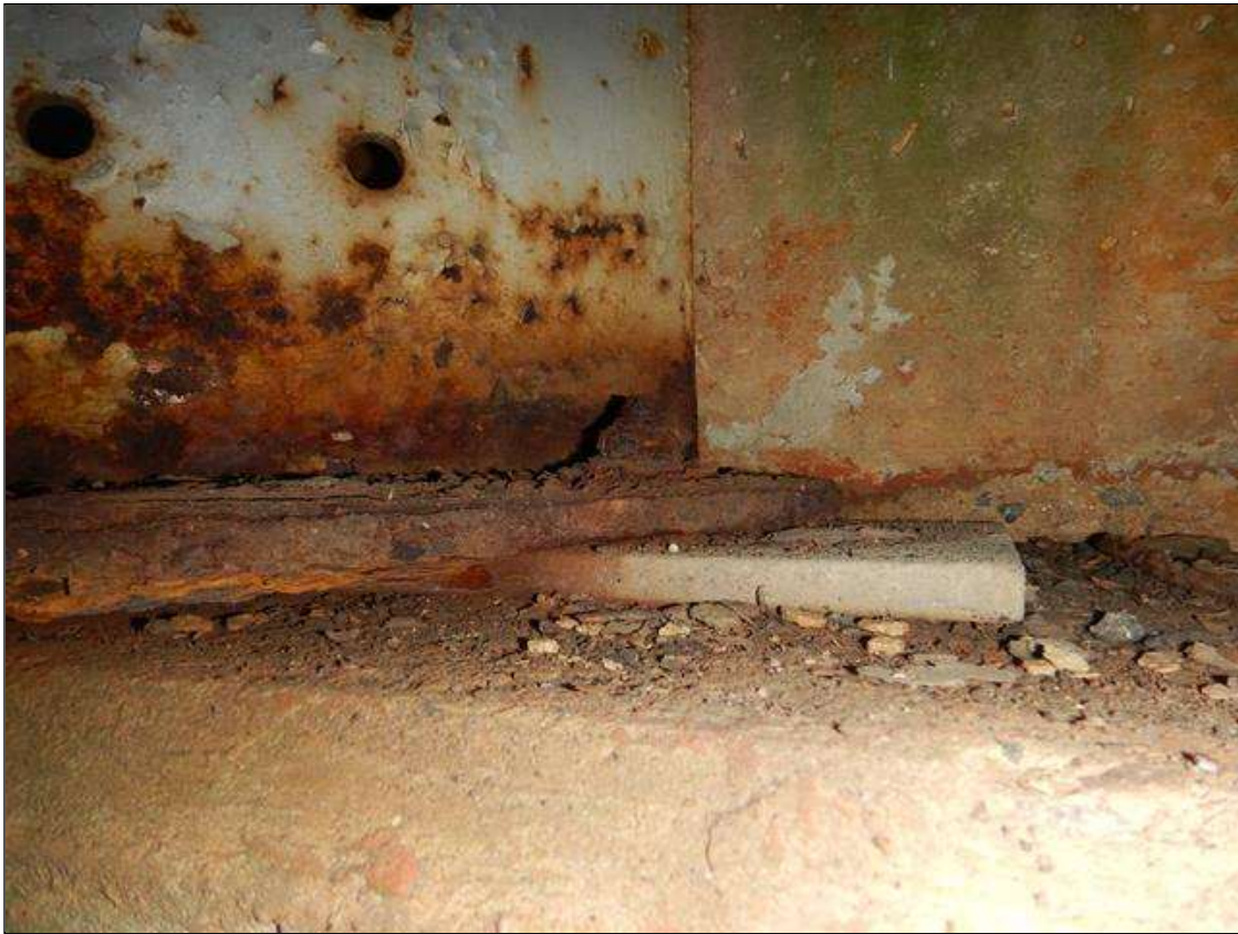
typical end bearing
