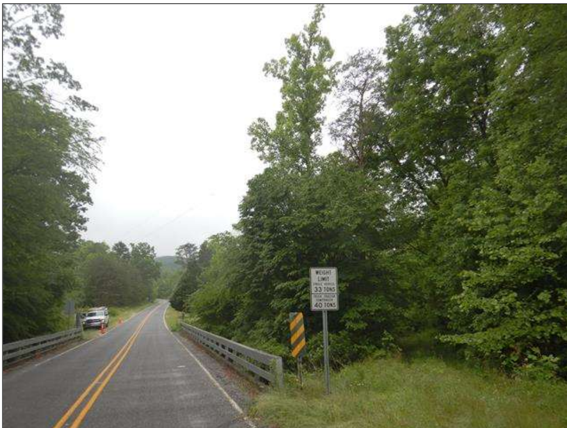
overhead utility across structure
