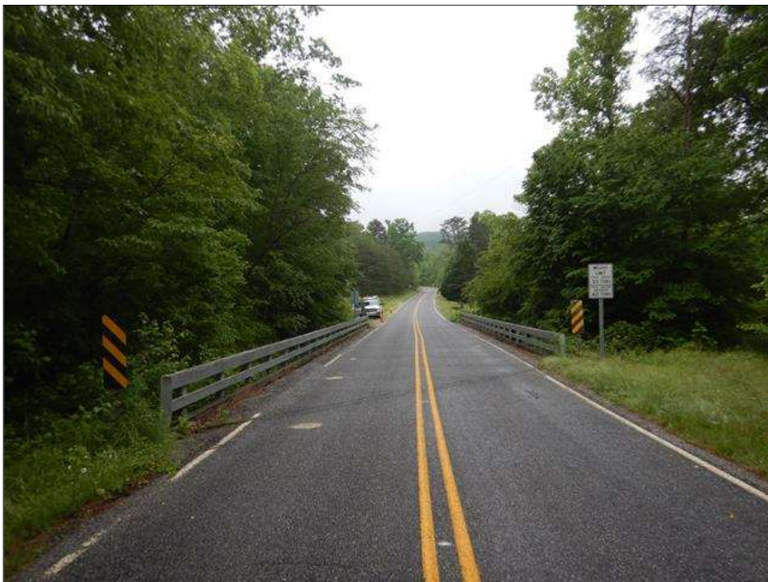
West approach looking East
