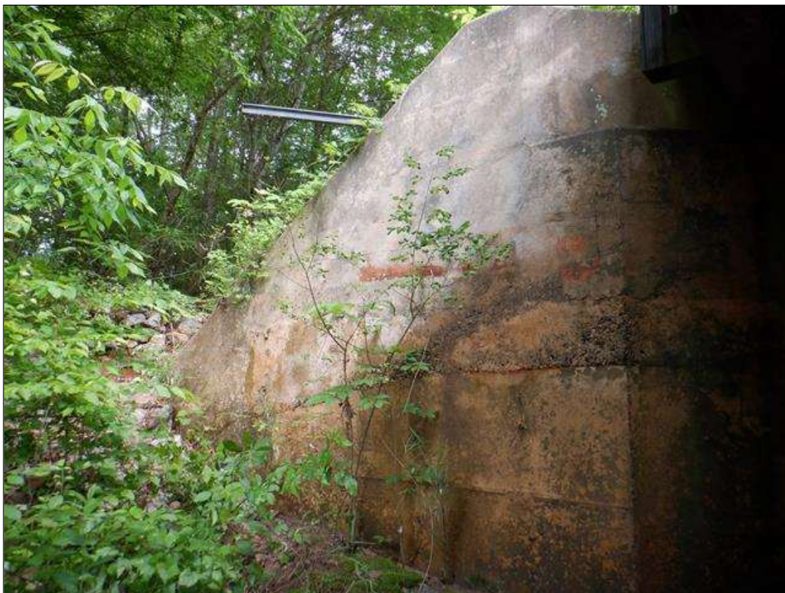
typical wingwall [Northwest in view]
