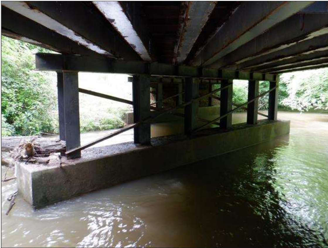
typical interior bent [bent 2 in view]
