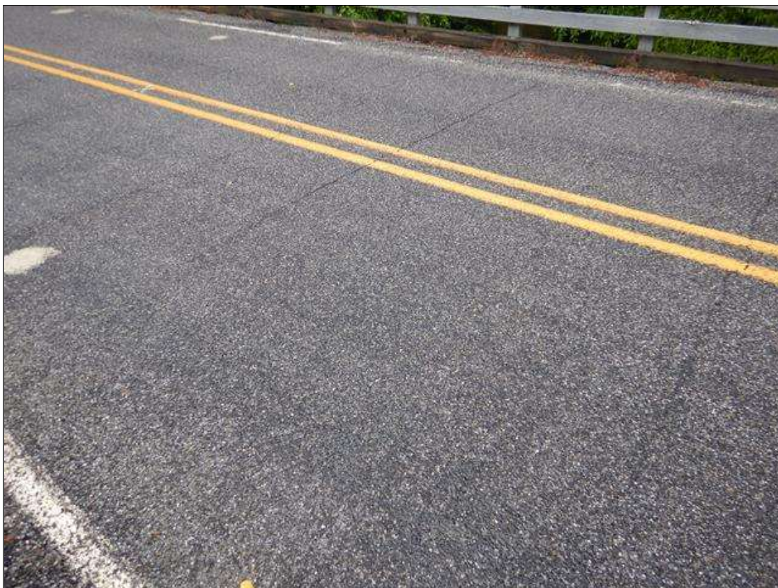
typical asphalt over interior bent [asphalt over bent 1 in view]
