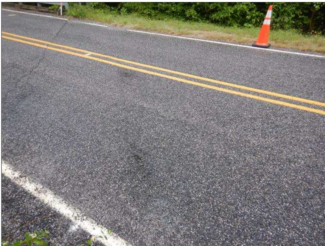
East approach asphalt
