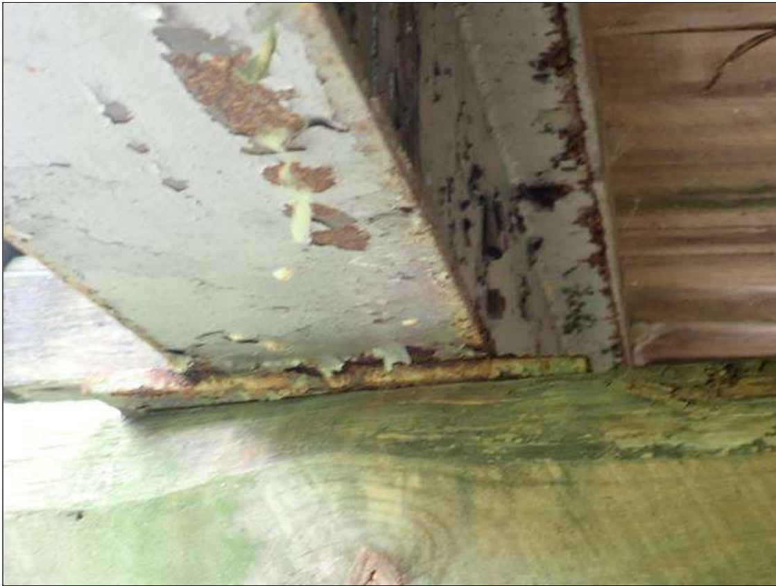
typical interior bearing
