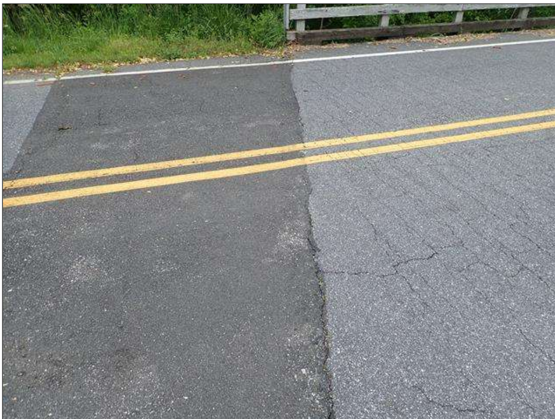
asphalt over end bent 1
