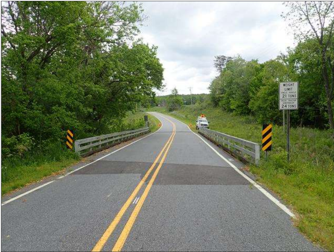
South approach looking North
