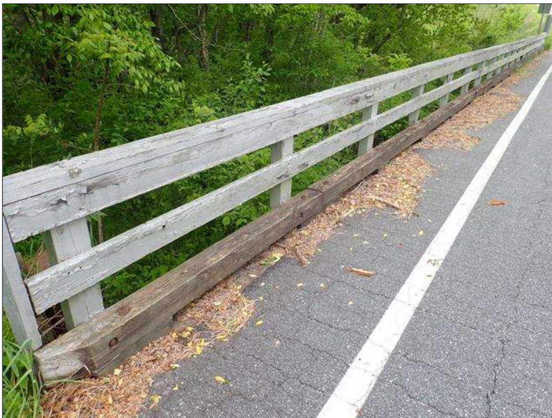
left bridge rail
