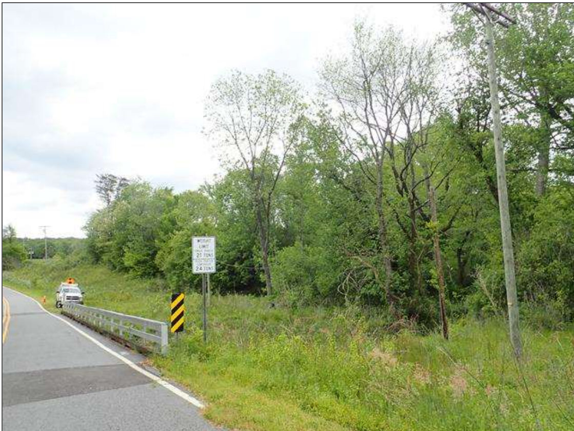
overhead utility along right side
