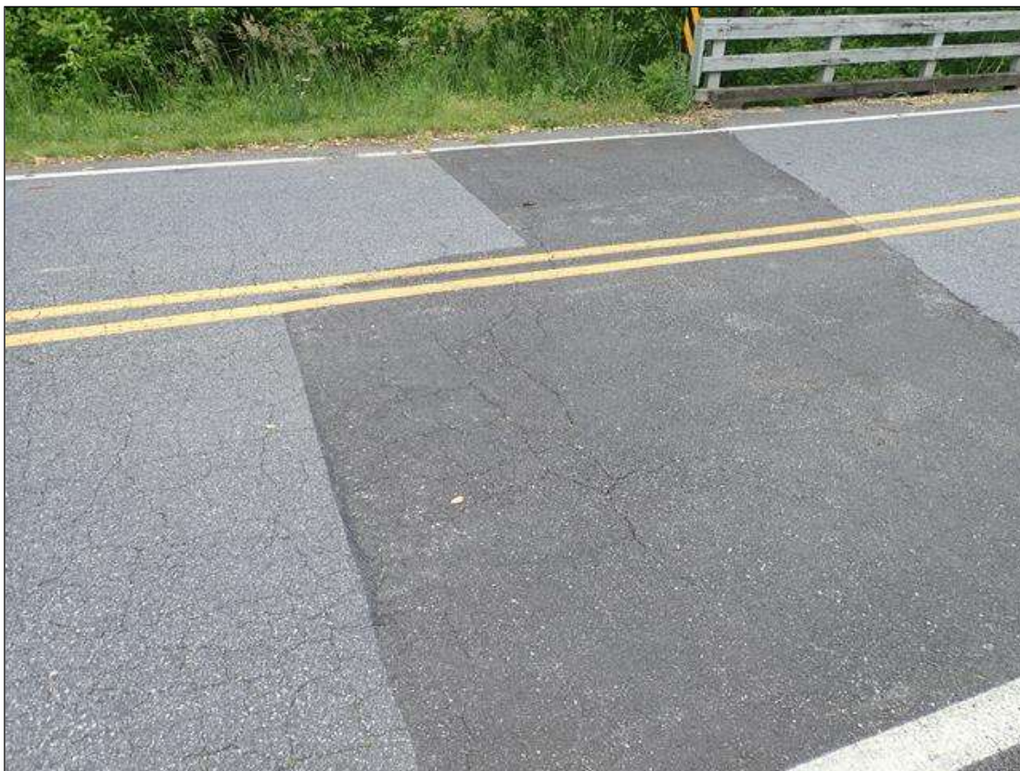
South approach asphalt
