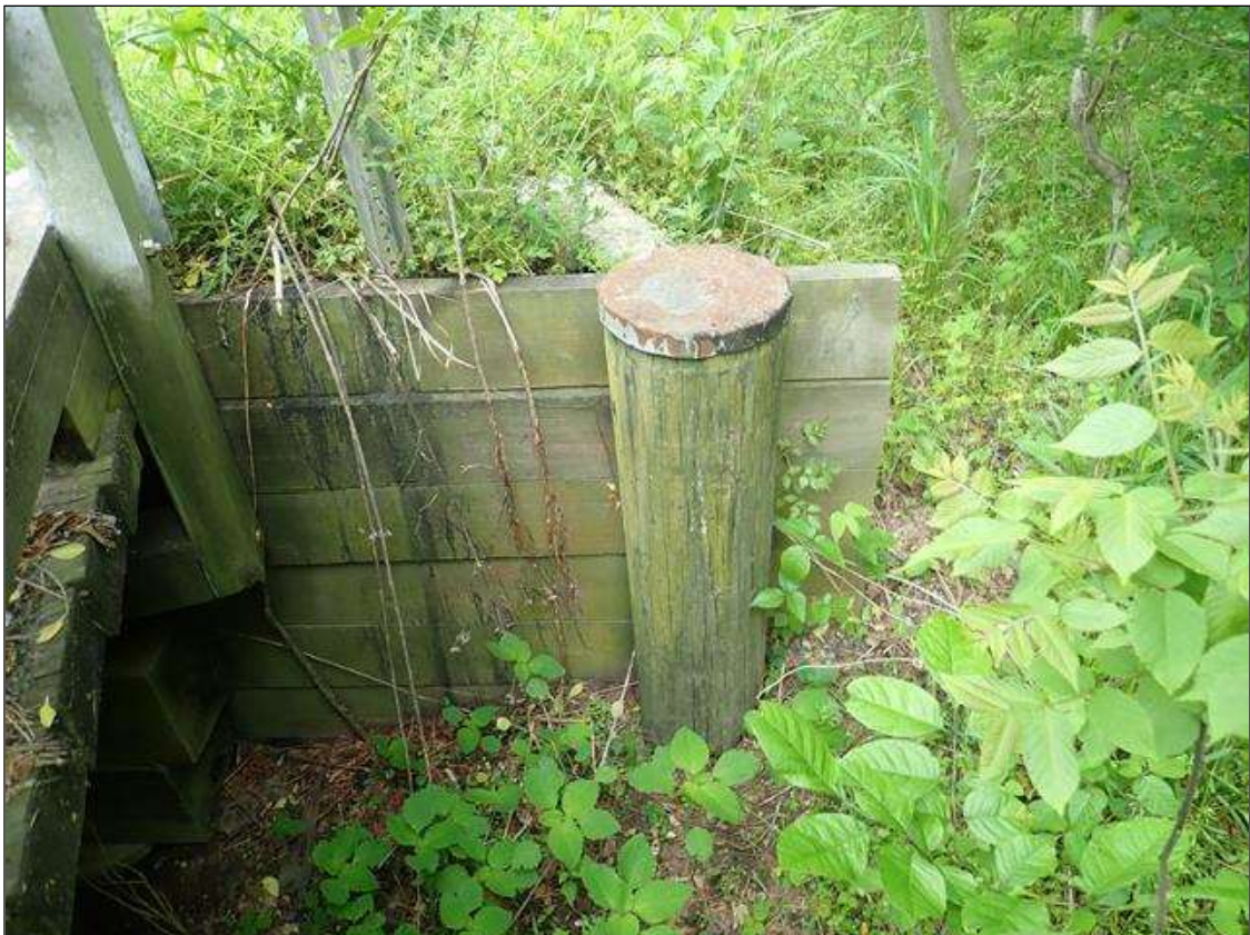
Southwest wingwall [all similar]
