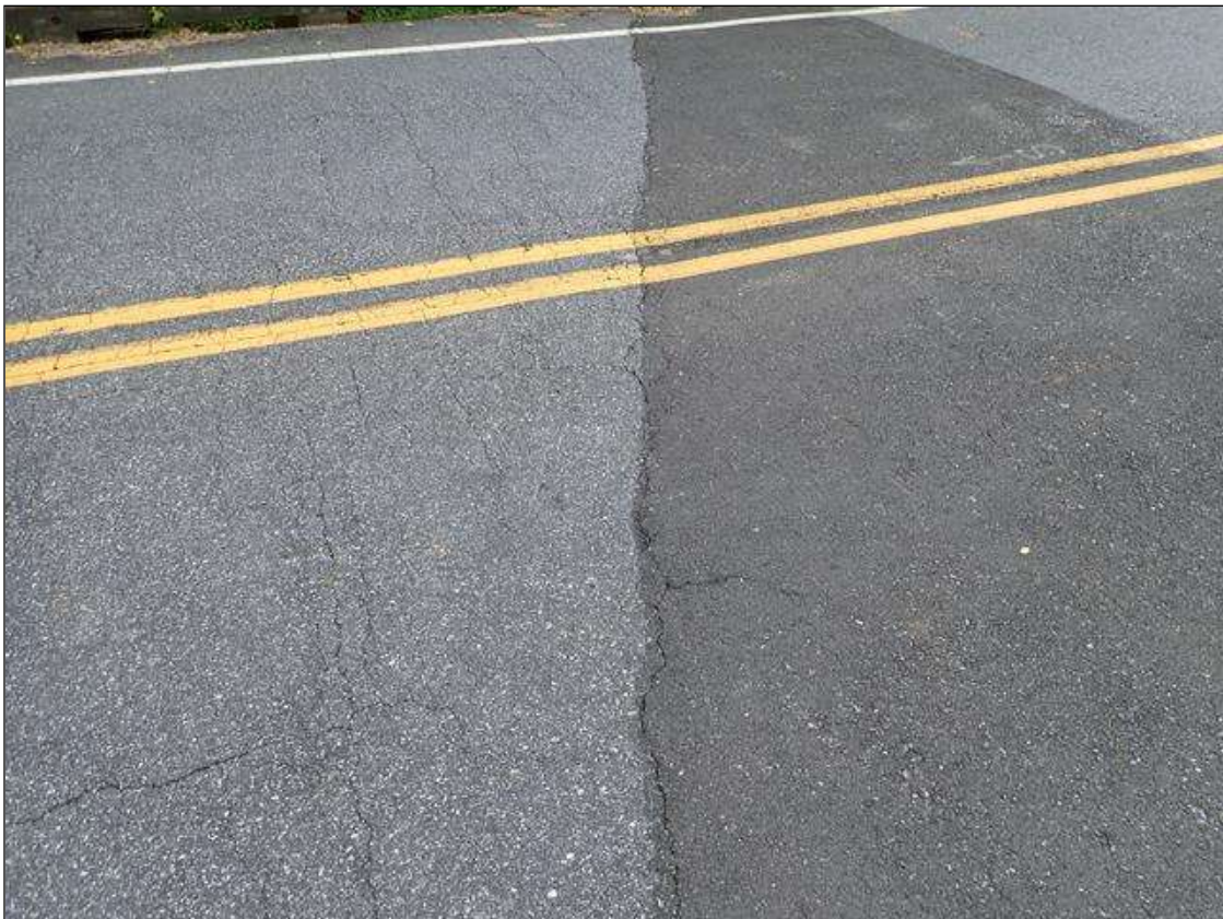
asphalt over end bent 2
