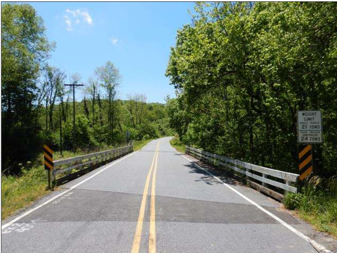
North approach looking South
