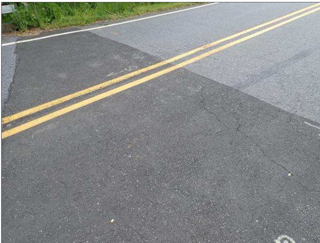
North approach asphalt
