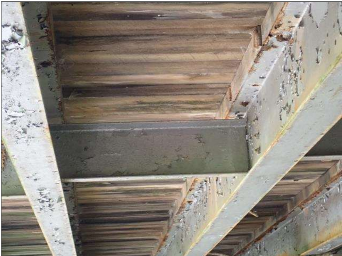
typical interior diaphragm
