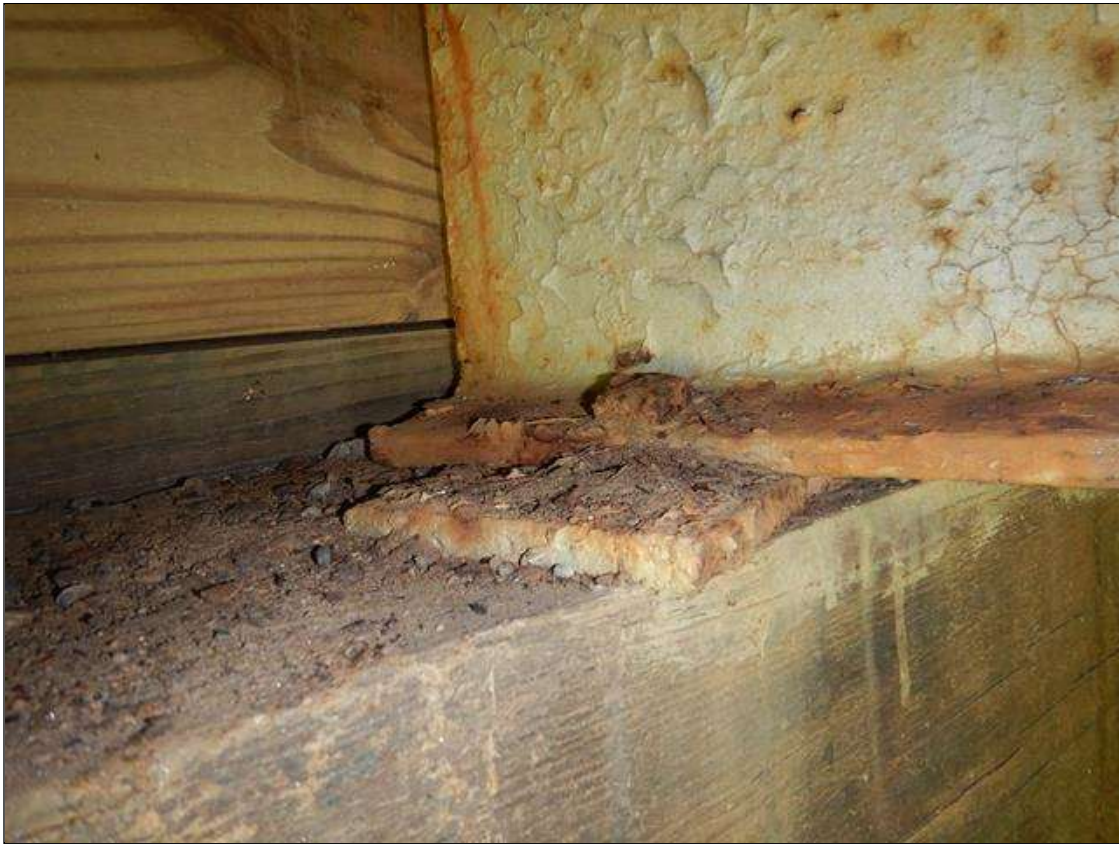
typical end bearing
