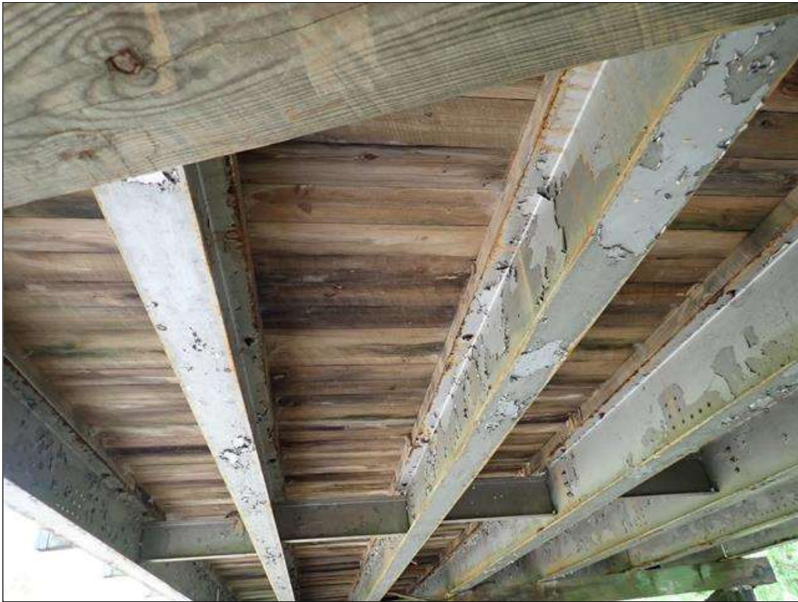
typical underside of deck
