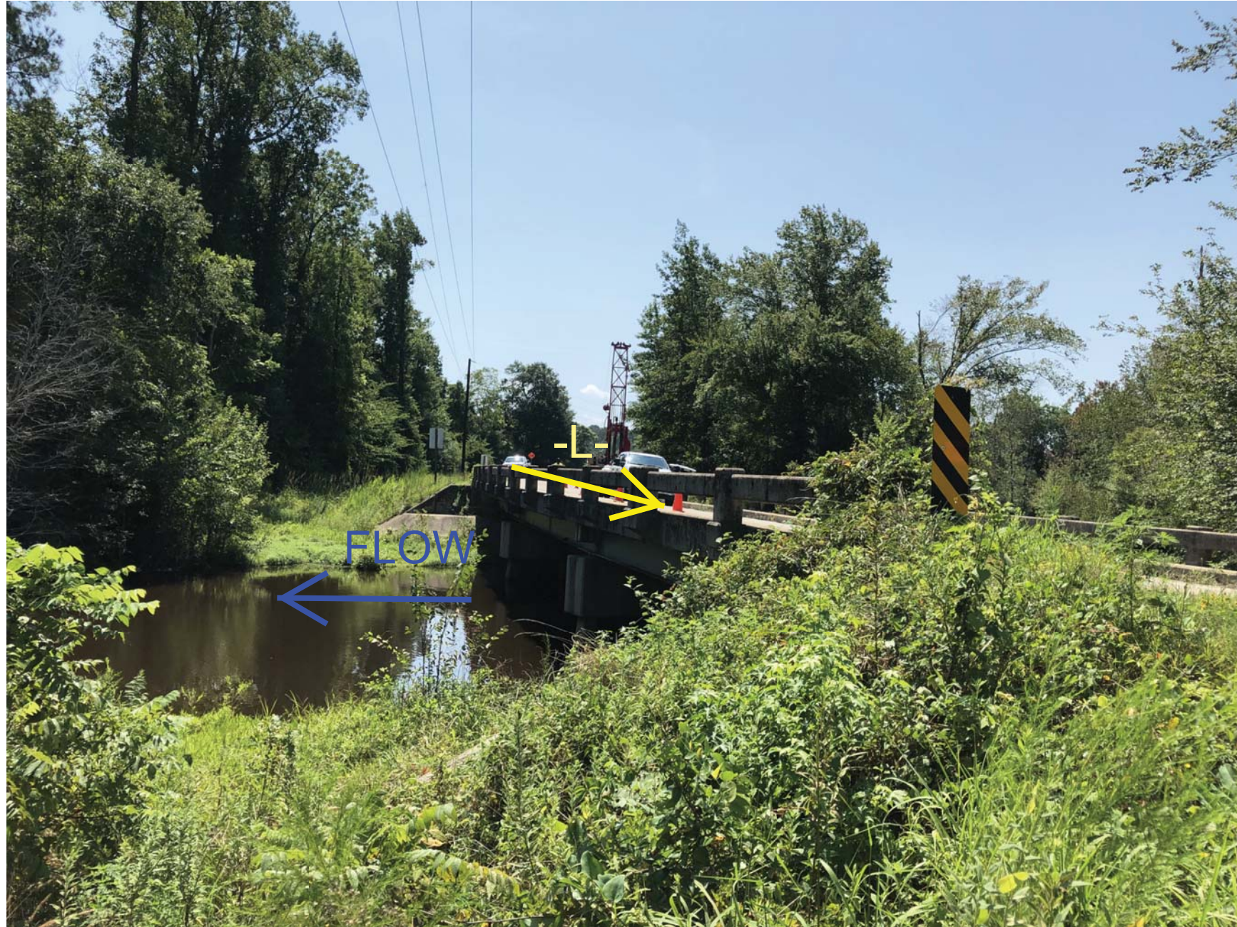
VIEW LOOKING SOUTH TOWARD END BENT 2
