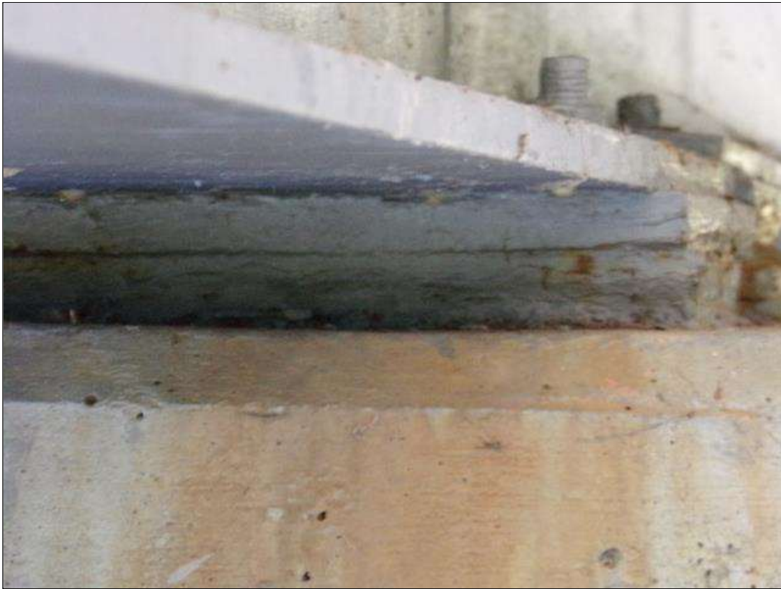
Typical bearing (Beam 2 Pier 1 Span 2)
