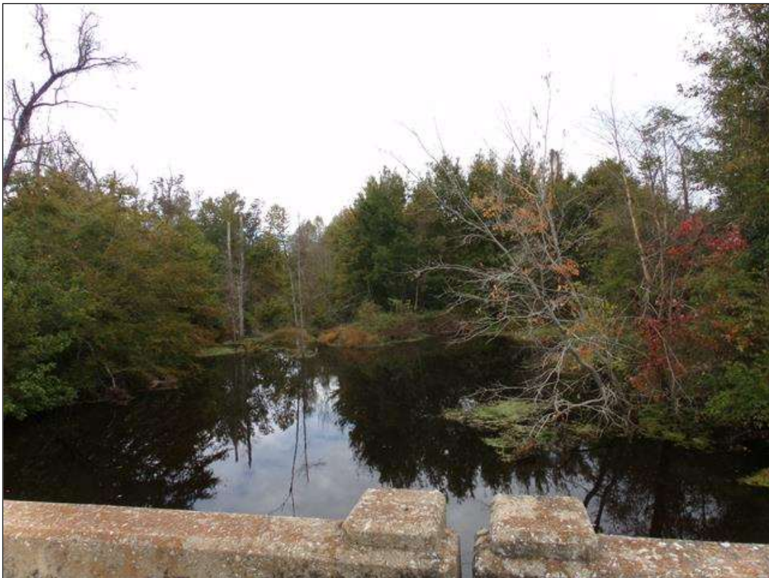
Looking north downstream
