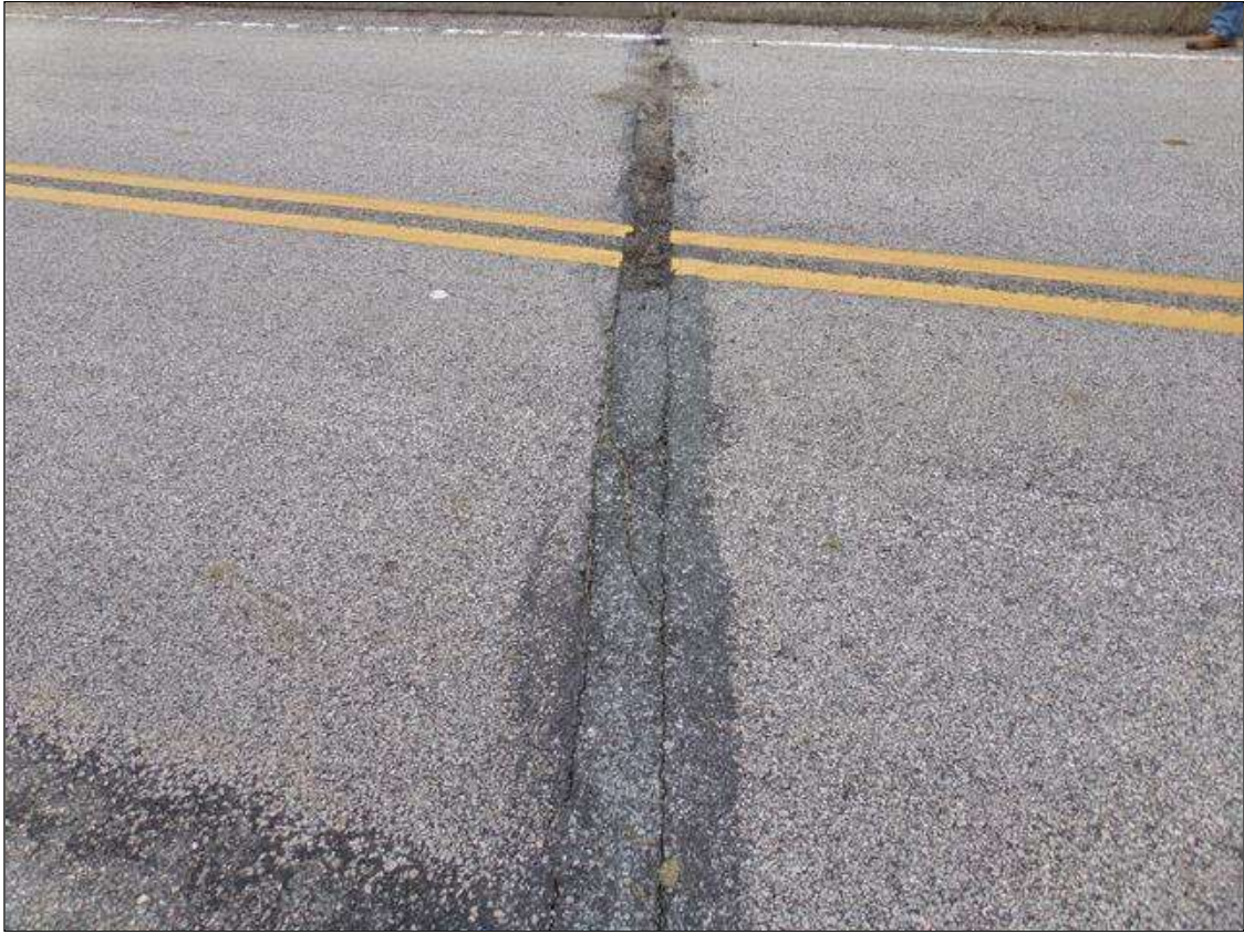
Joint over pier 1, pier 2 similar
