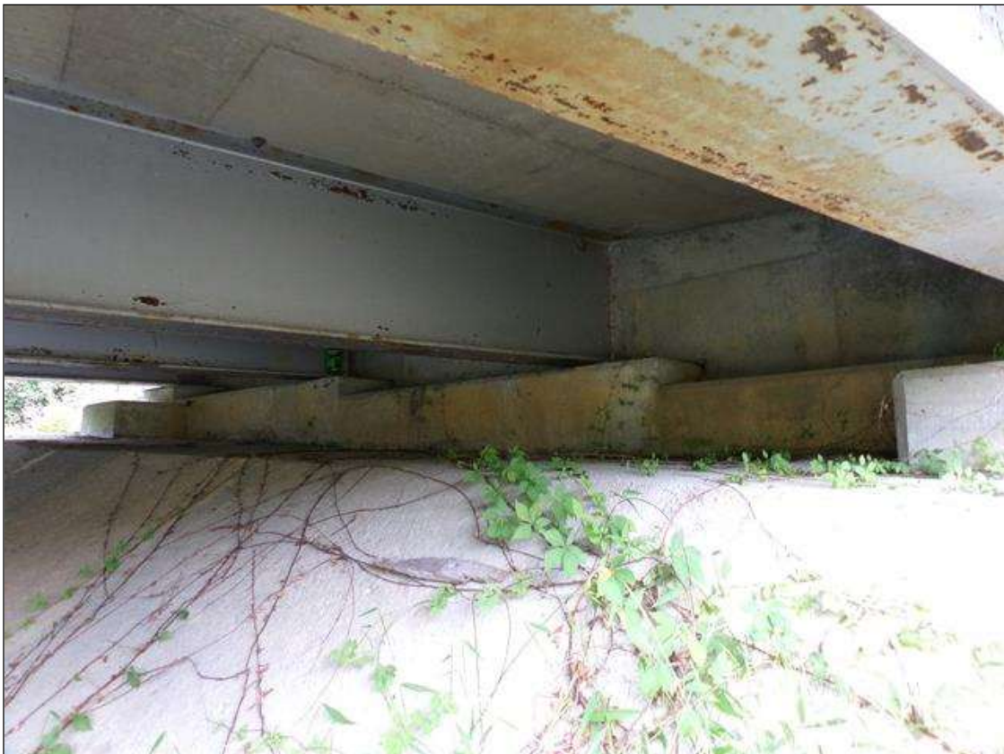
Abutment 2, abutment 1 similar
