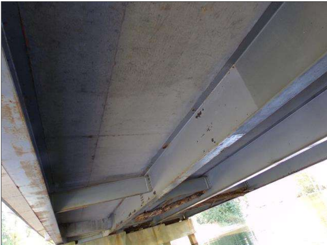
General Superstructure Underside (Span 2 shown.)
