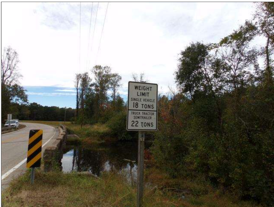
Posting sign at east approach
