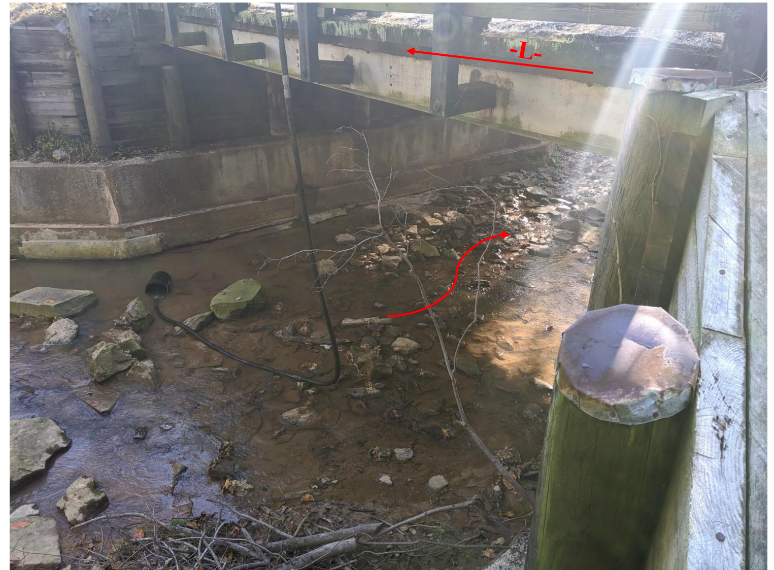
Photograph No. 2: Looking Upstream
