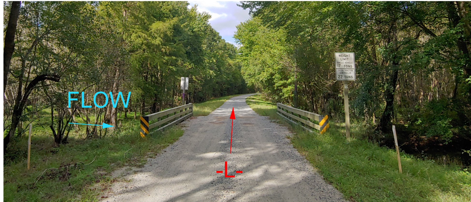
FROM END BENT 1 LOOKING UPSTATION
