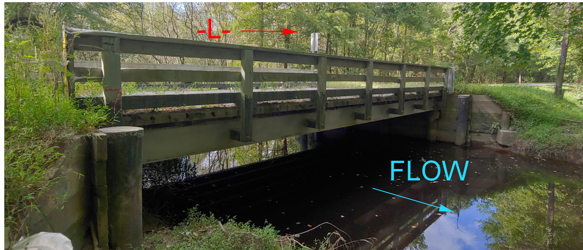
END BENT 1 RIGHT LOOKING UPSTREAM
