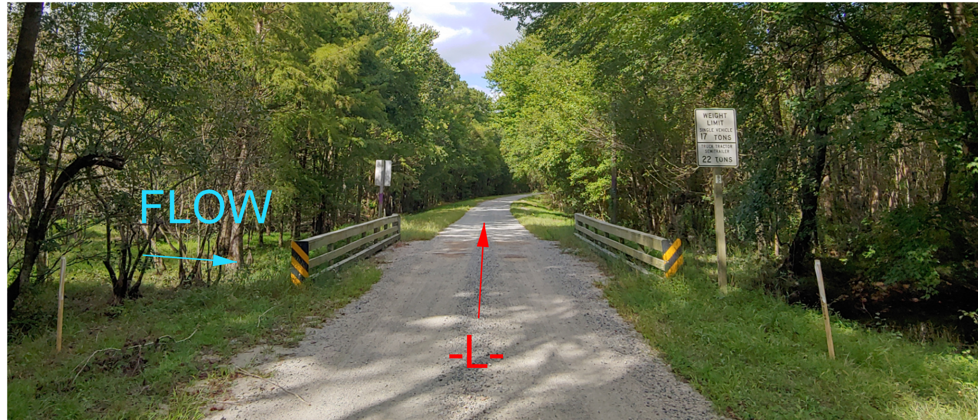
FROM END BENT 1 LOOKING UPSTATION
