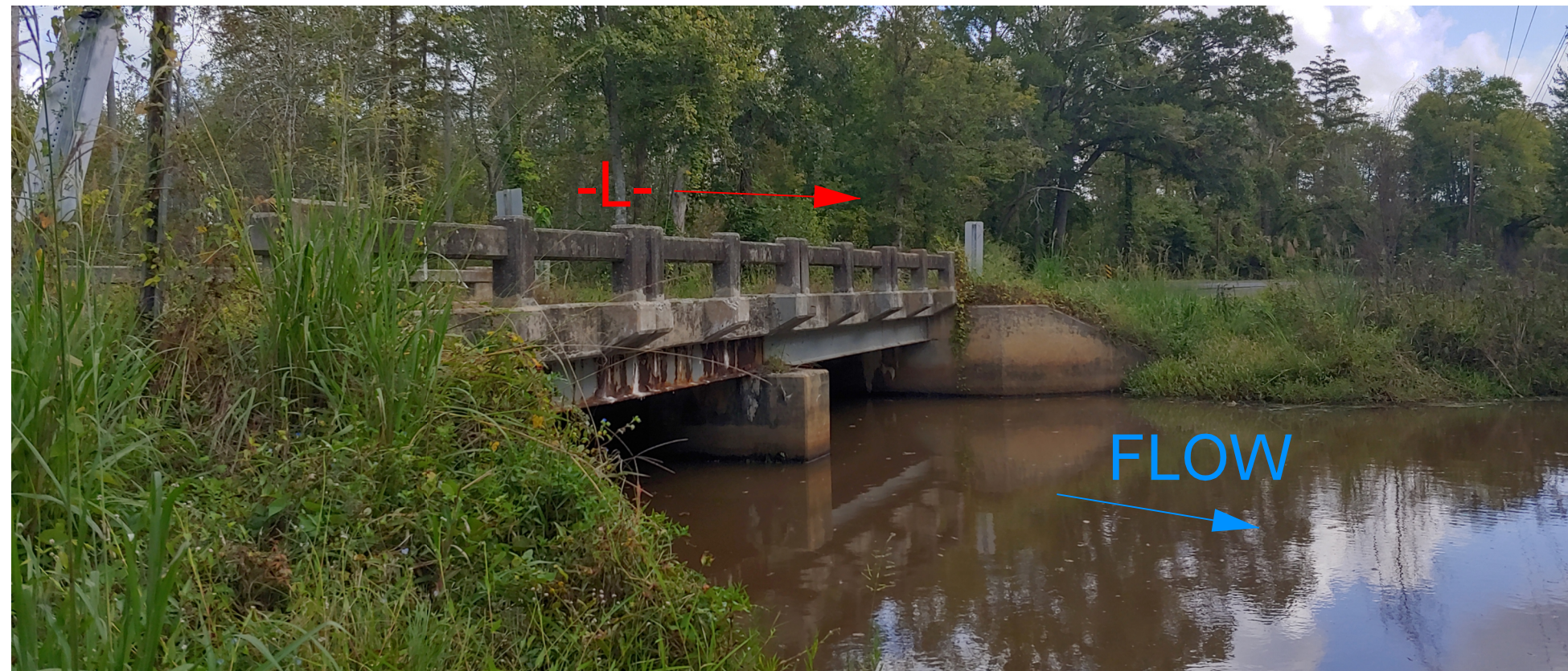
FROM END BENT 1 RIGHT LOOKING UPSTREAM
