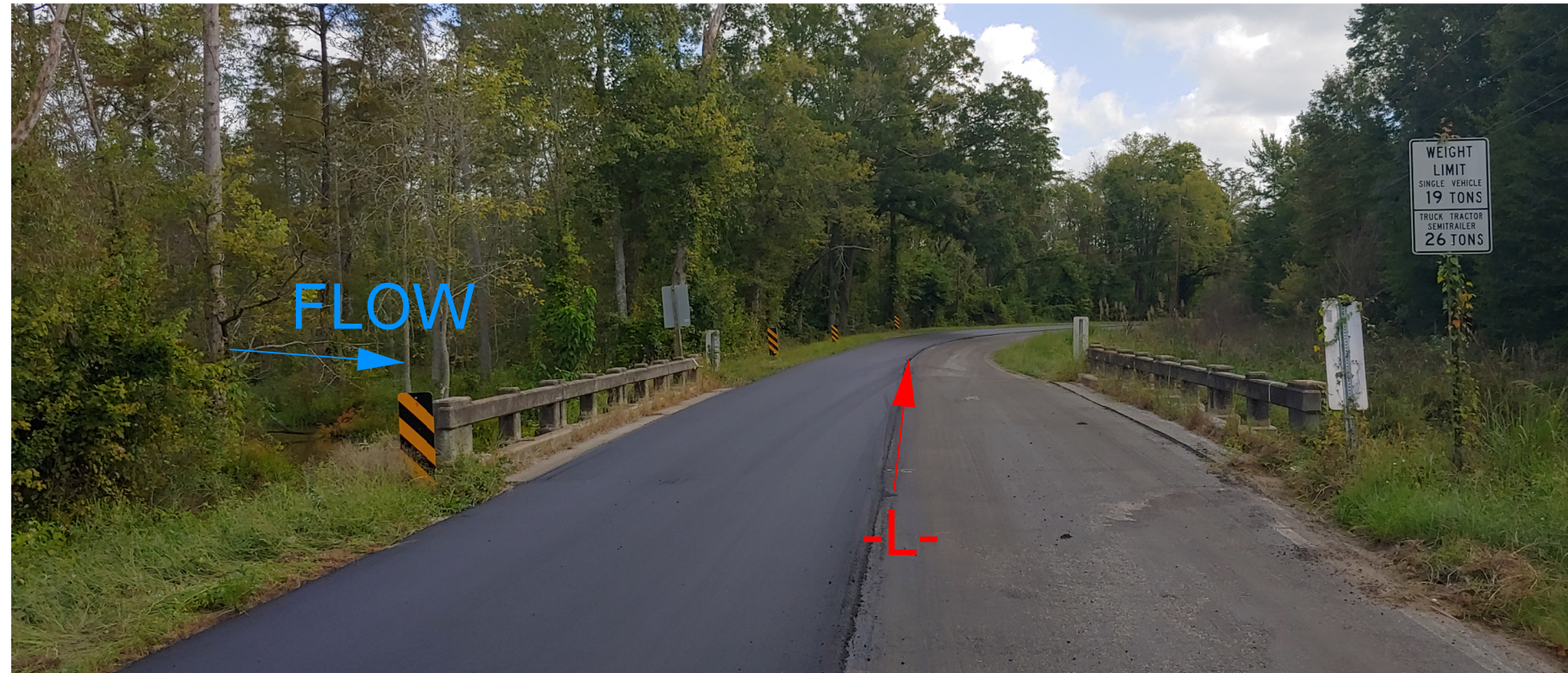
FROM END BENT 1 LOOKING UPSTATION
