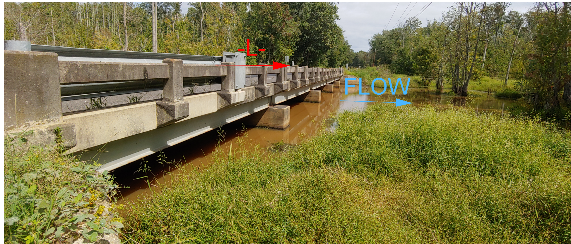
FROM END BENT 1 RIGHT LOOKING EAST
