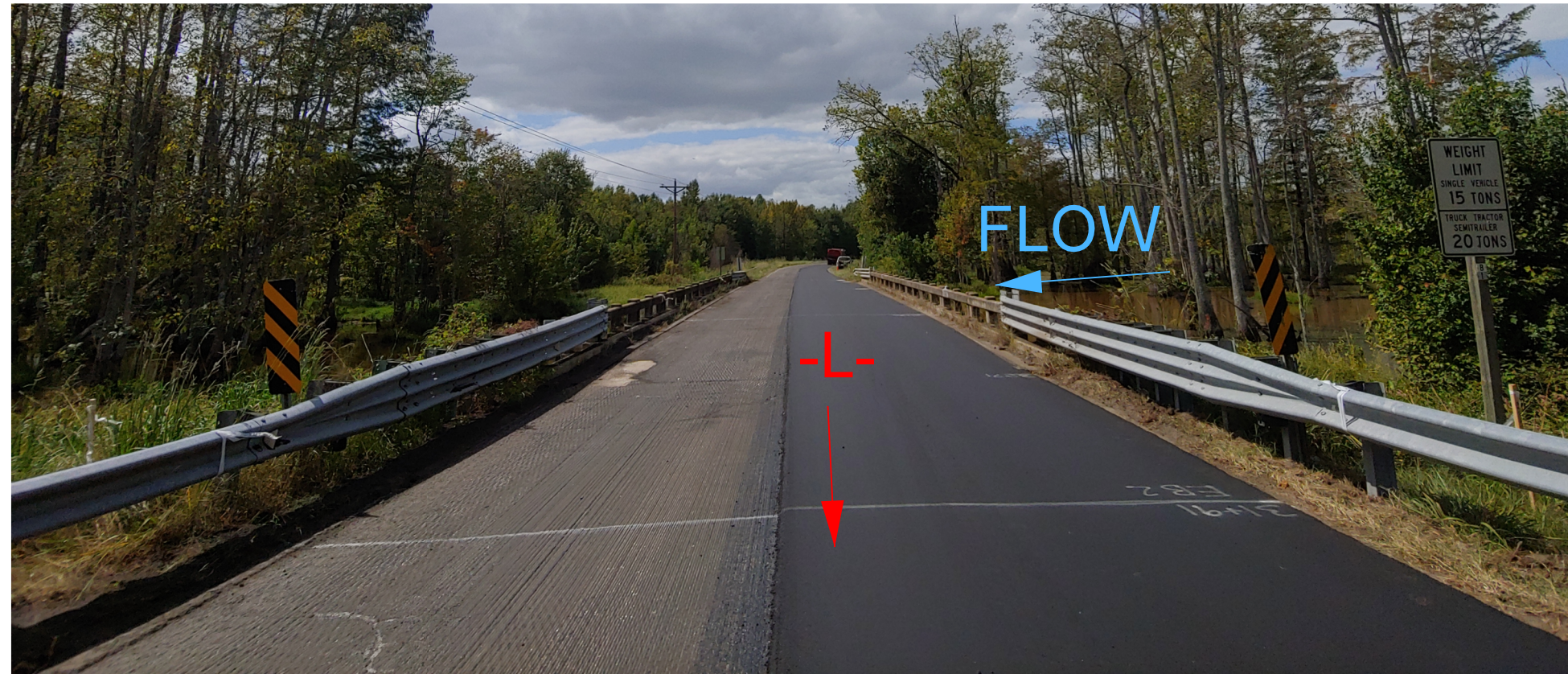
FROM END BENT 2 LOOKING WEST
