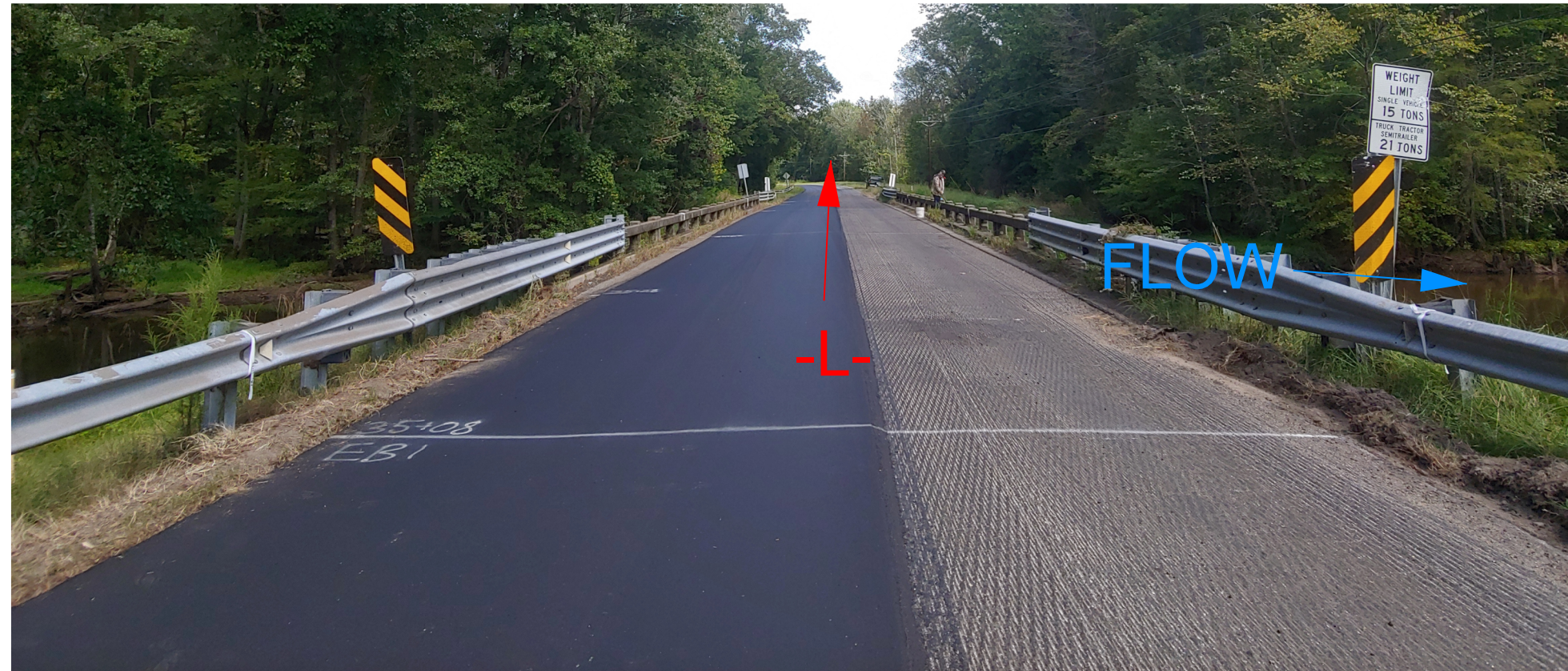
FROM END BENT 1 LOOKING EAST
