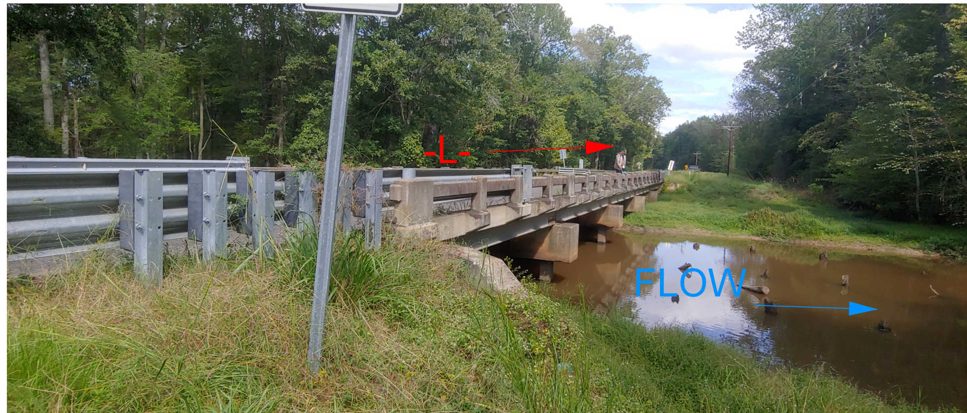
FROM END BENT 1 RIGHT LOOKING EAST
