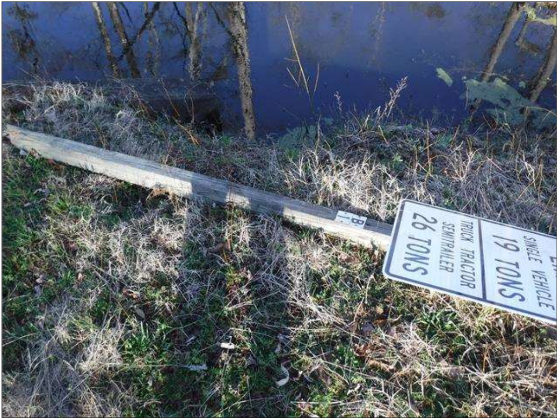
POSTING SIGN DOWN NORTH END MISSING AT SOUTH END PRIORITY MAINTENANCE ISSUED
