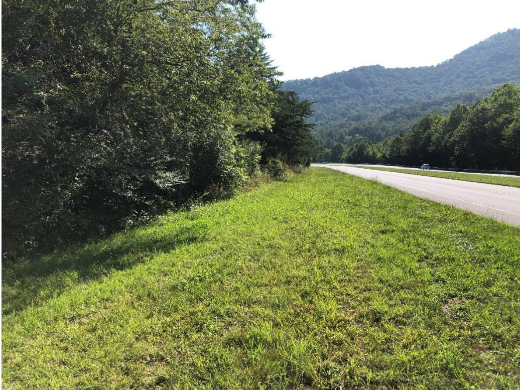
Waste Site Facing South
