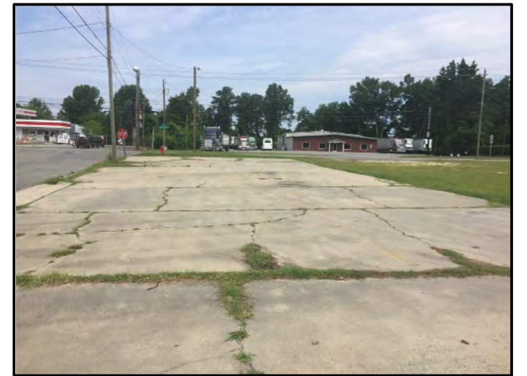
View of Survey Area (Facing Approximately West)
