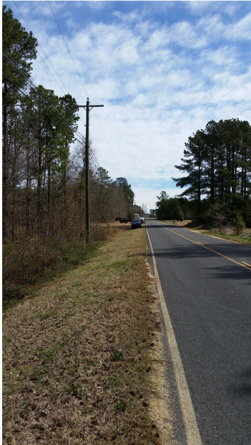
1. View looking East along -Y3- from EB1 to EB2.
