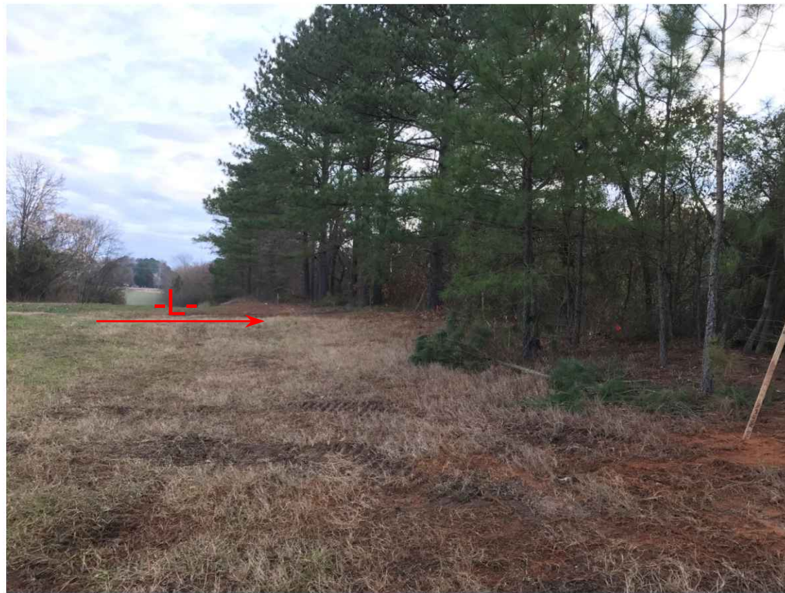
LOOKING RIGHT TO LEFT ALONG END BENT 1
