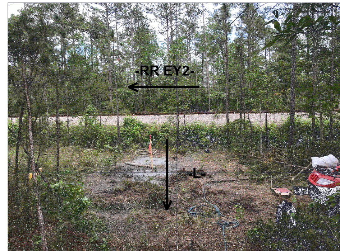
VIEW AT EB2-B RL ALONG -L- FACING DOWN-STATIONING TOWARDS B2-B RL AND -RR EY2- (CAMP LEJEUNE RAILROAD)
