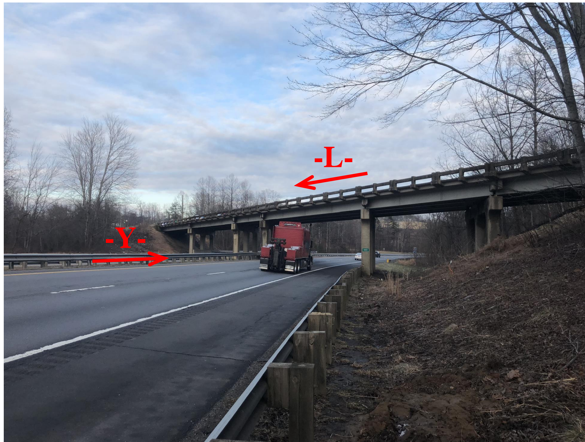
Looking Northeast towards End Bent 2
