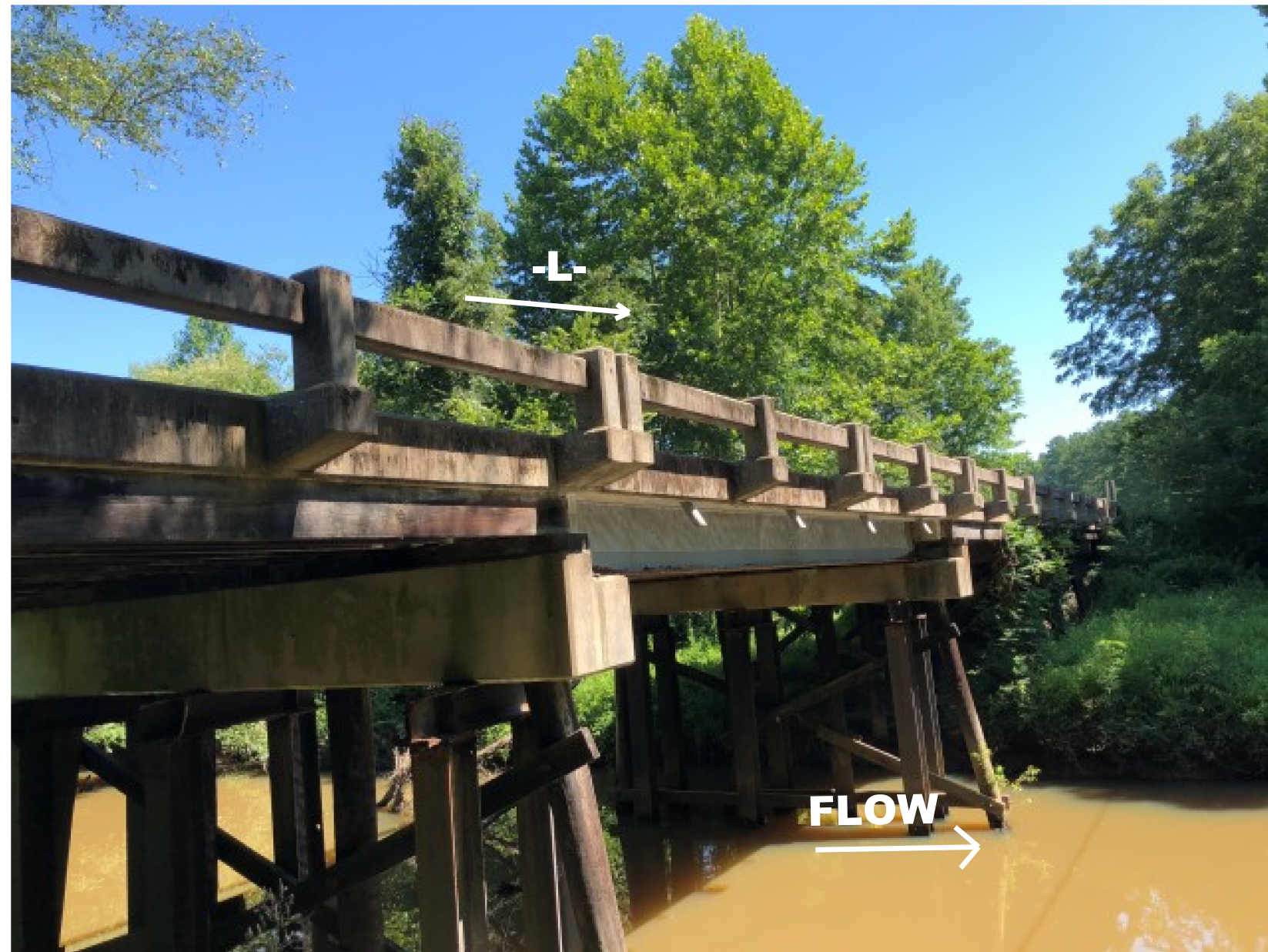
PHOTOGRAPH NO.1.: VIEW LOOKING NORTH.
